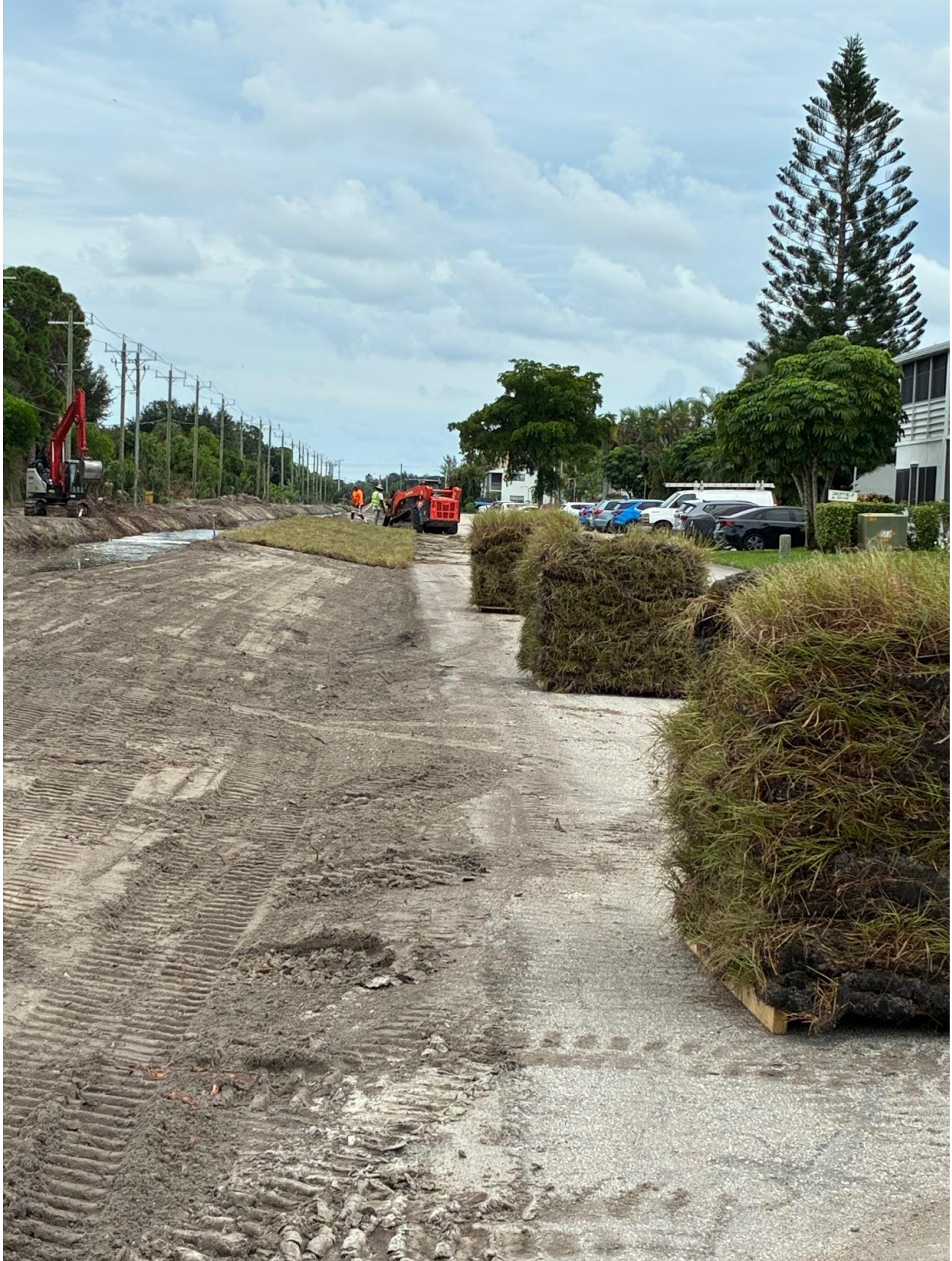
NORTH CANAL- SOD INSTALLATION CONTINUES.
