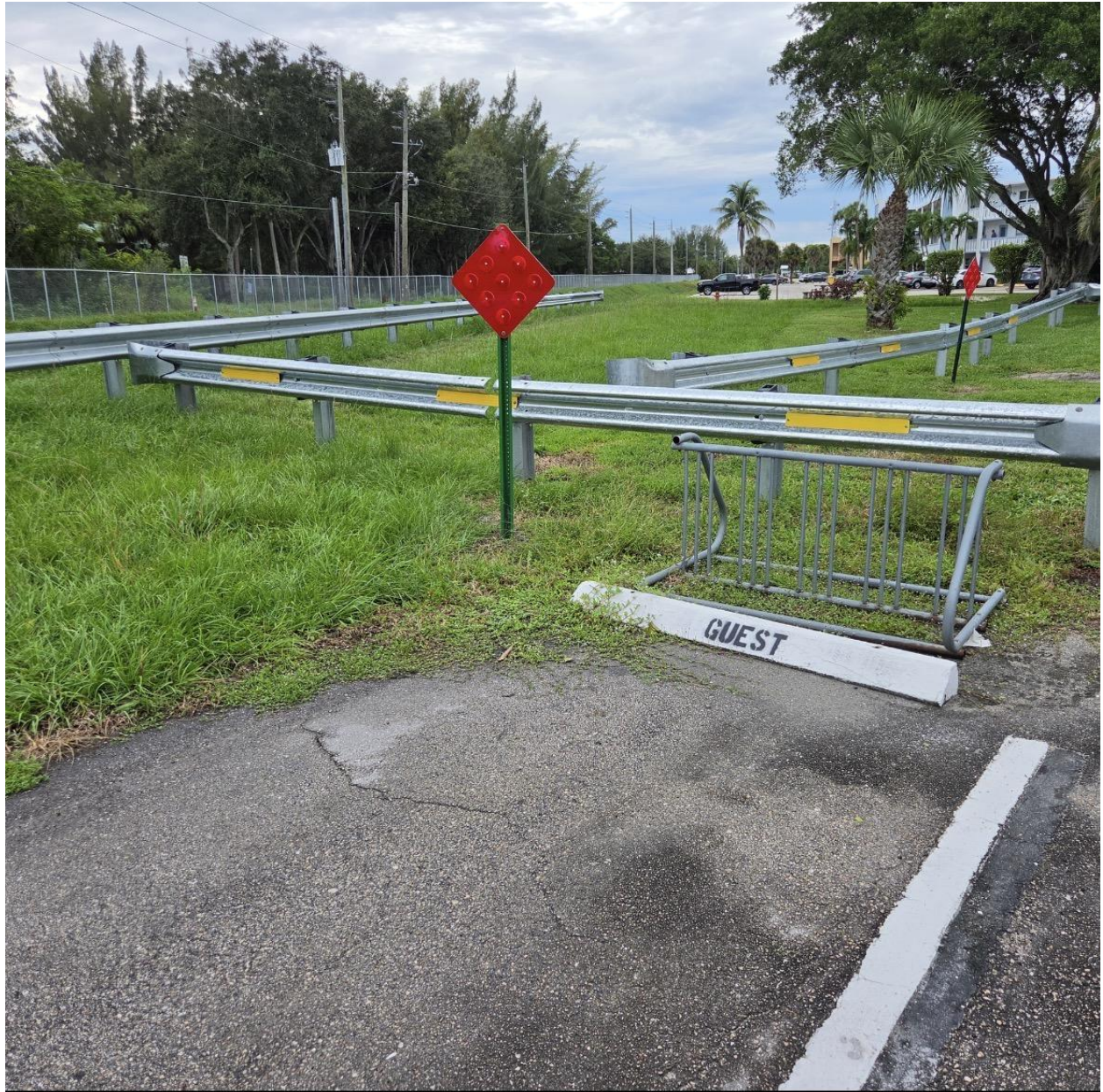
ANDOVER, WELLINGTON SECTIONS- JOSE INSTALLED ADDITIONAL REFLECTIVE STRIPS ON THESE NEW GUARDRAILS.
