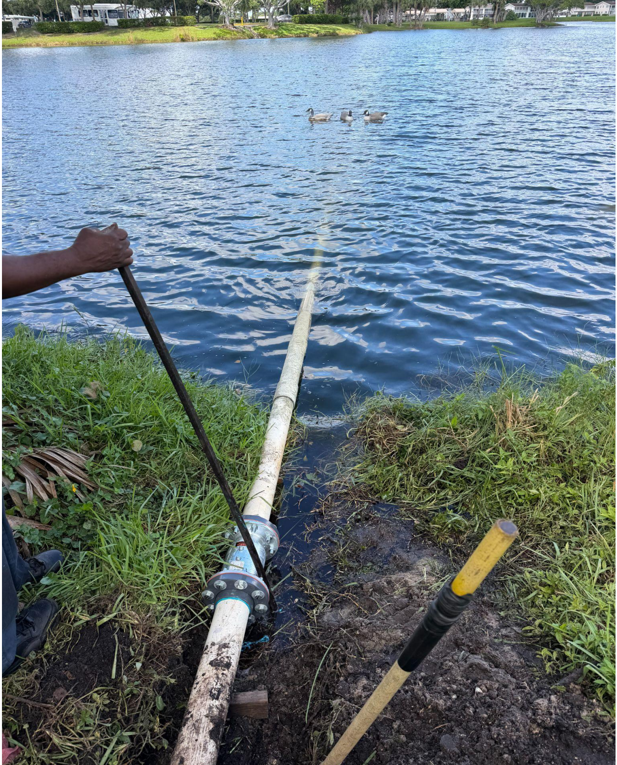
STRATFORD A- NEW CHECK VALVE INSTALLED ON IRRIGATION INTAKE PIPE BY CHABOT IRRIGATION.
