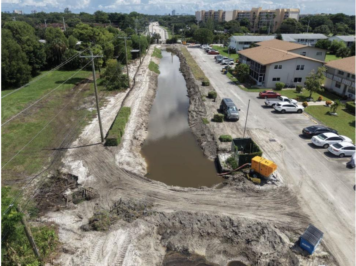
NORTH CANAL- DRONE'S EYE VIEW OF THE EASTERNMOST SECTION OF CANAL.
