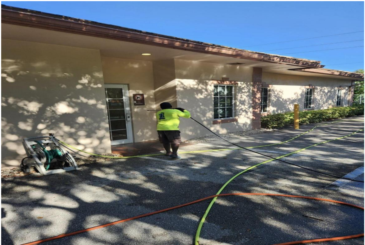
UCO OFFICE- EXTERIOR OF THE BUILDING WAS PRESSURE CLEANED ON 9/26.
