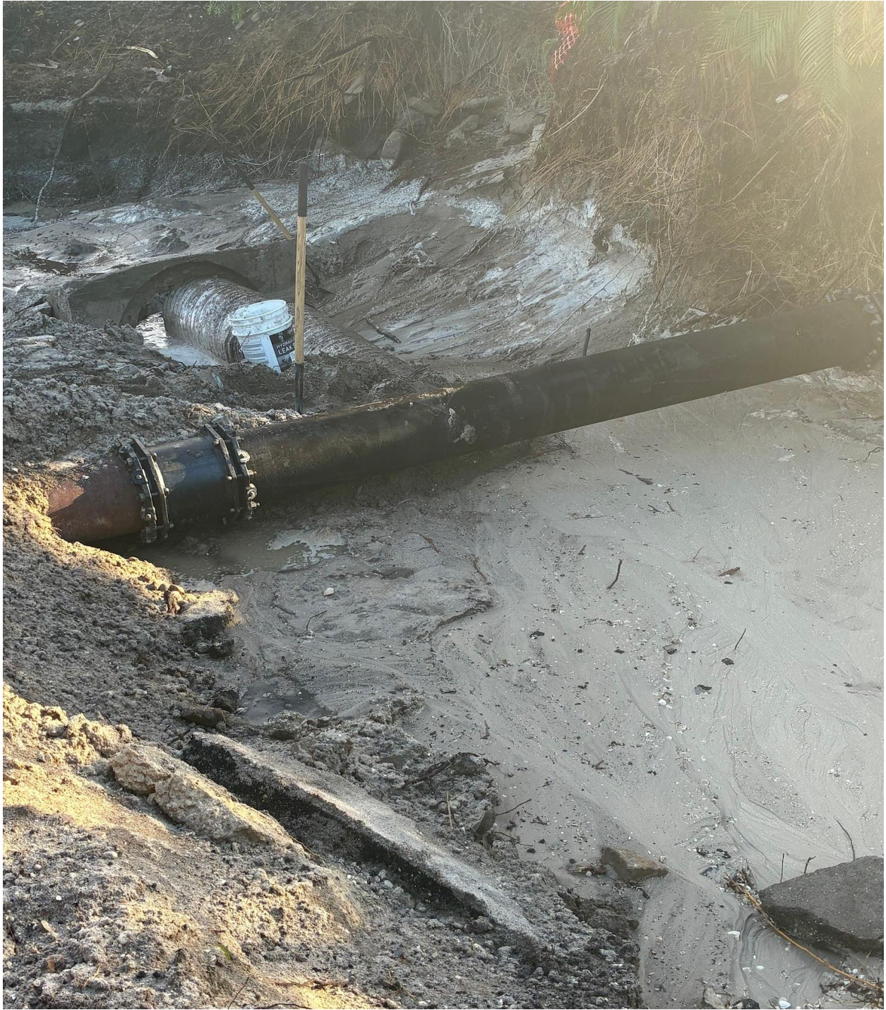
NORWICH SECTION- PERMANENT REPAIR TO THE WATER MAIN WAS COMPLETED ON 9/2.
