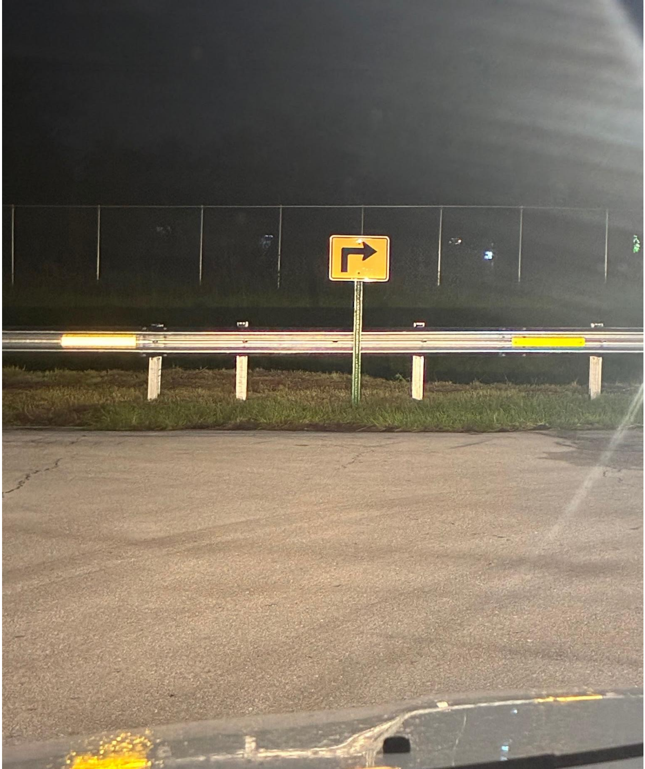
ANDOVER SECTION- NEW SIGN INSTALLED BY HANDYMAN JOSE.
