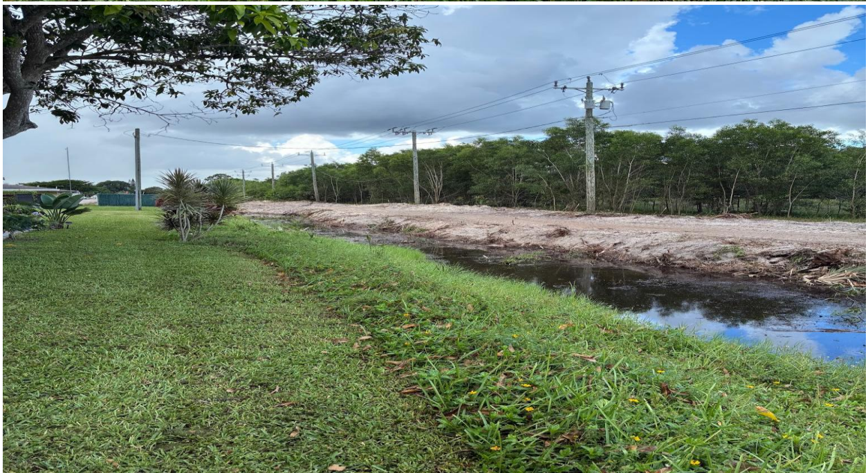
NORTH CANAL- LAND CLEARING WORK AT NORTH CANAL CONTINUES.
