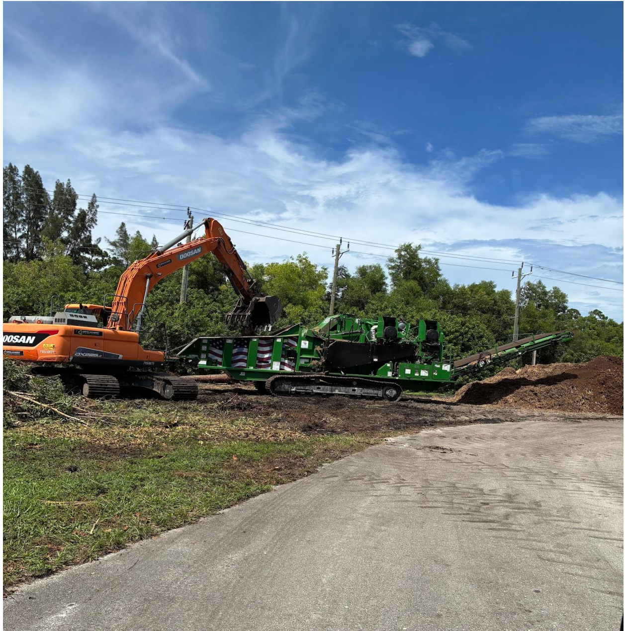
NORTH CANAL- LAND CLEARING WORK, BY JFB CONSTRUCTION, CONTINUES.
