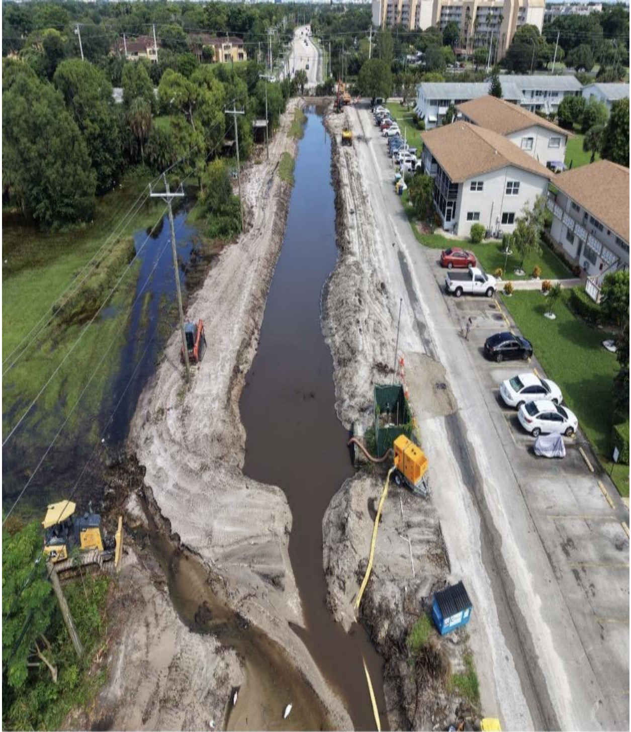
NORTH CANAL- DRONE'S EYE VIEW OF THE EASTERNMOST SECTION.
