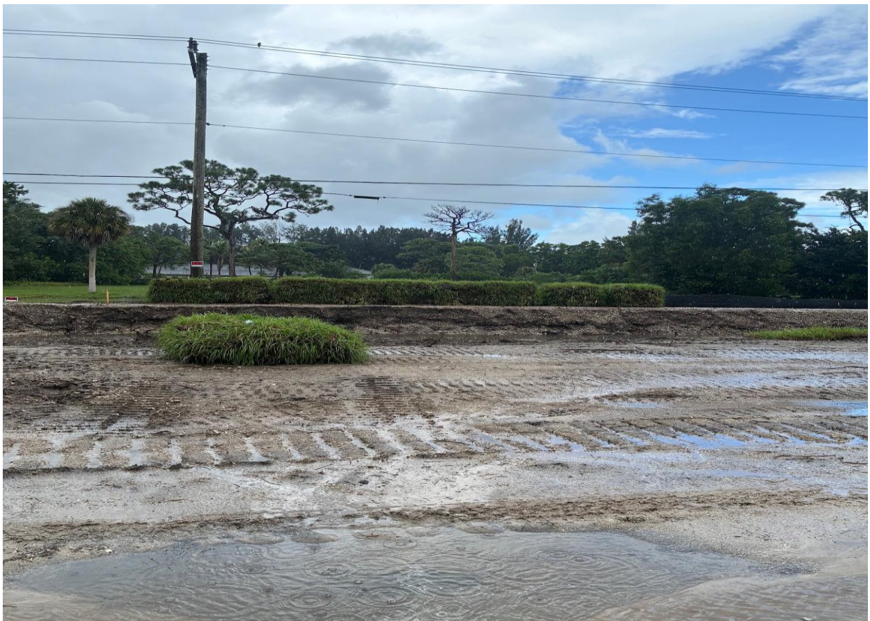
NORWICH/COVENTRY SECTIONS- SOD IS BEING INSTALLED ON BOTH SIDES OF THE CANAL.
