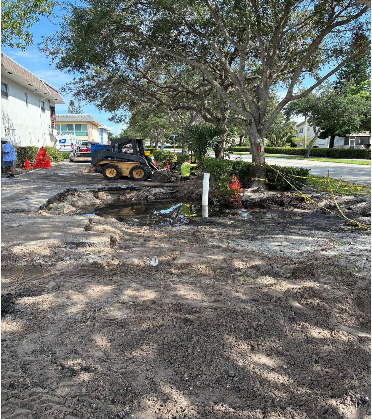
STRATFORD A- ON 9/21, FEDERAL MAINTENANCE BEGAN REPAIR OF THE GIANT CRATER.
