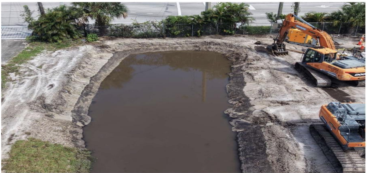
NORTH CANAL- DRONE'S EYE VIEWS OF THE EASTERNMOST SECTION.
