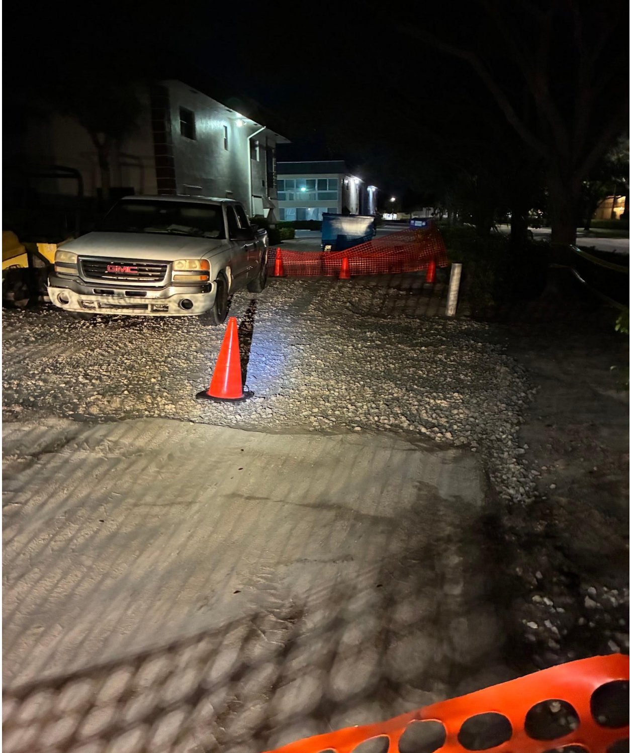
STRATFORD A- THE GIANT CRATER IS BACKFILLED AND COMPACTED. PAVING WILL NEED TO WAIT UNTIL THE GROUND DRIES OUT.
