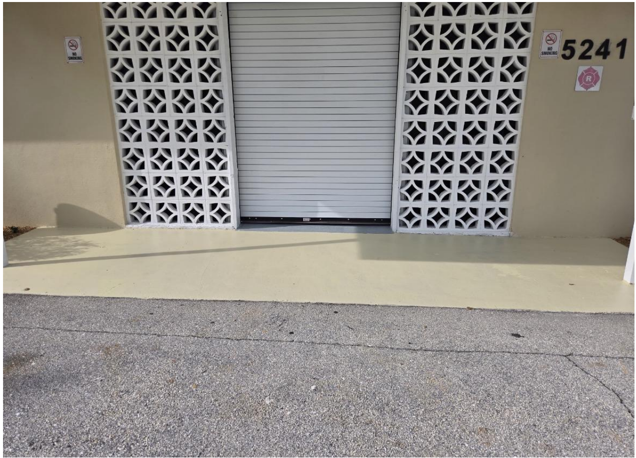
PLYMOUTH LAUNDRY- THE FRONT ENTRANCE FLOOR WAS REPAINTED BY HANDYMAN JOSE.
