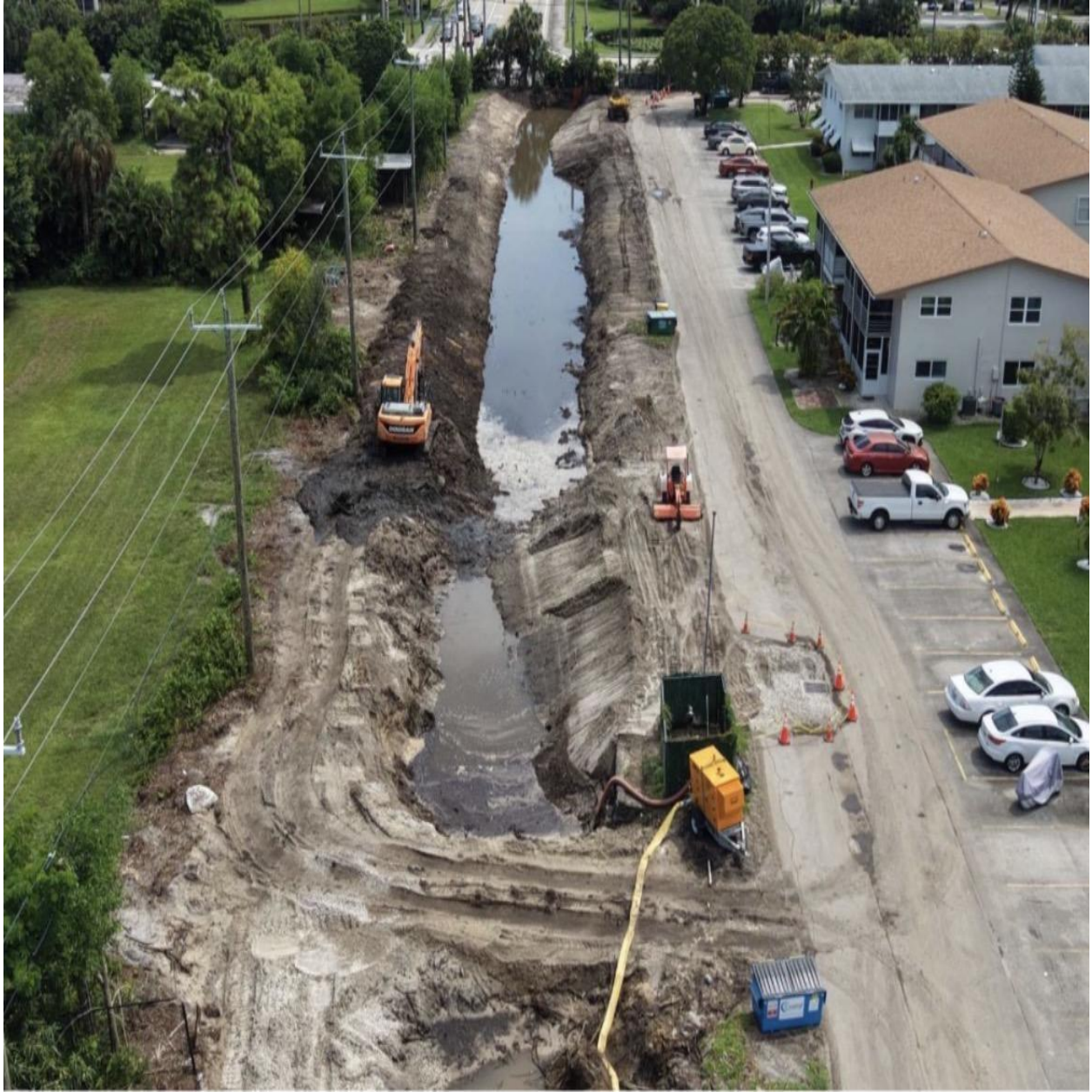
NORTH CANAL- A DKK PROJECT MANAGER USED A DRONE TO GET BIRD'S EYE PICTURES OF THE ONGOING WORK.
