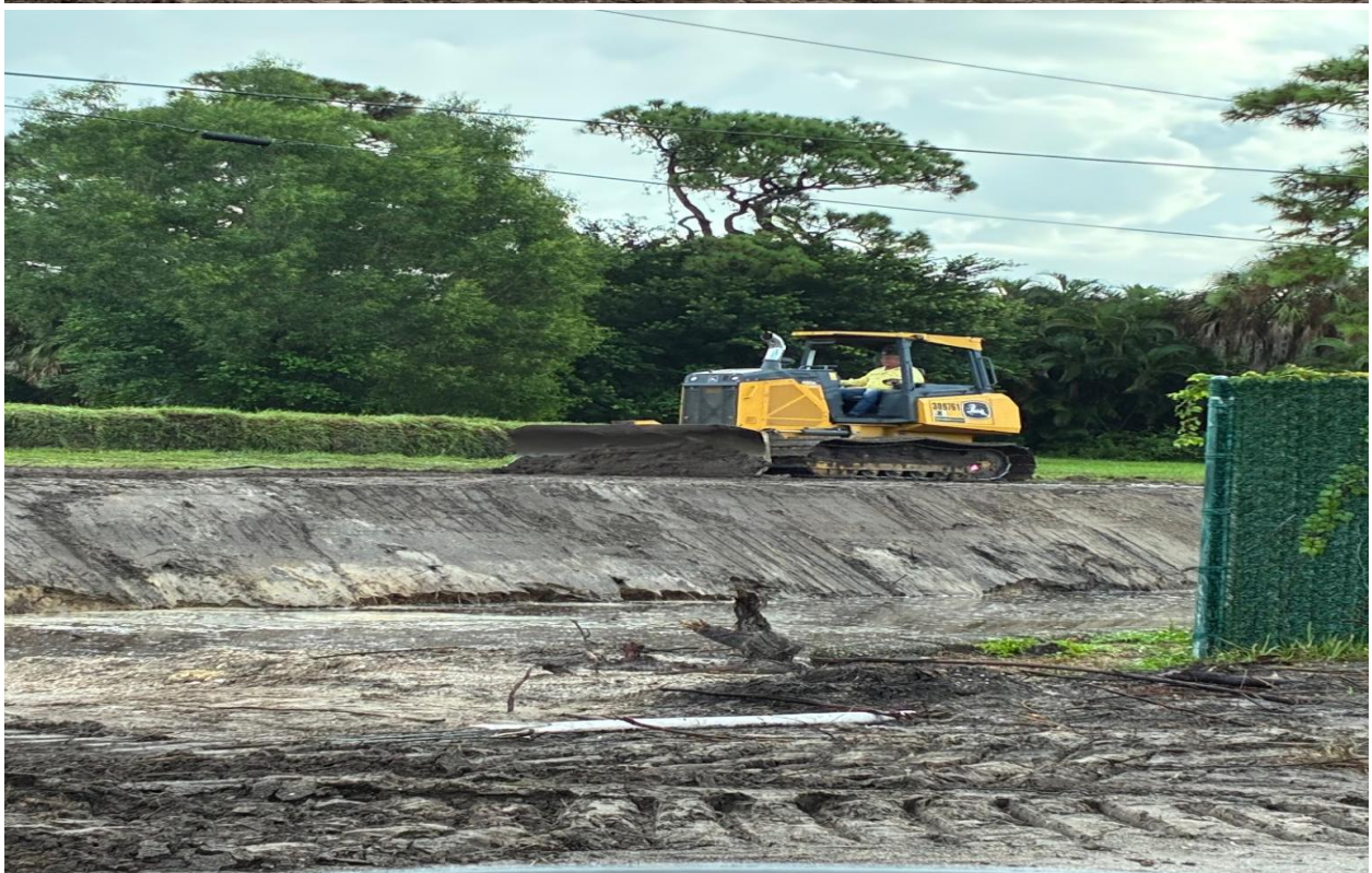
NORTH CANAL- JFB CONSTRUCTION BEGAN LAYING DOWN SOD AT THE EASTERNMOST SECTION ON 9/16.
