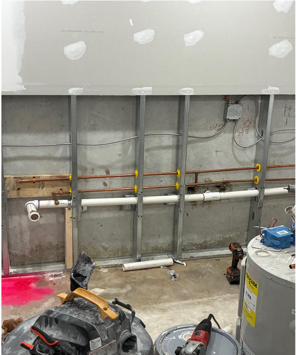
121 WELLINGTON G- KITCHEN REDESIGN. THIS REQUIRES PERMIT AND WRITTEN PERMISSION FROM THE BOARD BEFORE WORK STARTS.
