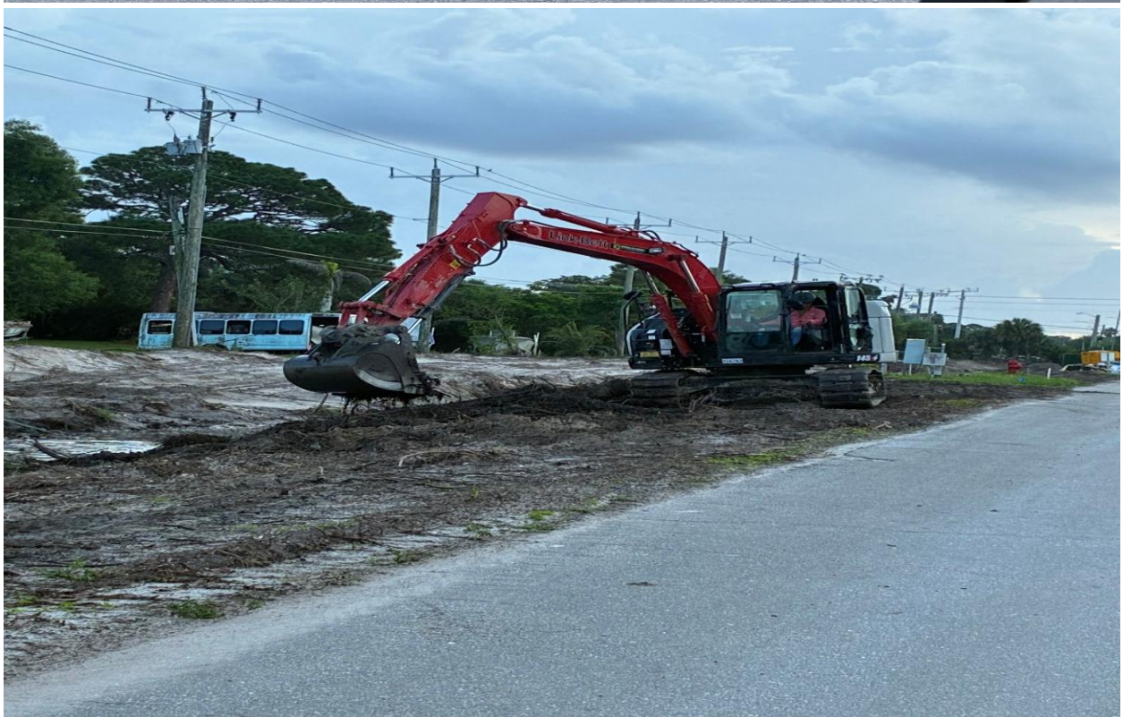
COVENTRY SECTION- DREDGING AND REGRADING WORK BY JFB CONSTRUCTION CONTINUES.
