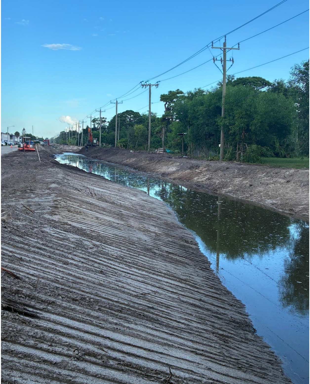
NORWICH SECTION- DREDGING AND REGRADING WORK BY JFB CONSTRUCTION CONTINUES.
