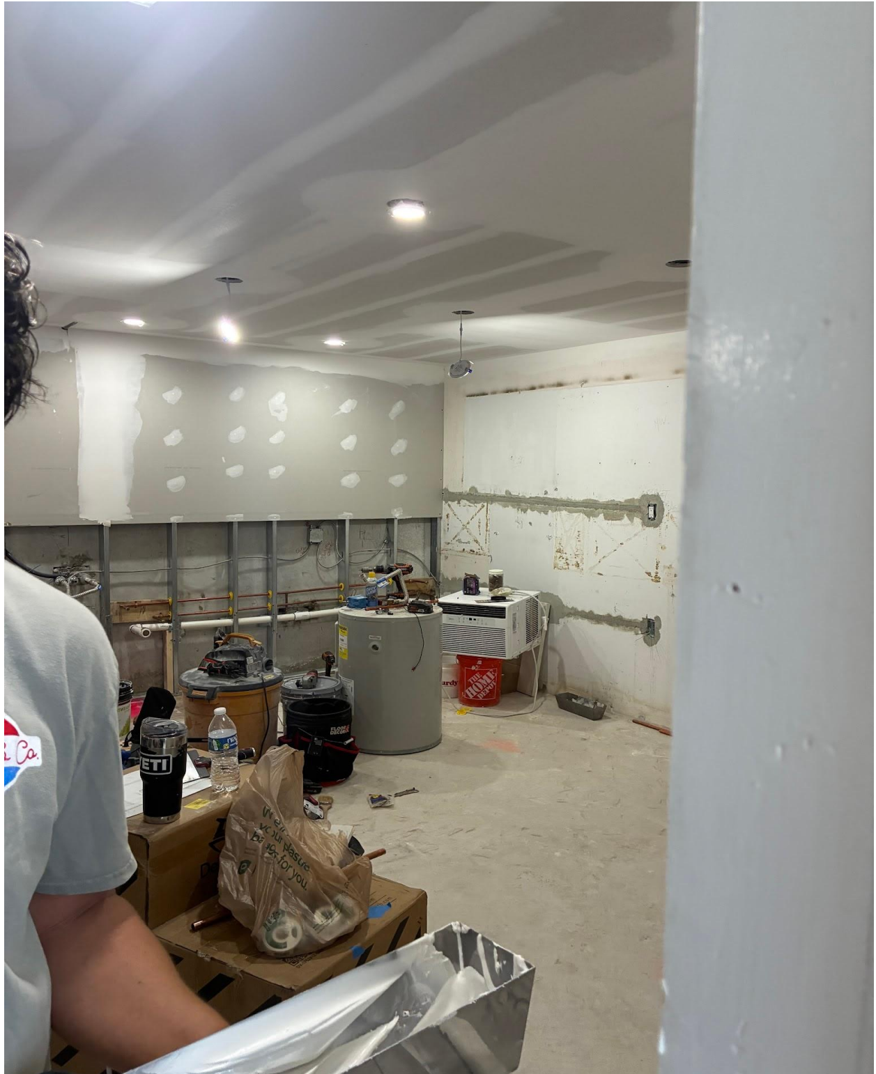
121 WELLINGTON G- KITCHEN REDESIGN, ELECTRICAL WORK, SUSPENDED CEILING AND RECESSED LIGHTING INSTALLED. THE ORIGINAL KITCHEN WALL WAS REMOVED.
