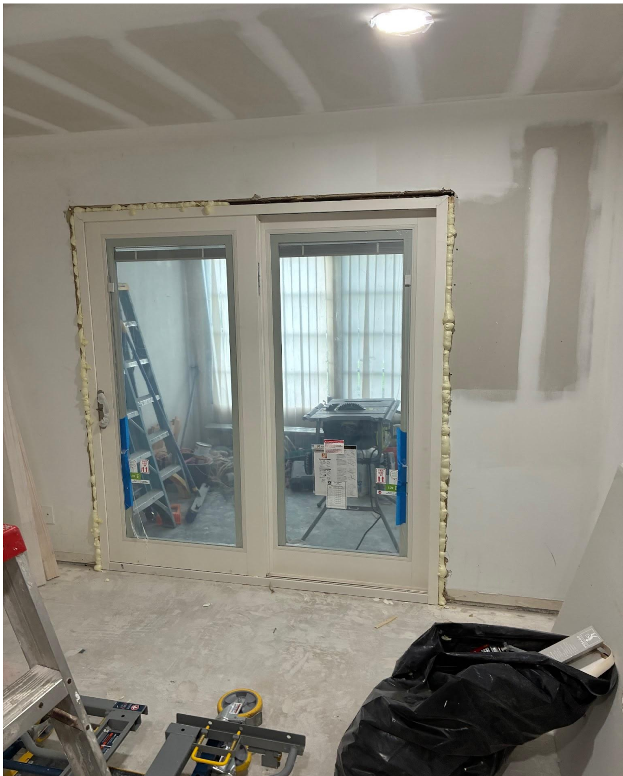
121 WELLINGTON G- NEW EXTERIOR DOORS INSTALLED. THIS REQUIRES PERMIT, AND SPECIFICATIONS FOR THE DOORS MUST BE SENT TO THE ASSOCIATION PRIOR TO INSTALLATION.
