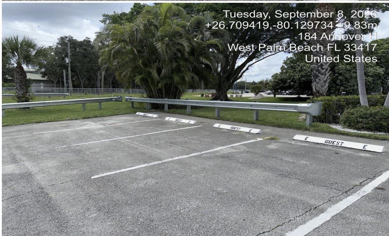
SOUTH CANAL- GUARDRAILS WERE INSTALLED NEAR ANDOVER H AND WELLINGTON E.
