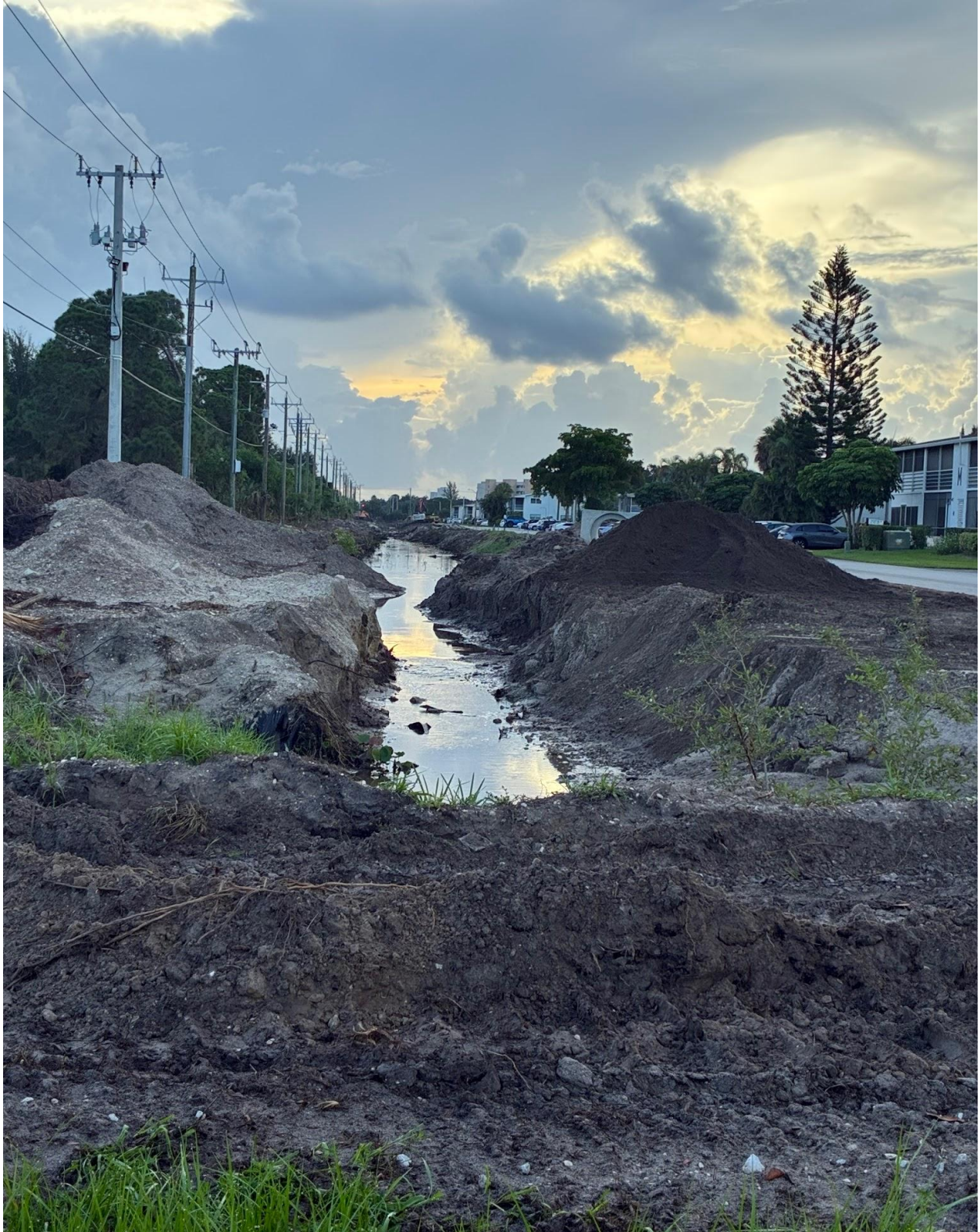
SHEFFIELD SECTION- DREDGING AND REGRADING WORK BY JFB CONSTRUCTION CONTINUES.
