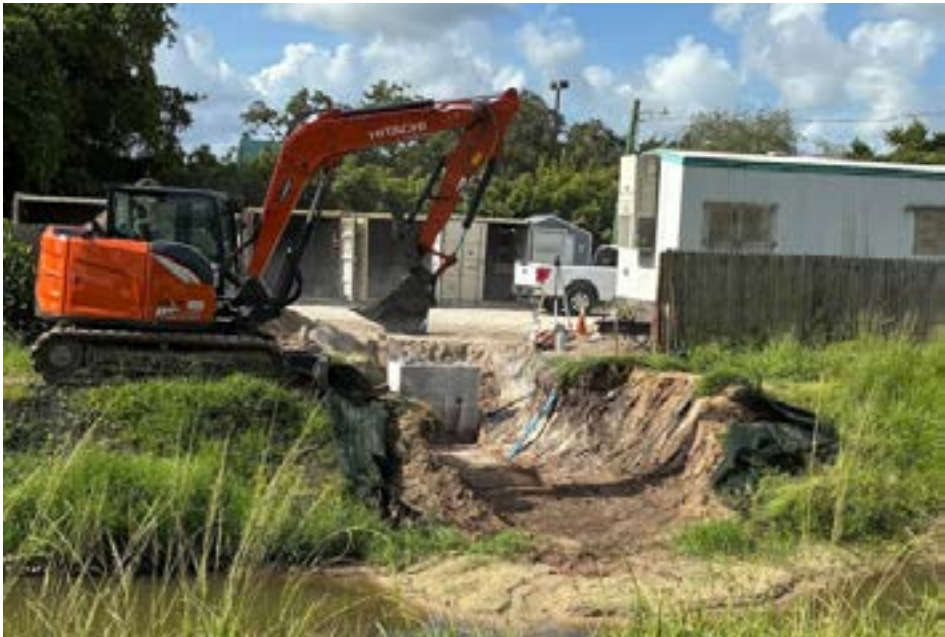
SOUTH CANAL- NEW DRAIN BEING INSTALLED AT BEDFORD SECTION
