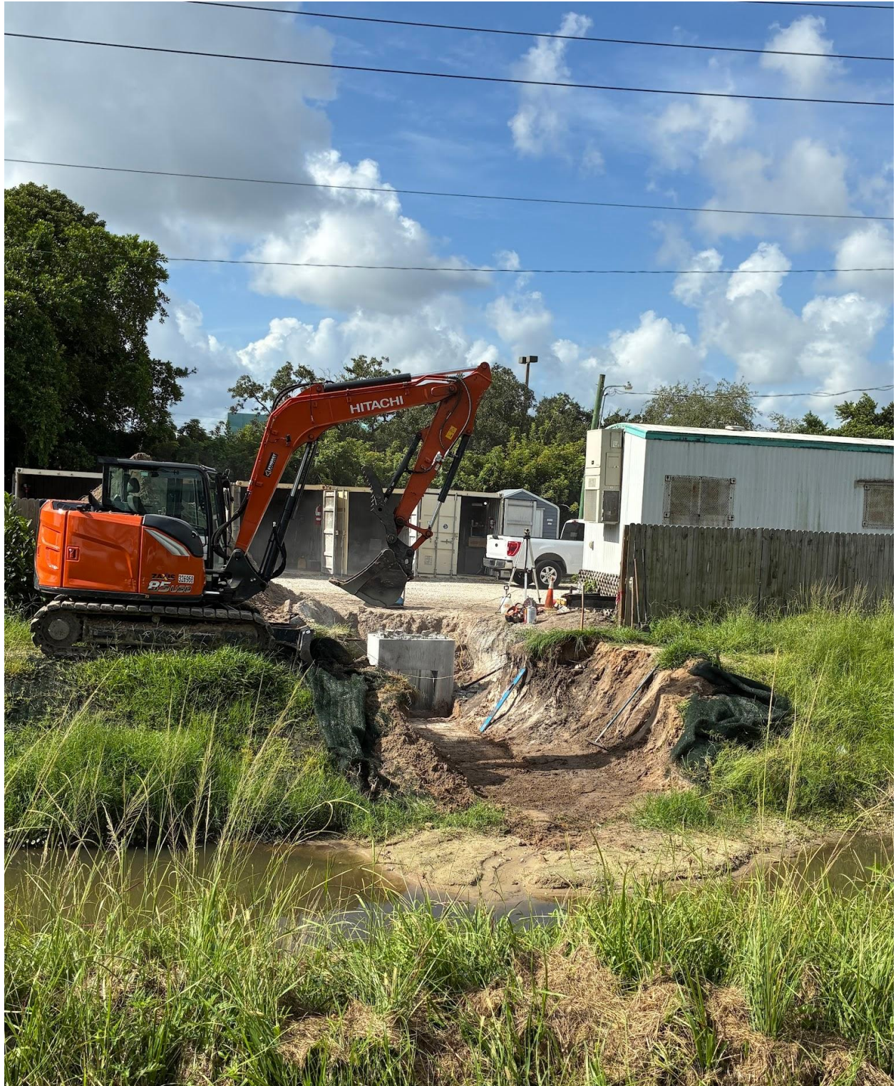
SOUTH CANAL- EXCAVATION CONTINUED ON 8/24.
