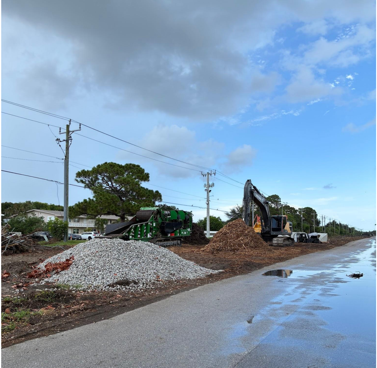
NORTH CANAL- LAND CLEARING, TREE/PALM GRINDING, AND REMOVAL CONTINUES. THIS IS AT SHEFFIELD SECTION.
