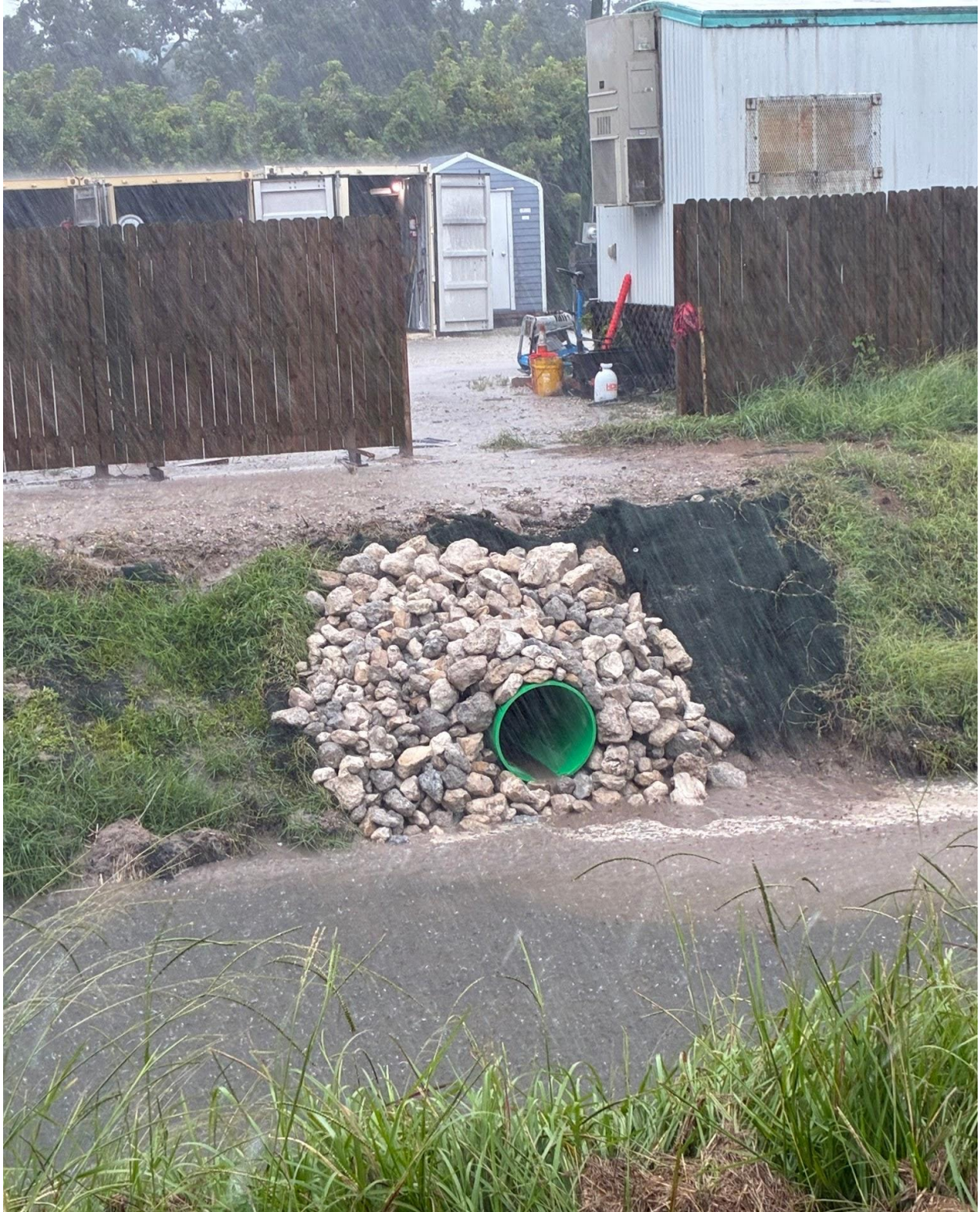
NORTH CANAL- DRAIN INSTALLATION CONTINUED ON 8/26.
