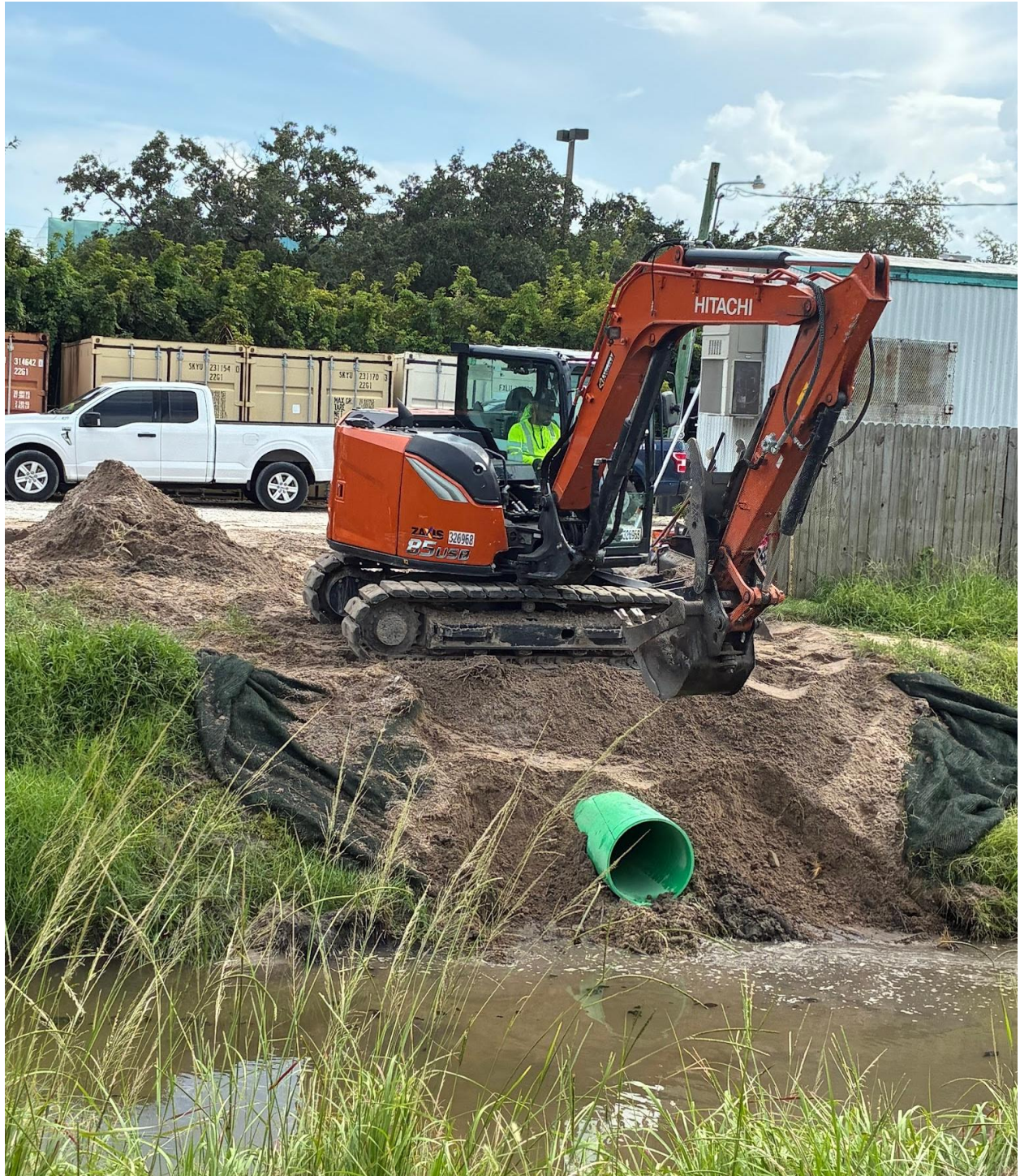
NORTH CANAL- NEW DRAINPIPE INSTALLED ON 8/25.
