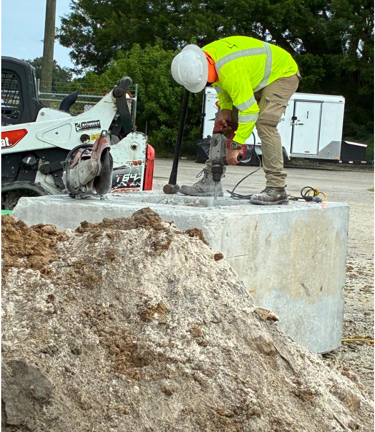
SEACREST COMPOUND- THIS CONCRETE BOX WILL BE THE NEW STORM DRAIN, DRAINING INTO NORTH CANAL OPPOSITE BEDFORD K.
