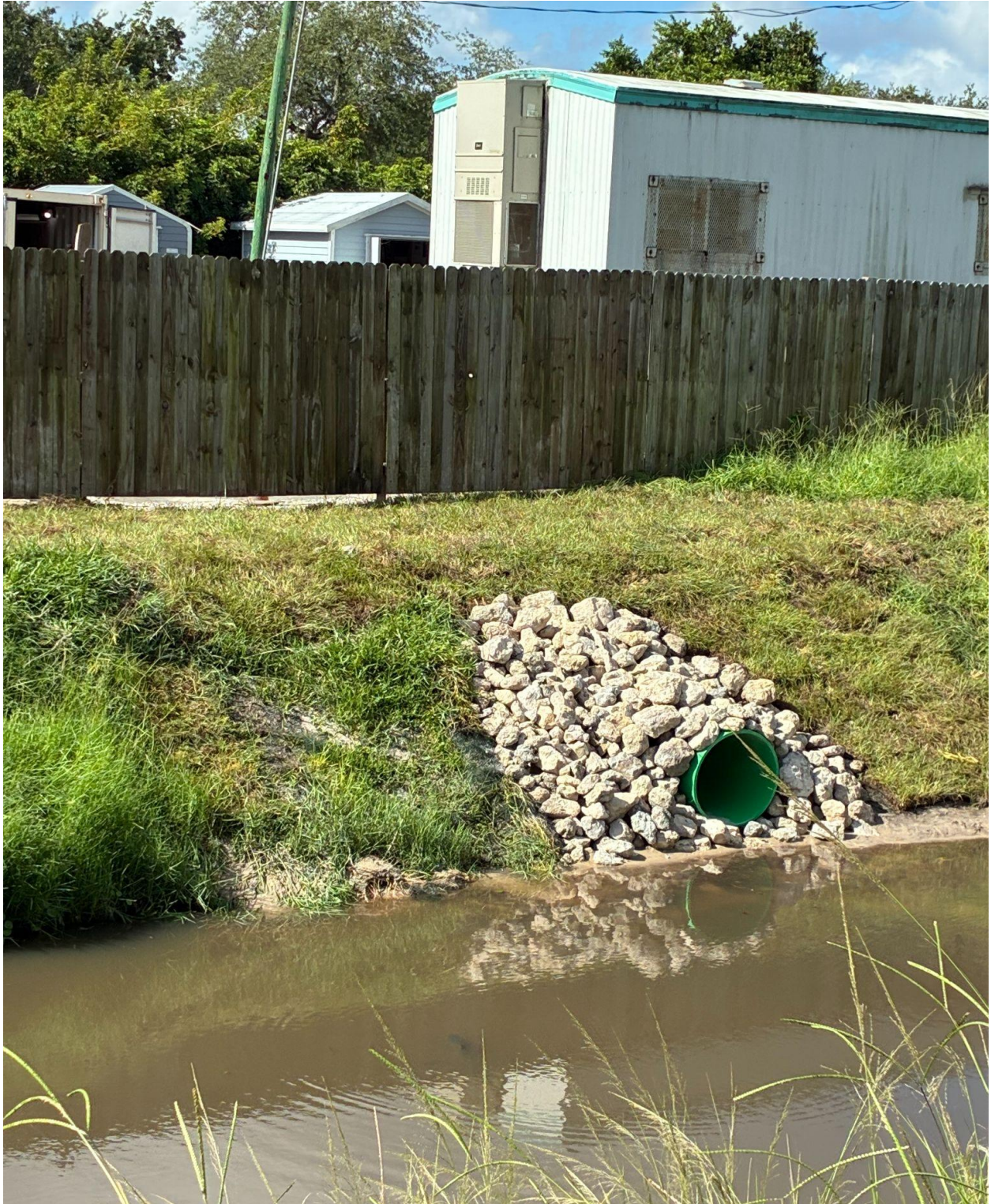
NORTH CANAL- DRAIN INSTALLATION COMPLETE ON 8/27.
