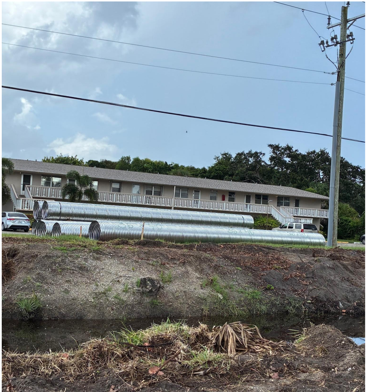
NORTH CANAL- BUILDING MATERIALS STAGED FOR INSTALLATION BY JFB CONSTRUCTION. THIS IS AT HASTINGS SECTION.
