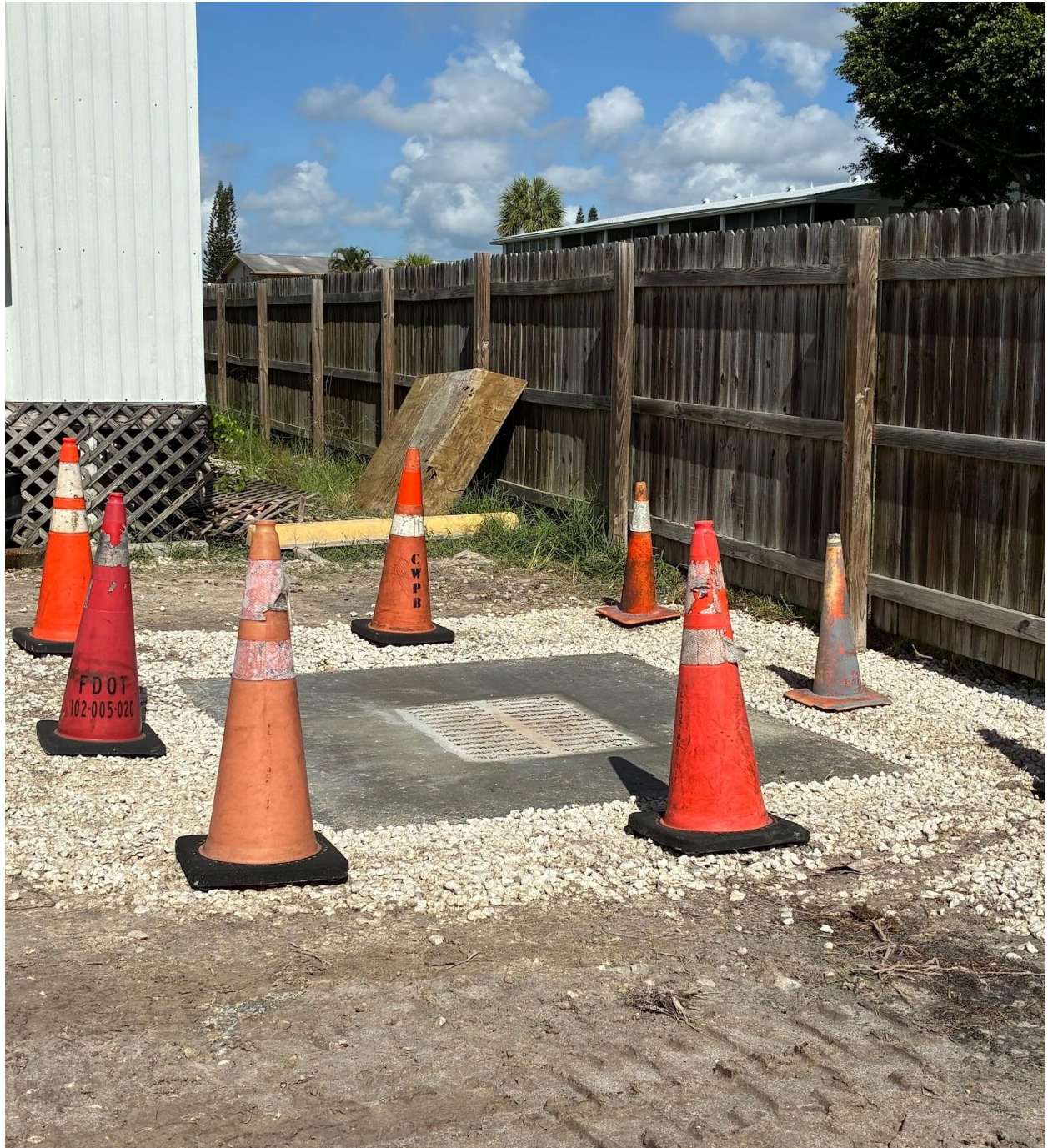
SEACREST COMPOUND- A FOUR-SIDED RAILING WILL BE INSTALLED AROUND THIS NEW CATCH BASIN TO KEEP CARS AND DEBRIS OFF OF IT.
