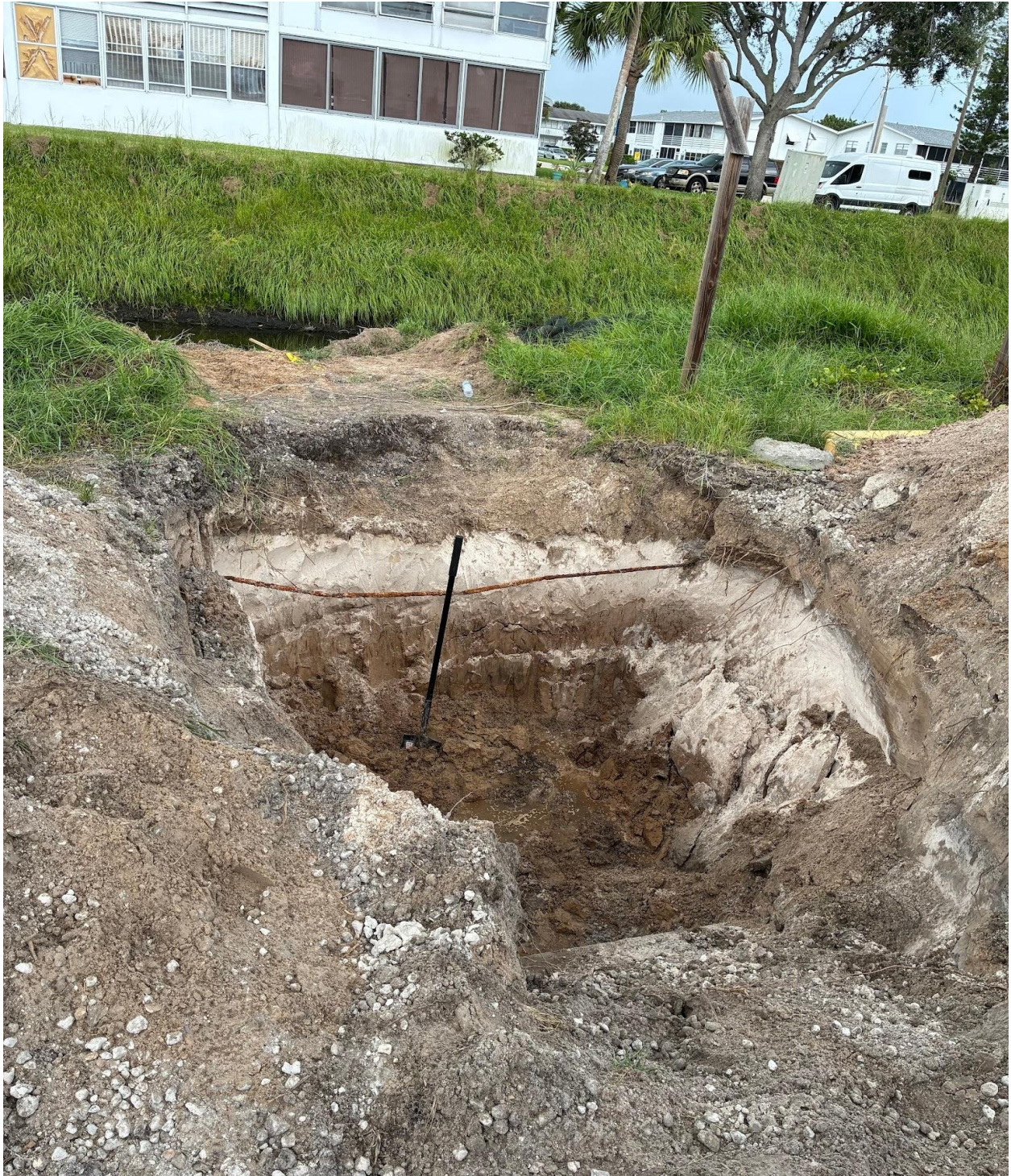
SEACREST COMPOUND- THE HOLE FOR THE NEW STORM DRAIN WAS EXCAVATED ON 8/24.
