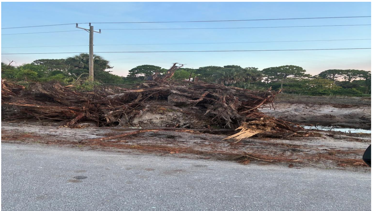
NORTH CANAL- LAND CLEARING WORK CONTINUED LAST WEEK.
