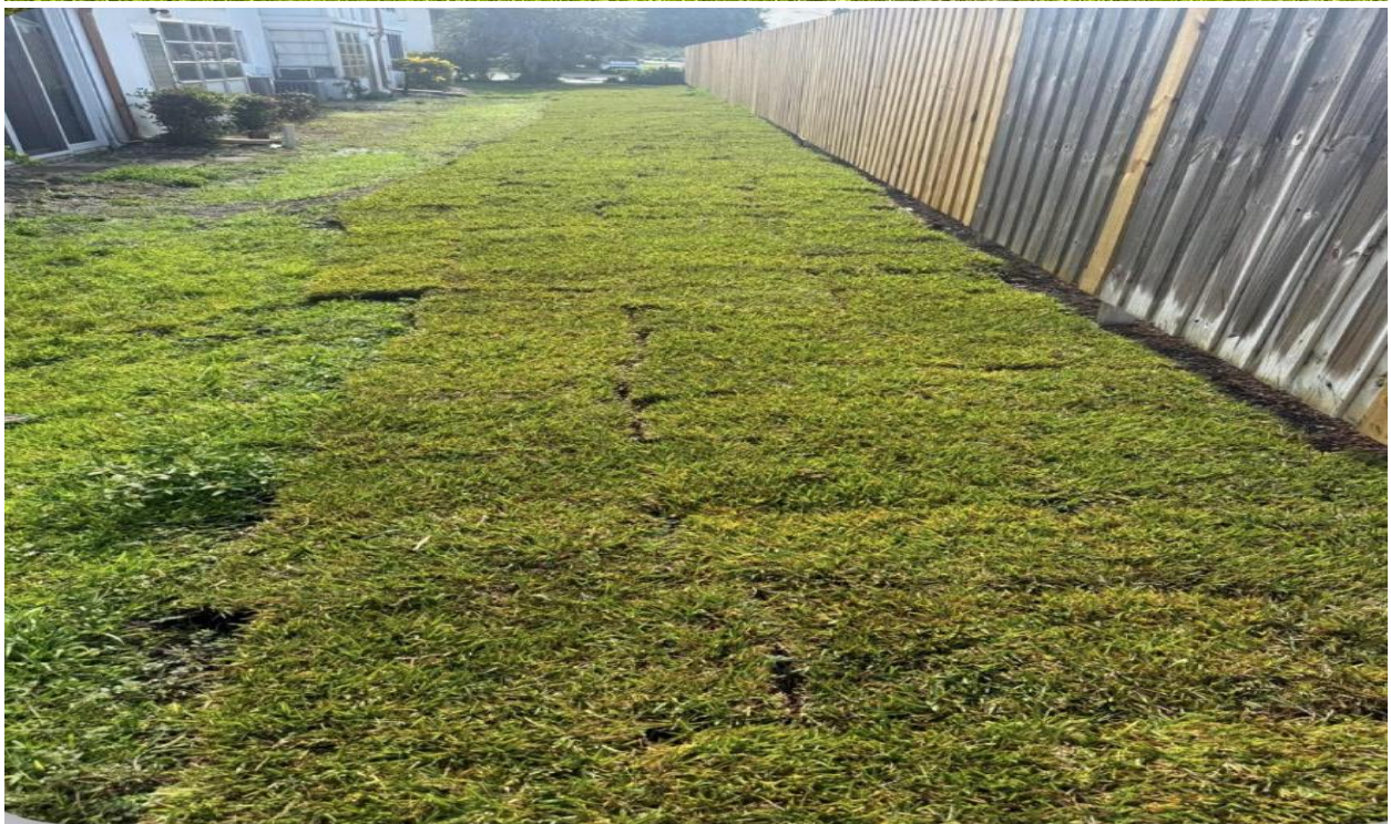
PLYMOUTH LAUNDRY- SOD WAS INSTALLED ON 8/6.
