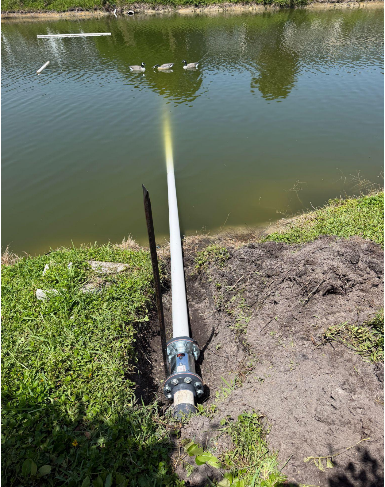
BEDFORD SECTION- NEW INTAKE PIPE AND CHECK VALVE INSTALLED BY CHABOT IRRIGATION.
