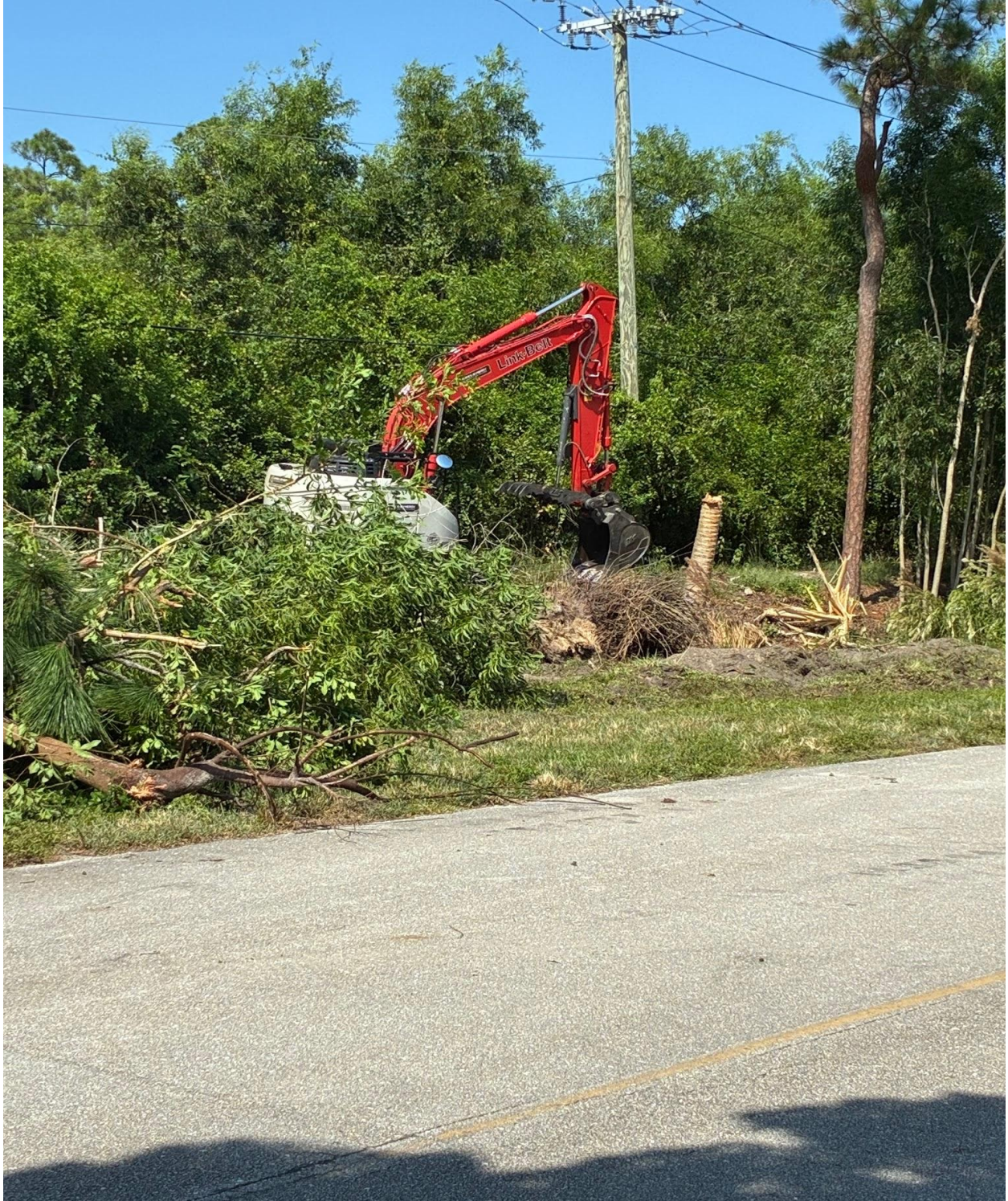
NORTH CANAL- LAND CLEARING WORK HAS BEGUN AT THE WESTERN END OF THE CANAL.
