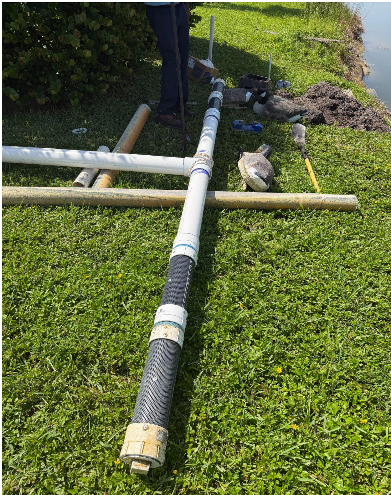
BEDFORD SECTION- NEW INTAKE PIPES AND SCREENS INSTALLED BY CHABOT IRRIGATION.
