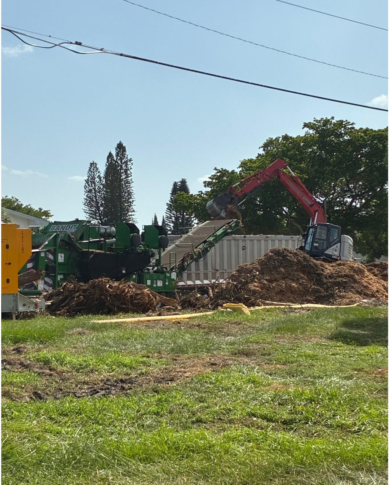
NORTH CANAL- LAND CLEARING, GRINDING, AND REMOVAL WORK CONTINUES.
