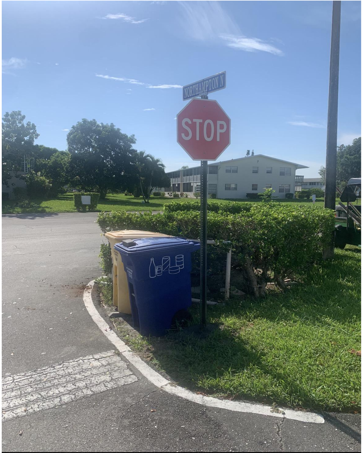
NORTHAMPTON SECTION- FADED STOP SIGN REPLACED BY HANDYMAN JOSE.
