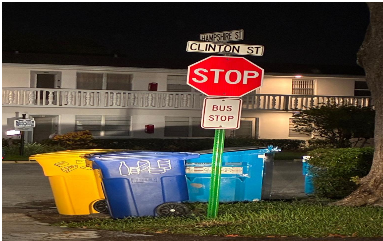
CHATHAM SECTION- FADED STOP SIGN REPLACED BY HANDYMAN JOSE.
