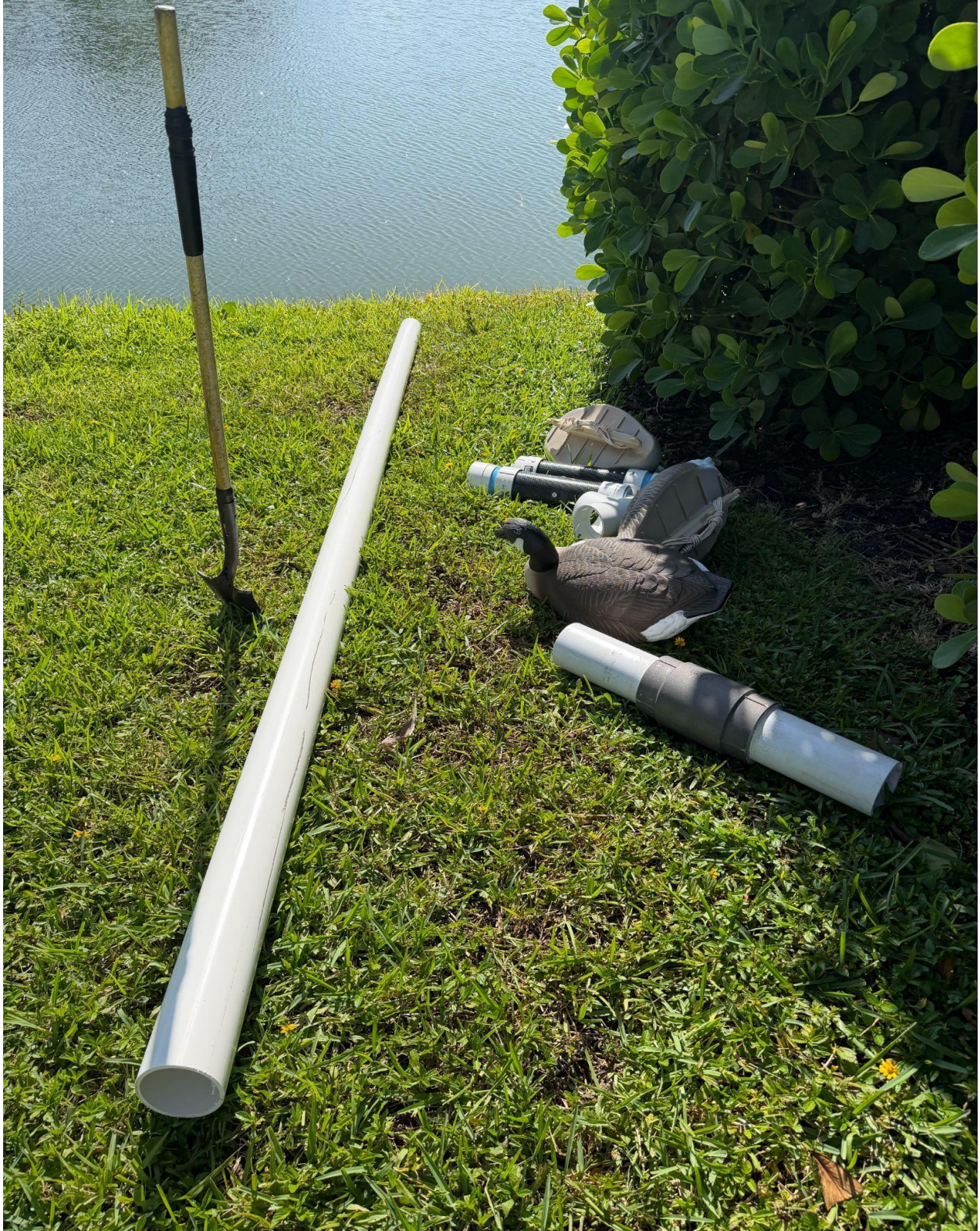
CHATHAM SECTION- NEW INTAKE PIPE AND SCREENS INSTALLED BY CHABOT IRRIGATION.
