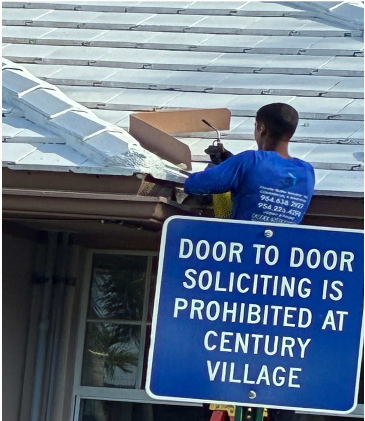
OKEECHOBEE BOULEVARD GUARDHOUSE- SMASHED RAIN GUTTERS WERE REPAIRED BY GUTTER SOLUTIONS ON 8/21.
