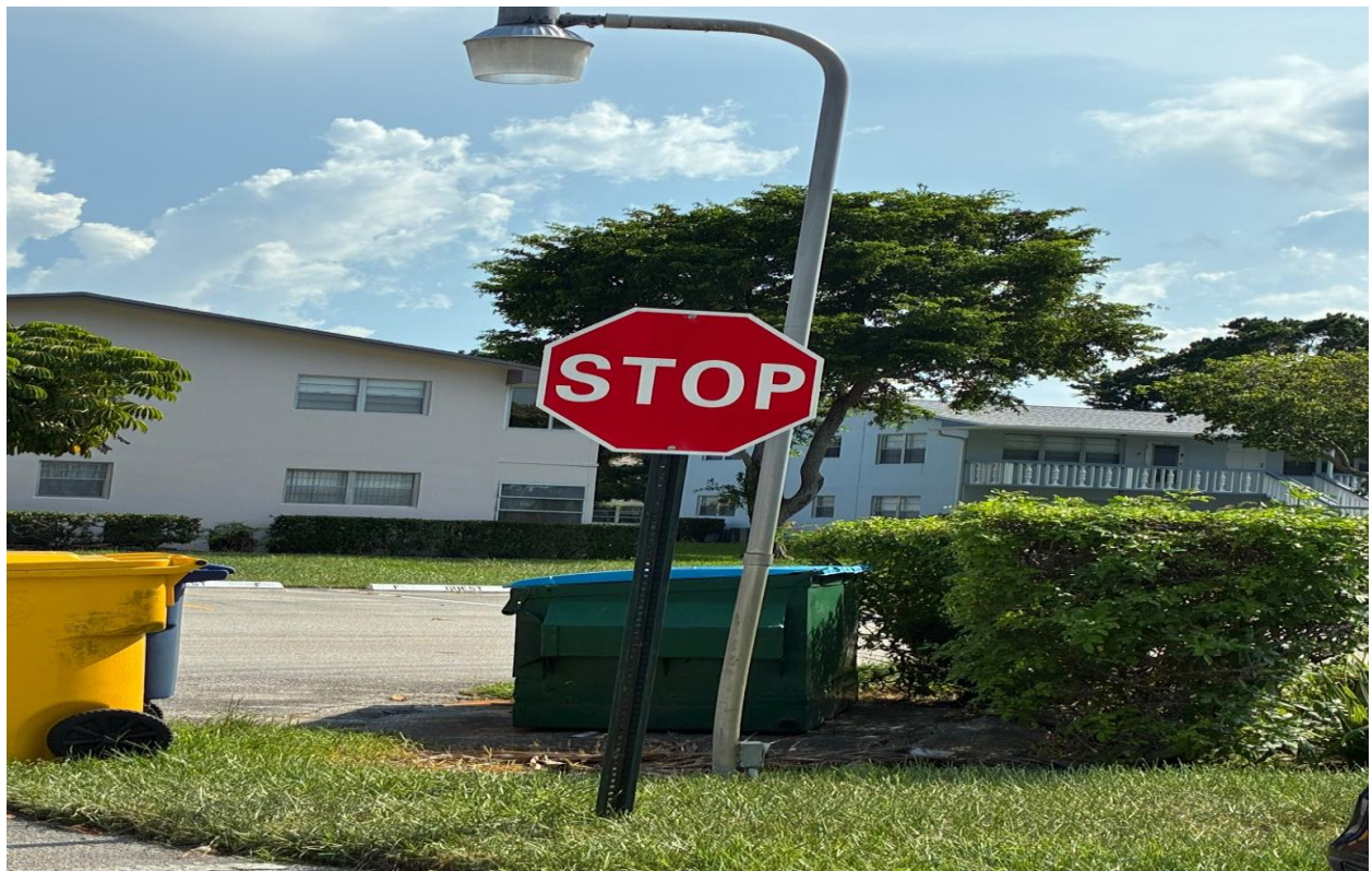
CANTERBURY SECTION- FADED STOP SIGN REPLACED BY HANDYMAN JOSE.
