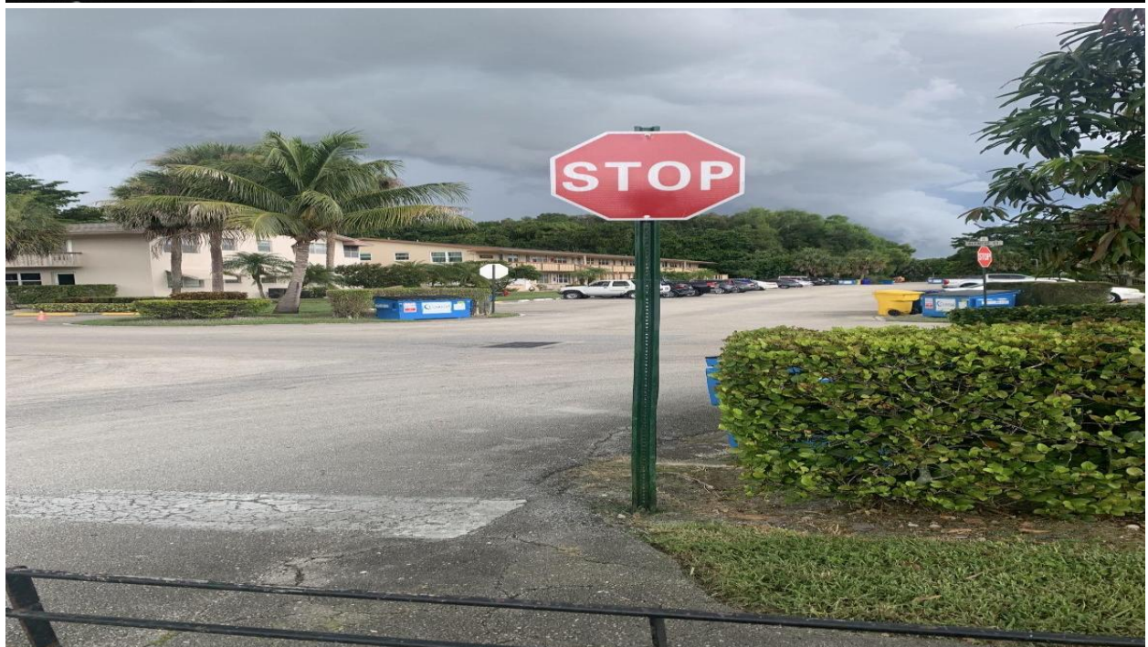
HASTINGS SECTION- FADED STOP SIGN REPLACED BY HANDYMAN JOSE.
