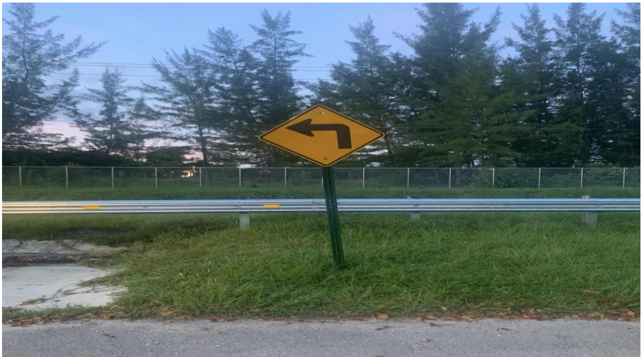
WINDSOR SECTION- FADED DIRECTIONAL SIGN REPLACED BY HANDYMAN JOSE.
