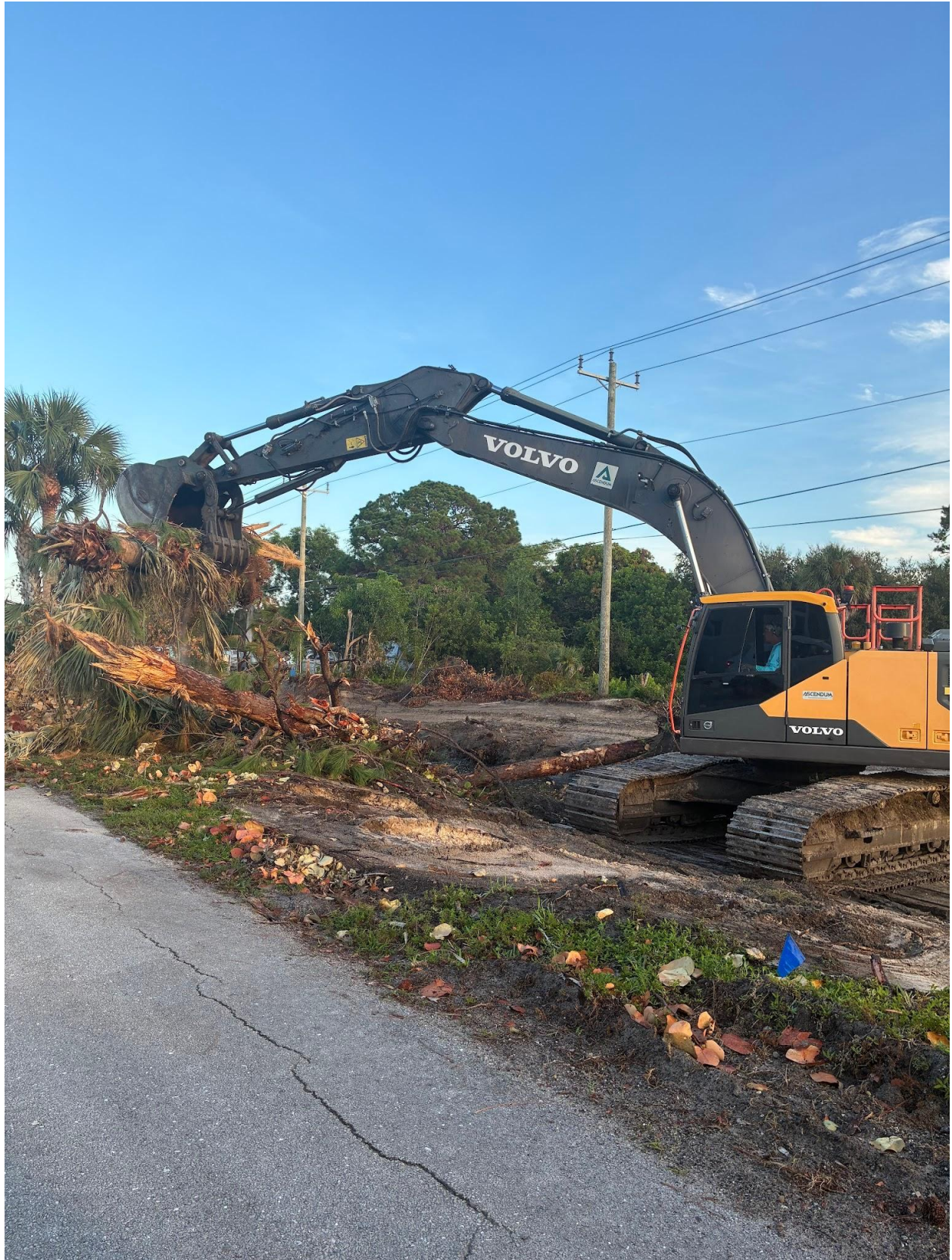
NORTH CANAL- LAND CLEARING WORK CONTINUES.
