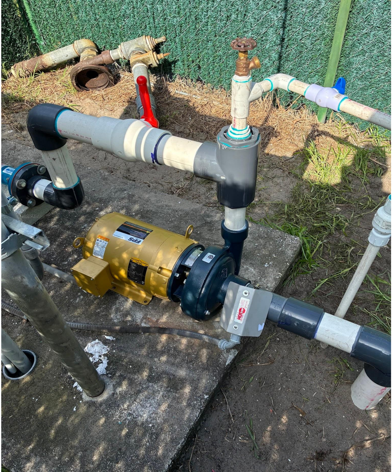
DORCHESTER POOL- CHABOT IRRIGATION INSTALLED A NEW PUMP, PUMP MOTOR, “HOT STOP” SWITCH, PIPES, VALVES, AND ELECTRICAL COMPONENTS.
