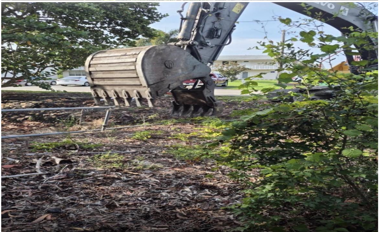
NORTH CANAL- LAND CLEARING AND EXCAVATION WORK BEGAN ON 7/29.
