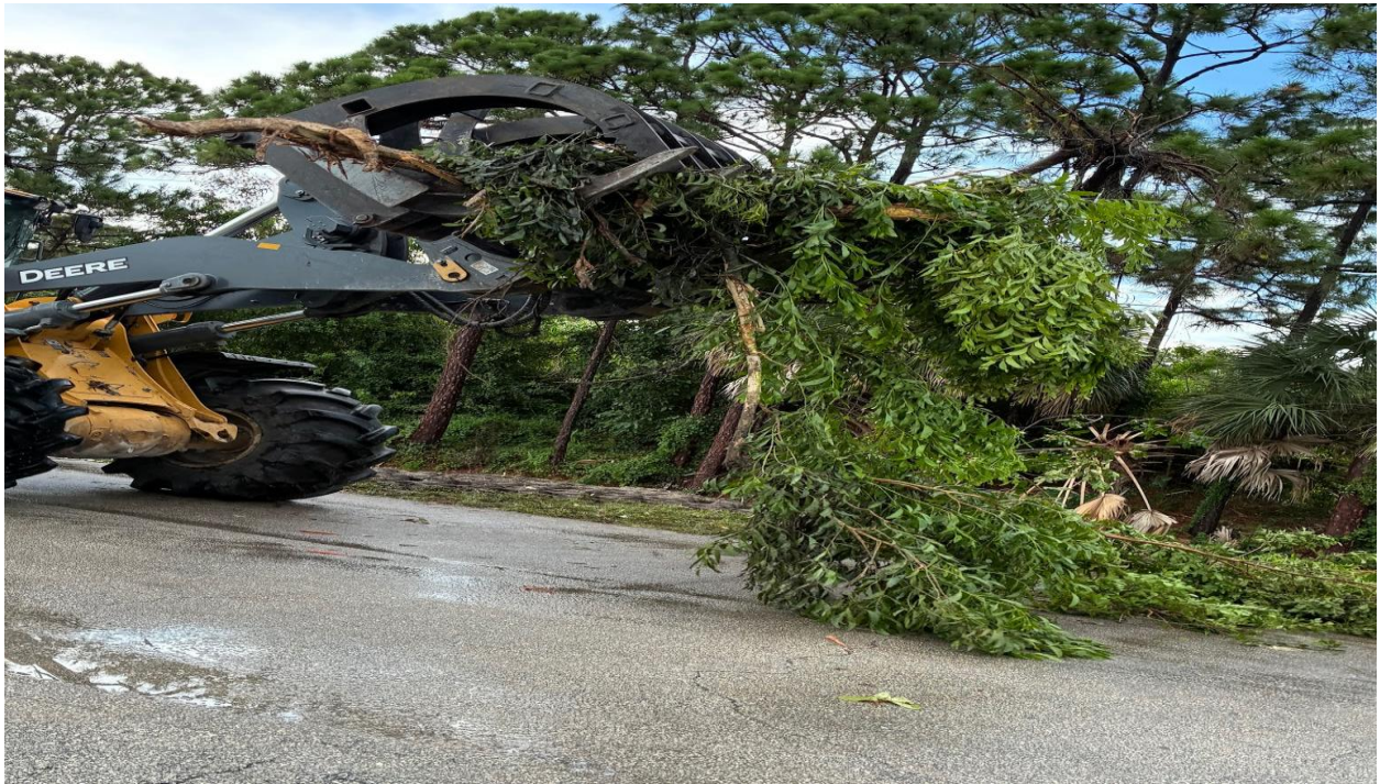
NORTH CANAL- SIXTY YEARS OF OVERGROWN JUNGLE IS BEING REMOVED FROM BOTH SIDES OF THE CANAL.
