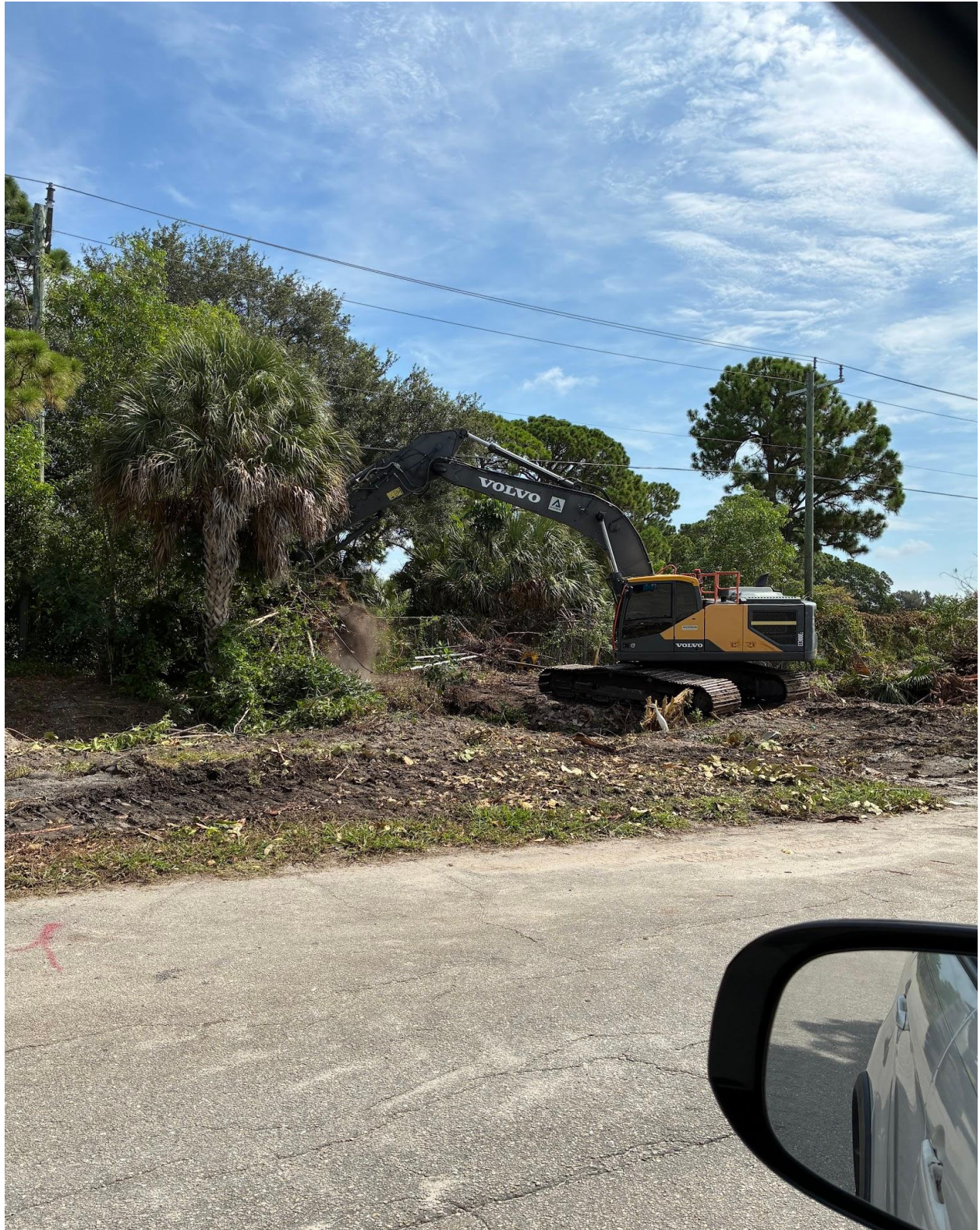
NORTH CANAL- ALL TREES AND PALMS AT BOTH SIDES OF THE CANAL ARE BEING REMOVED.
