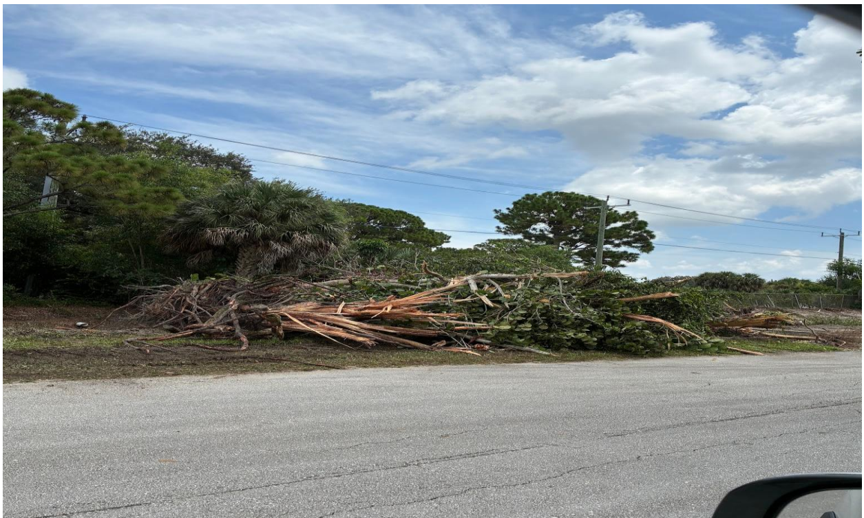
NORTH CANAL- SIXTY YEARS OF OVERGROWN JUNGLE IS BEING REMOVED ON BOTH SIDES OF THE CANAL.
