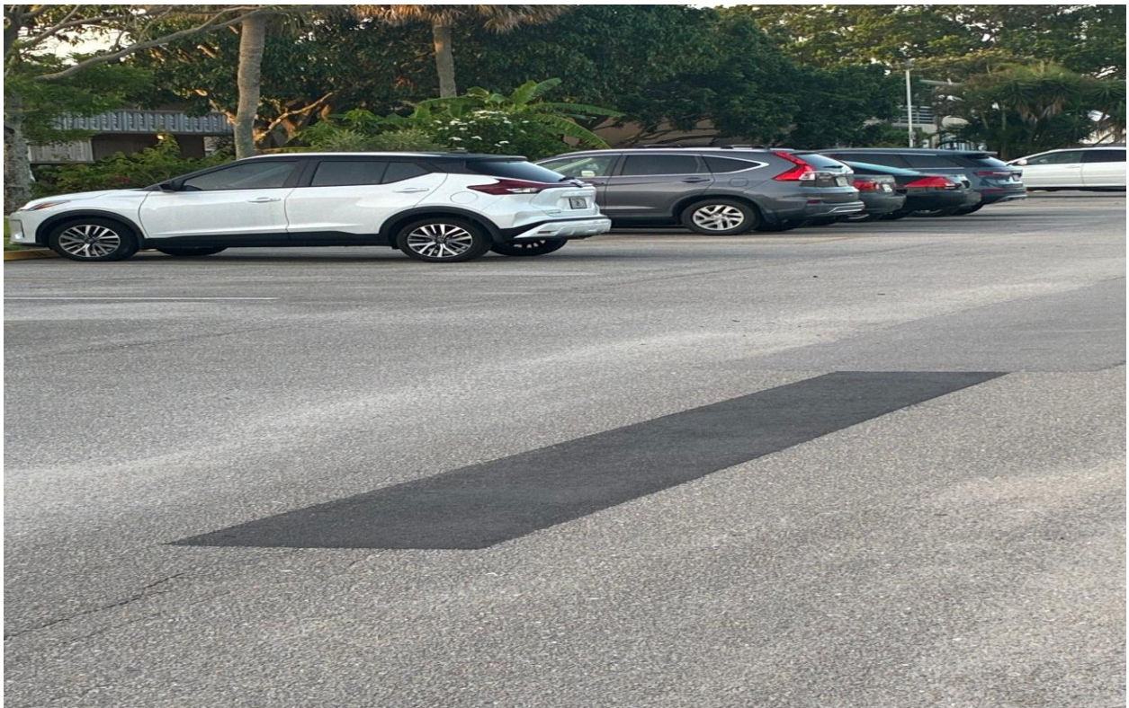
BEDFORD SECTION- ROAD REPAIRS COMPLETE.
