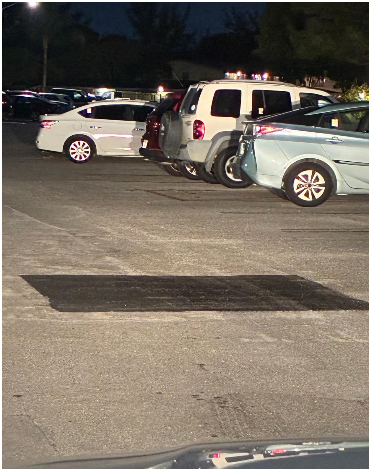
WINDSOR SECTION- ROAD REPAIR COMPLETE.
