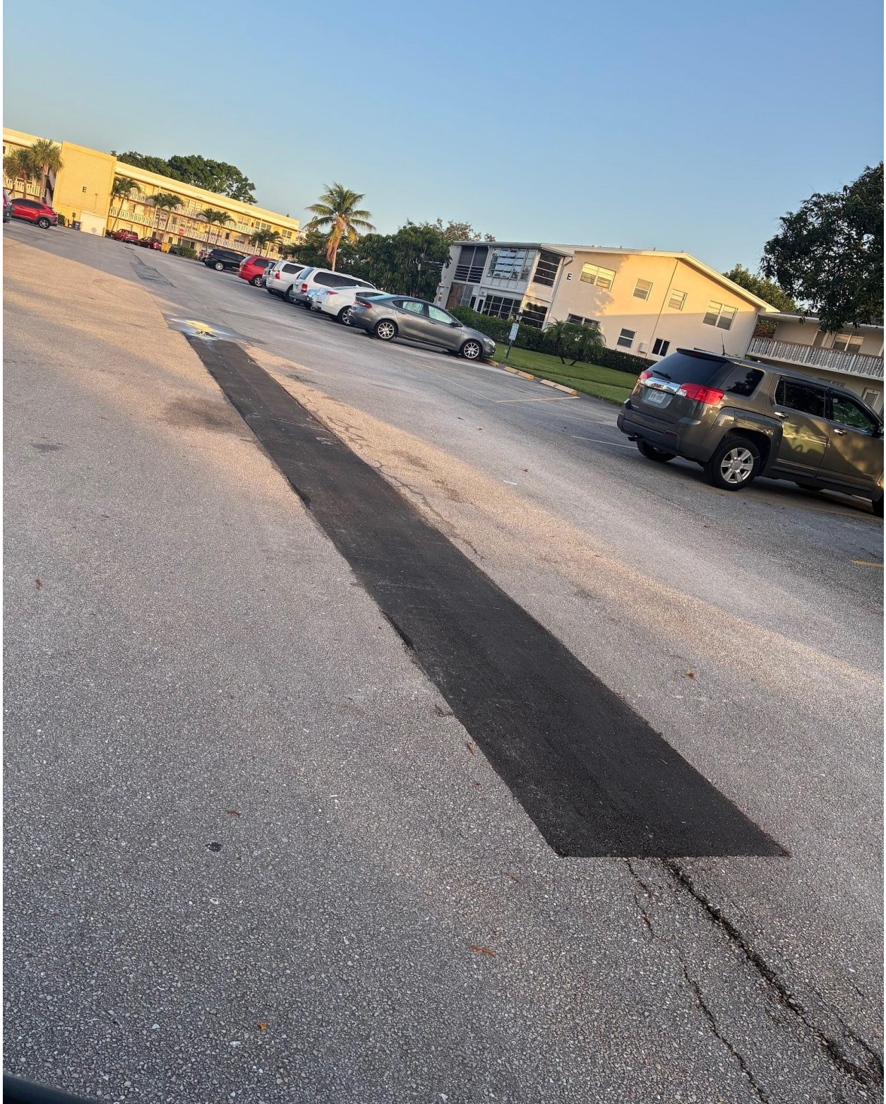
ANDOVER SECTION- ROAD REPAIR COMPLETE.
