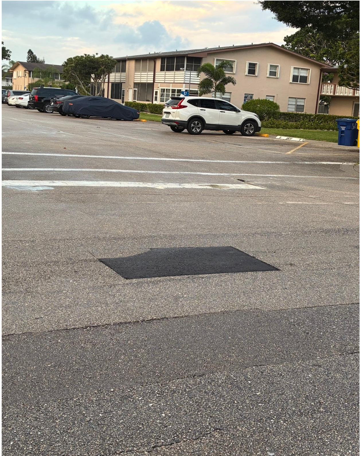
NORTH DRIVE- ROAD REPAIR COMPLETE.
