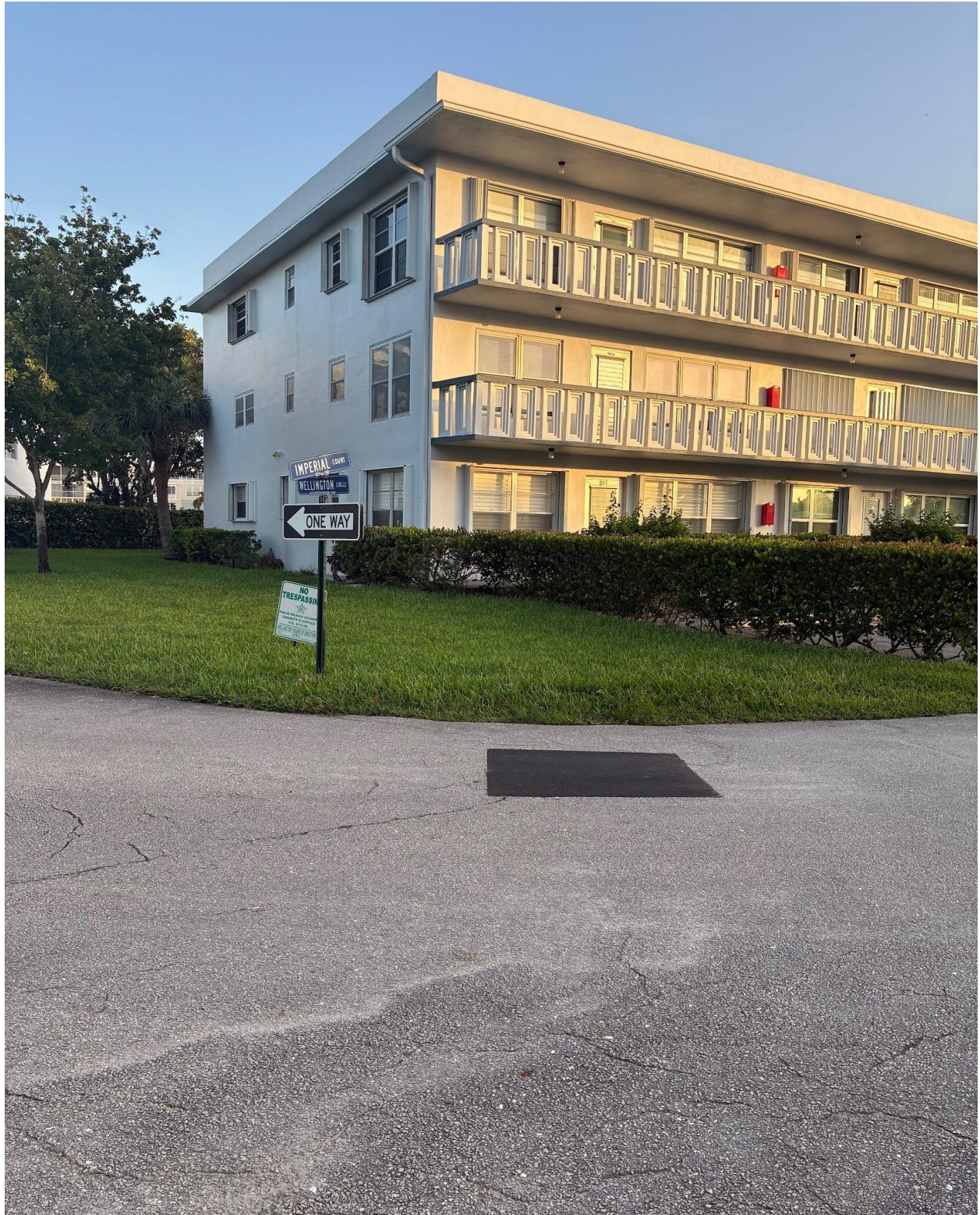
WELLINGTON SECTION- ROAD REPAIR COMPLETE.
