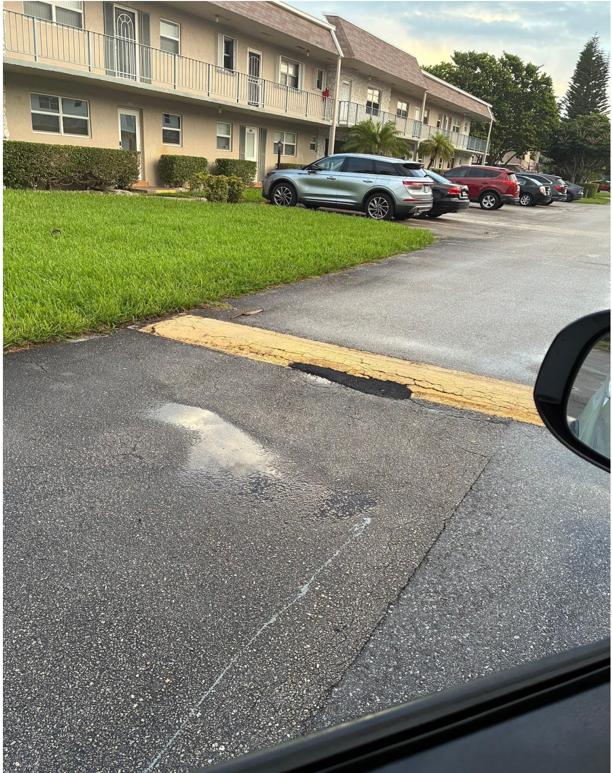
OXFORD SECTION- SPEED BUMP REPAIR COMPLETE.
