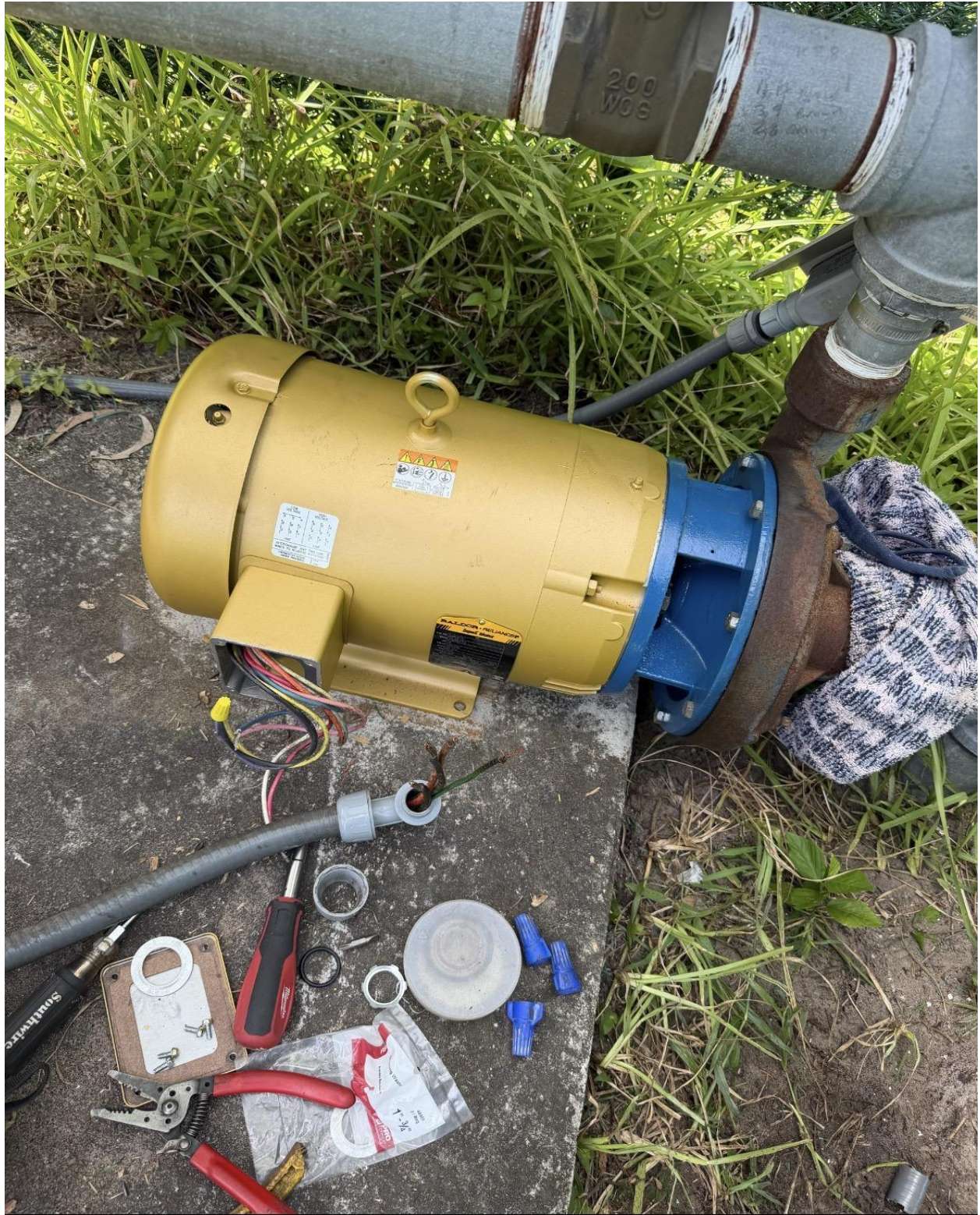
SOUTHAMPTON SECTION- THIS IRRIGATION PUMP AND PUMP MOTOR WAS REMOVED FOR SHOP SERVICE BY CHABOT IRRIGATION; REINSTALLED ON 7/17.
