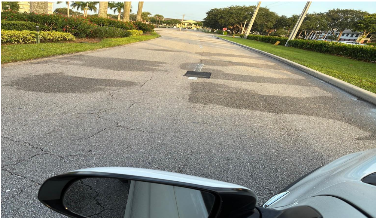
CENTURY BOULEVARD- ROAD REPAIRS COMPLETE.
