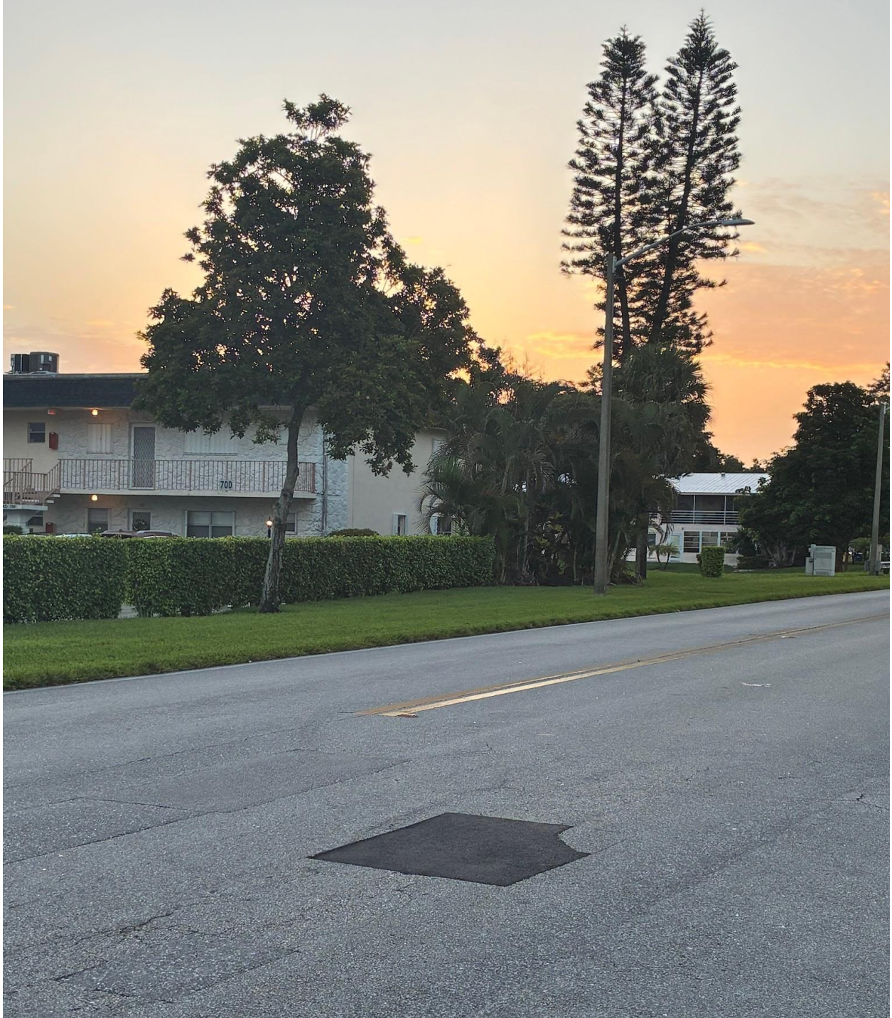
NORTH DRIVE- ROAD REPAIR COMPLETE.
