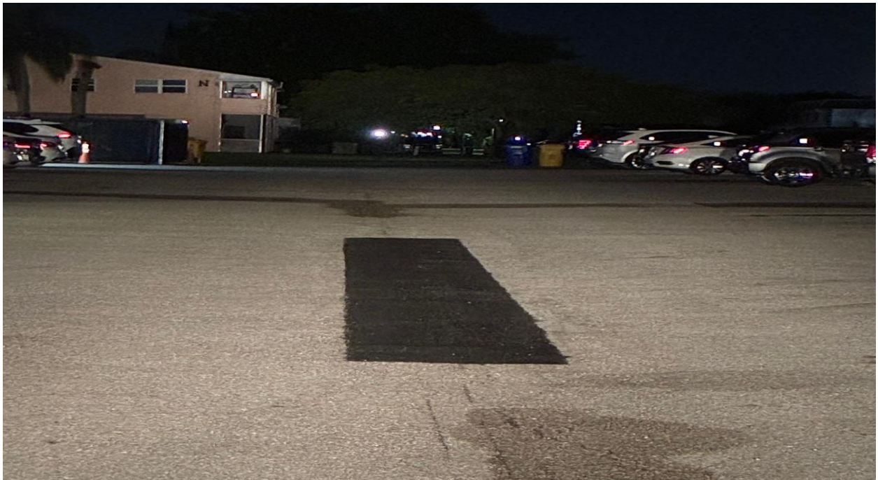
SHEFFIELD SECTION- ROAD REPAIR COMPLETE.
