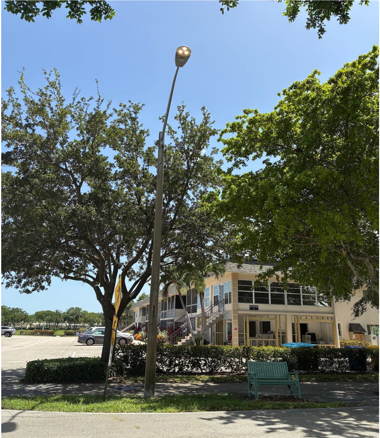
NORTH DRIVE, STRATFORD SECTION. DAYBURNER STREETLIGHT. REQUEST FOR REPAIR WAS SENT TO FPL, TICKET #46727.
