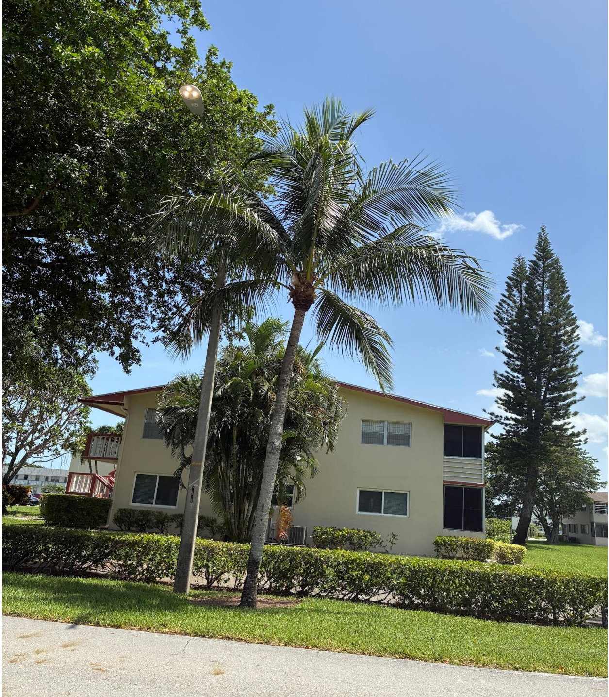
NORTH DRIVE- CHATHAM SECTION- DAYBURNER. A REQUEST WAS SENT TO FPL, TICKET #46726.
