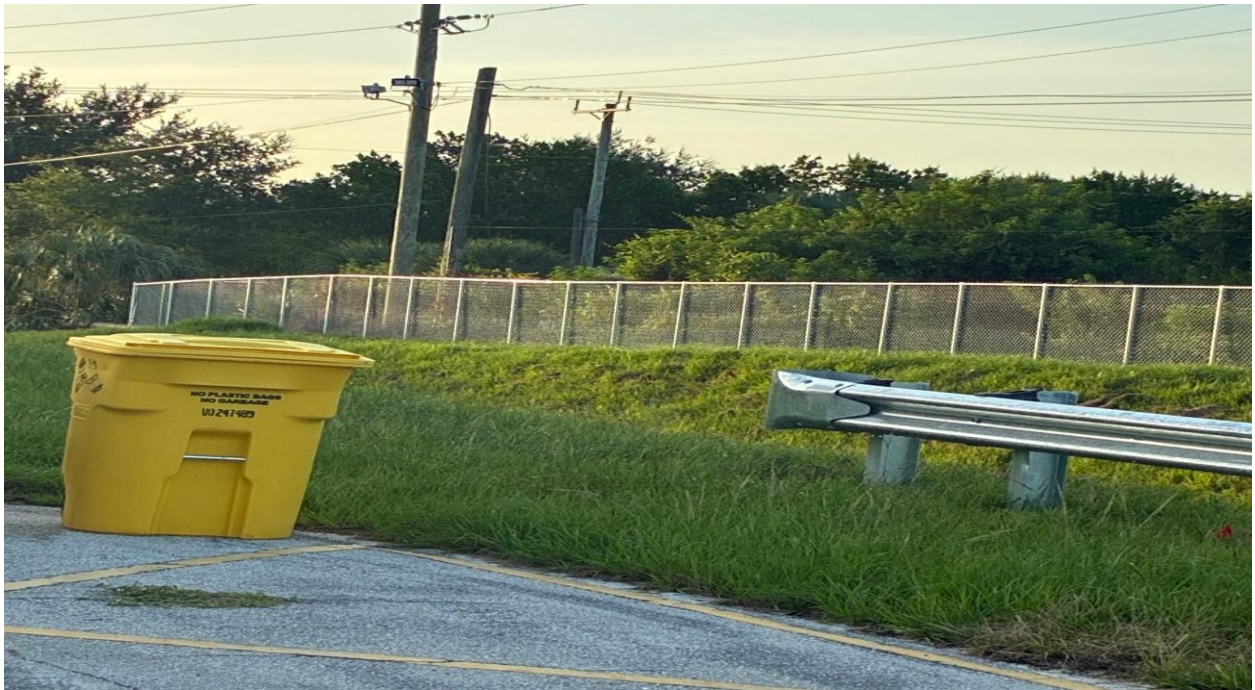
SOUTH CANAL- THE FINAL SECTION OF FENCE WAS INSTALLED BY BUDGET FENCE AND GATE ON 7/14.
