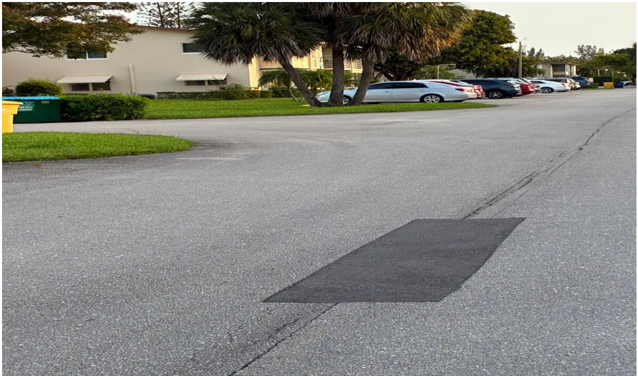
BEDFORD, EASTHAMPTON SECTIONS- ROAD REPAIRS COMPLETE,
