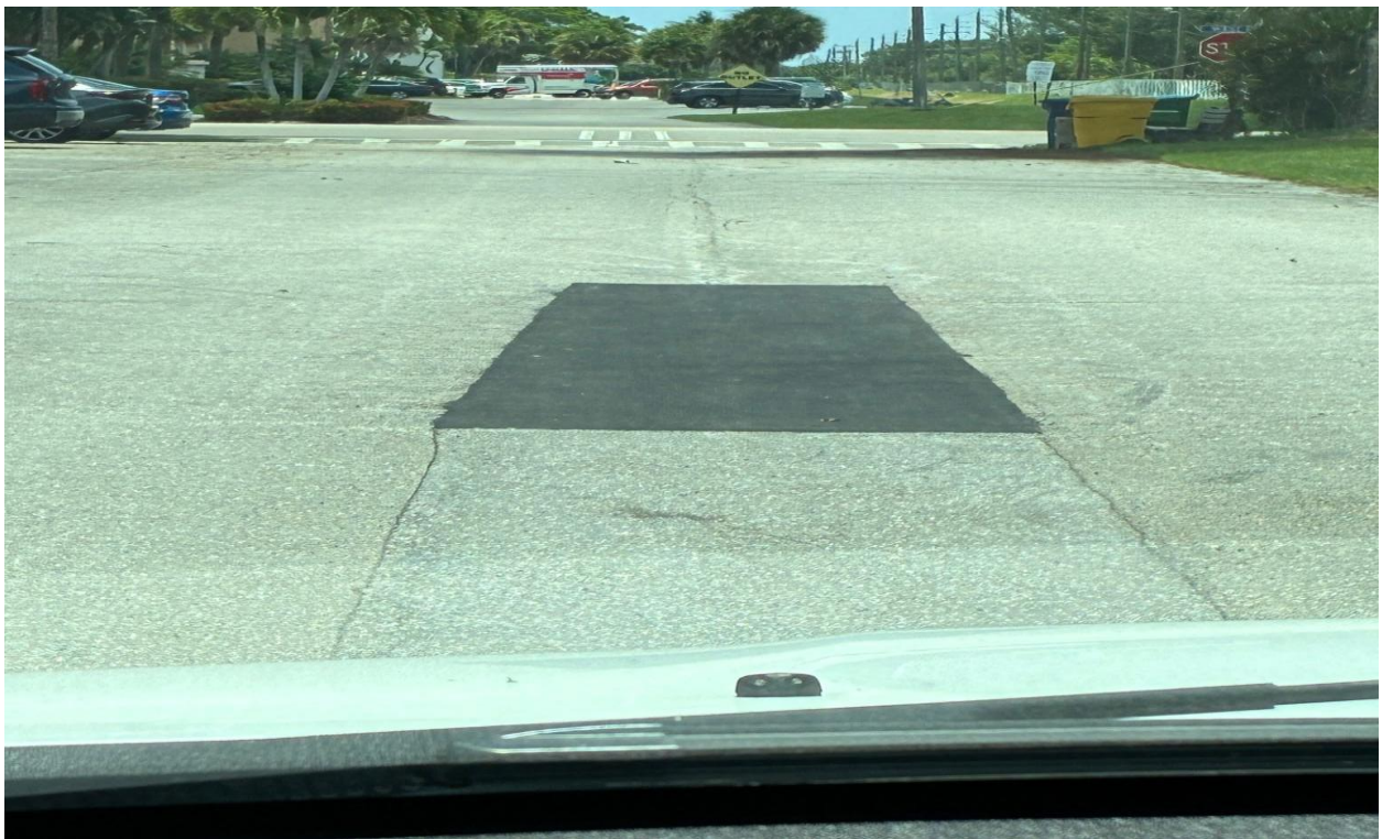
WINDSOR SECTION- REPAIR OF ROADWAY BY FEDERAL MAINTENANCE.
