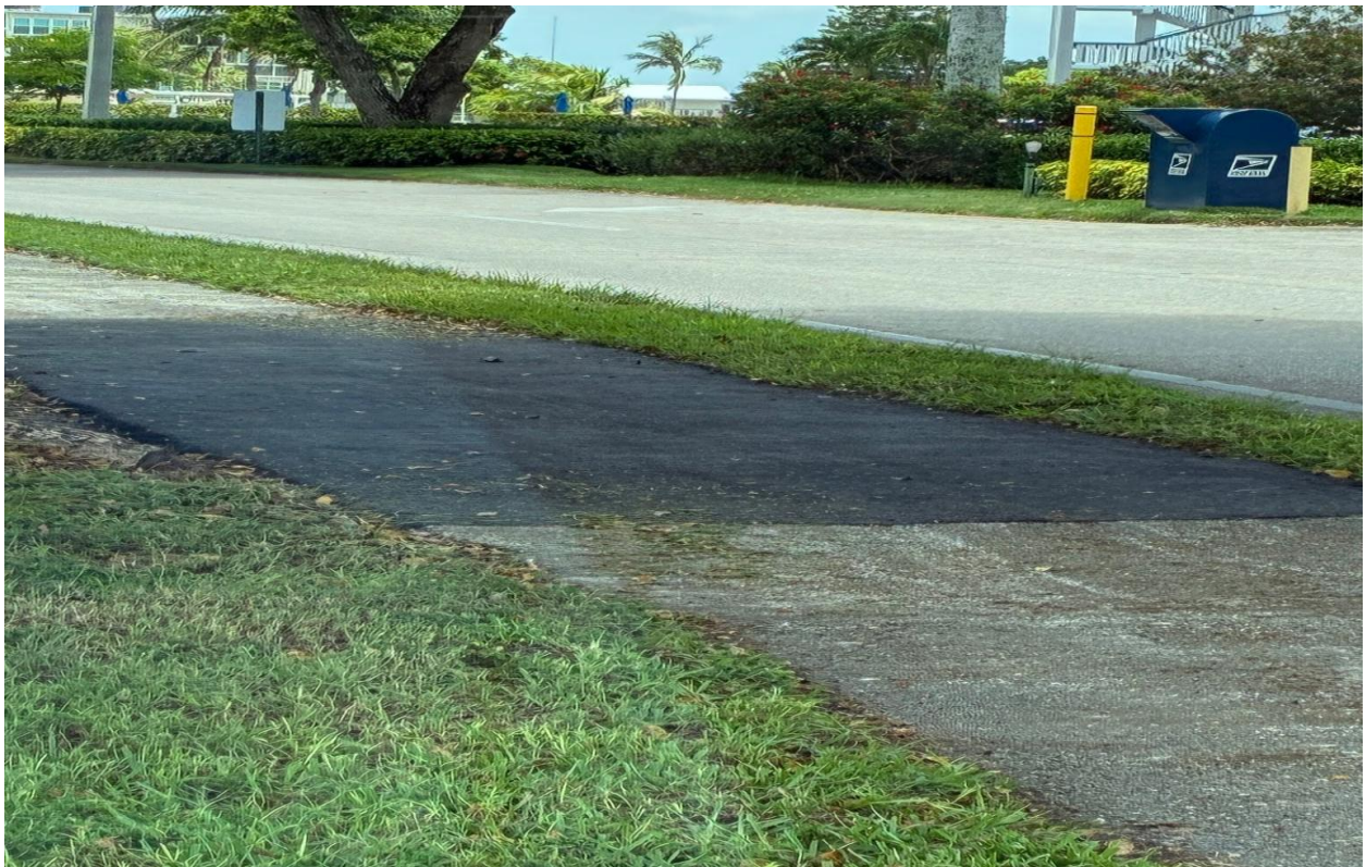
WEST DRIVE- REPAIR OF WALKWAY BY FEDERAL MAINTENANCE.
