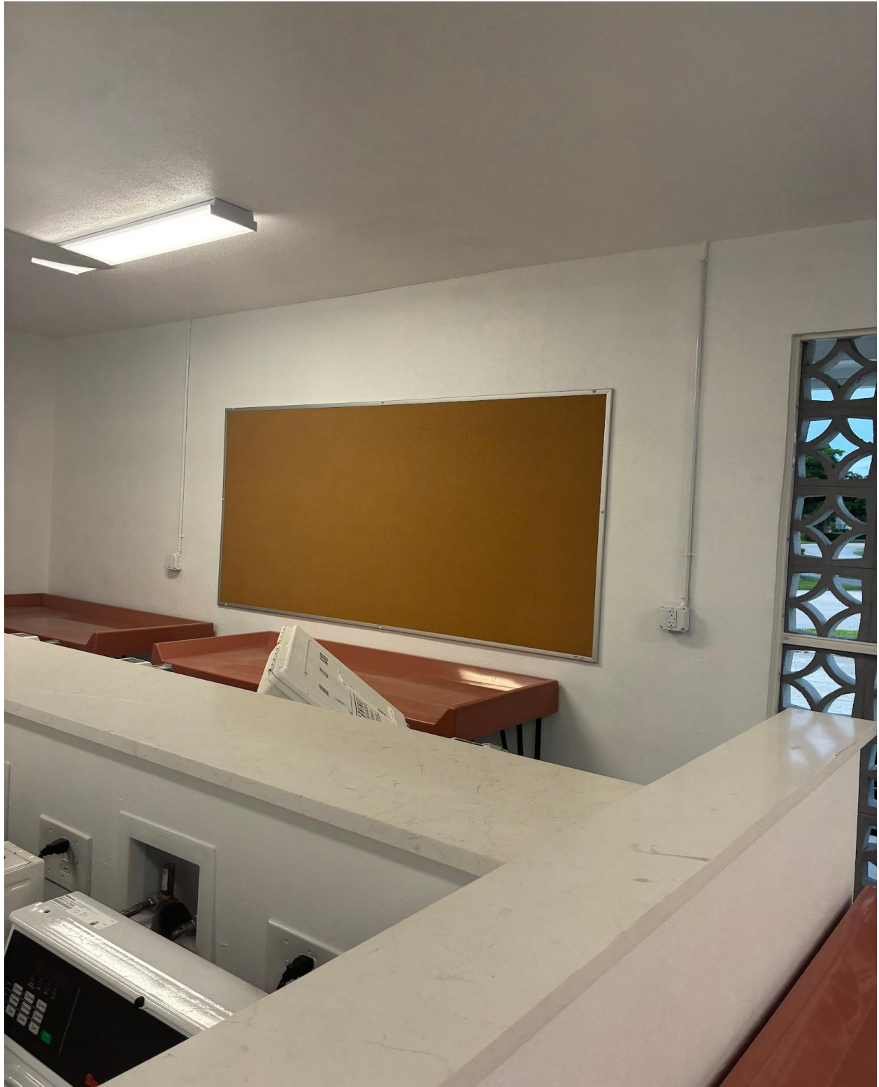
PLYMOUTH LAUNDRY- NEW BULLETIN BOARD INSTALLED BY DOS SANTOS CONSTRUCTION.
