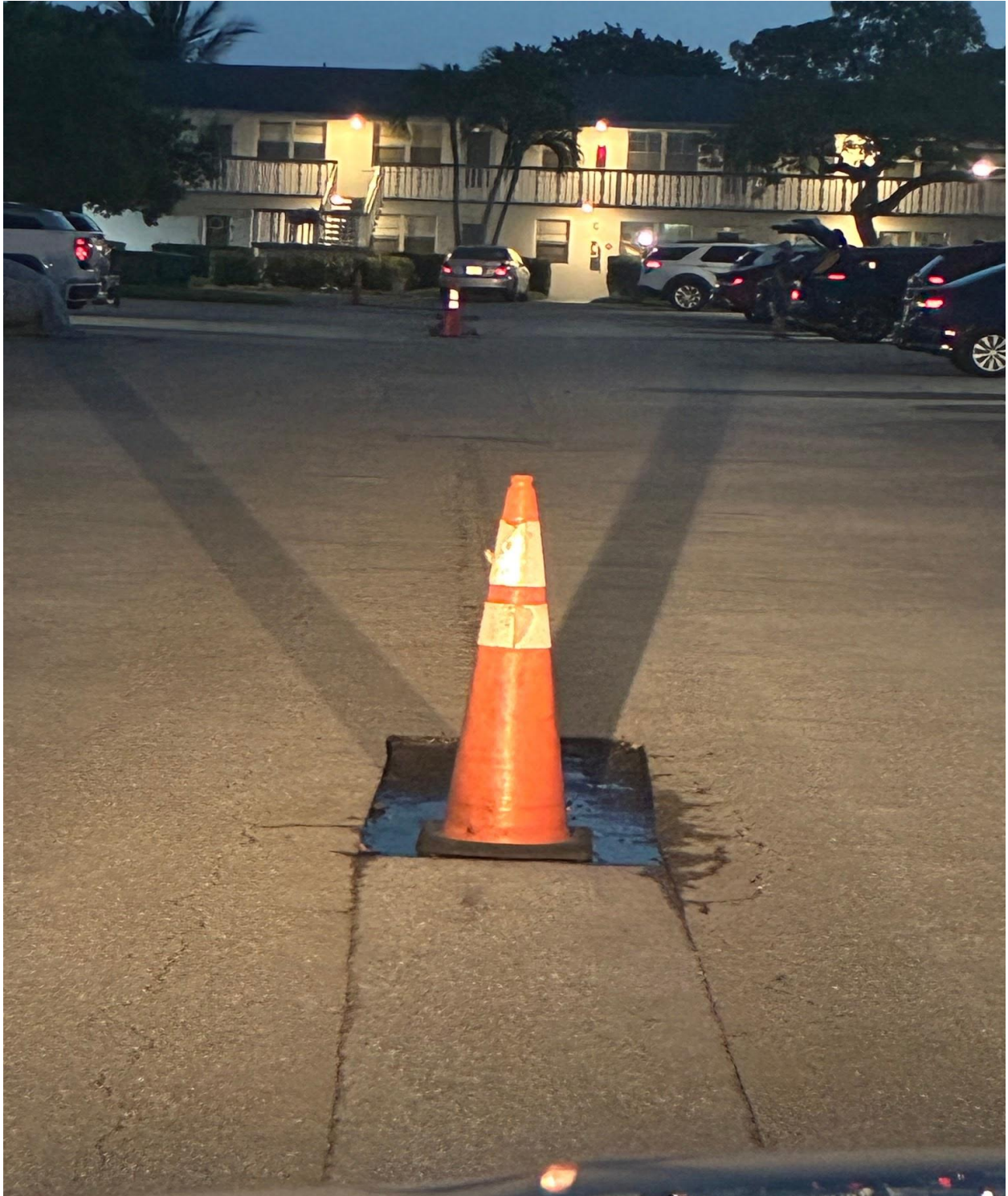
CAMDEN SECTION- REPAIR OF ROADWAY BY FEDERAL MAINTENANCE.
