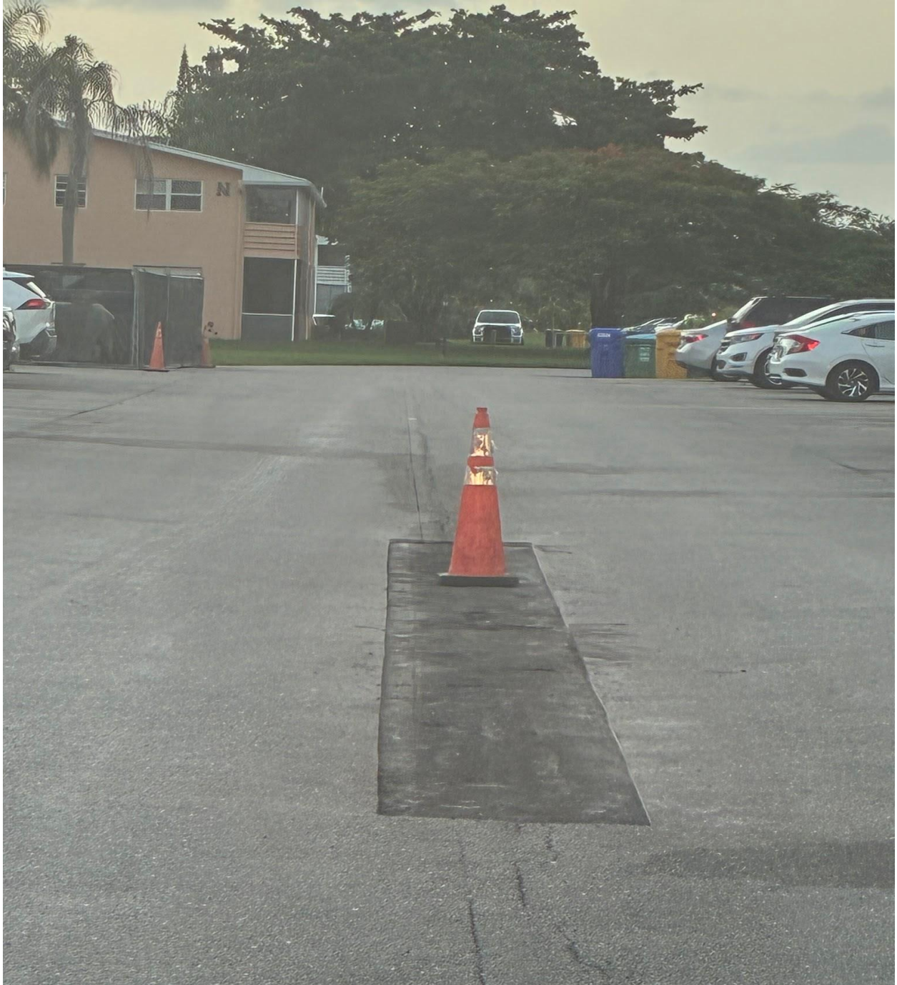
SHEFFIELD SECTION- REPAIR OF ROADWAY BY FEDERAL MAINTENANCE.
