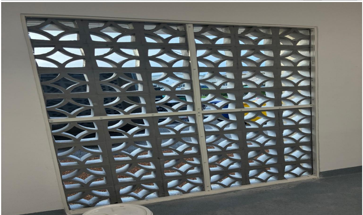
PLYMOUTH LAUNDRY- THESE NEW SCREENS WILL KEEP OUT BUGS AND RAIN, BUT STILL ALLOW FOR AIR CIRCULATION.
