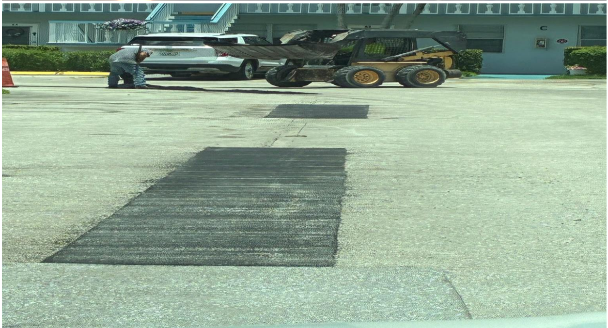
BERKSHIRE SECTION- REPAIR OF ROADWAY BY FEDERAL MAINTENANCE.
