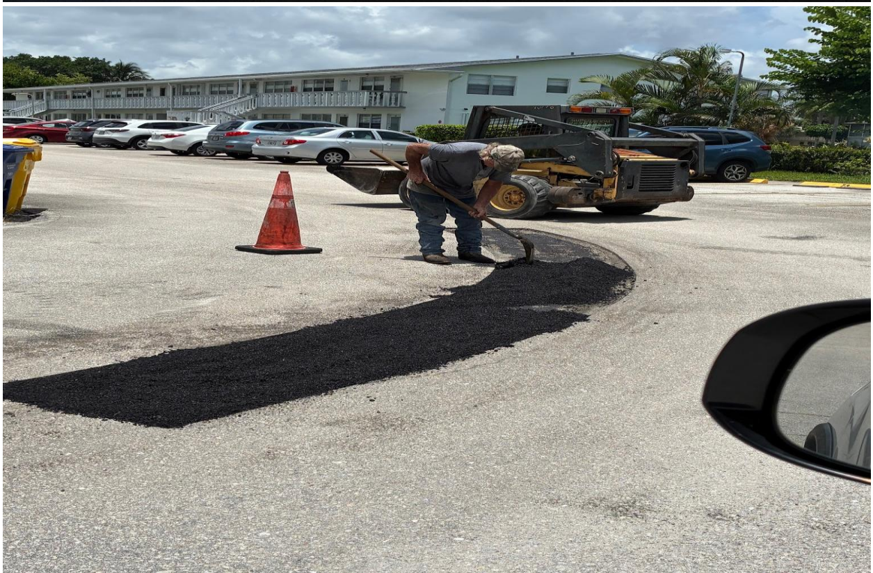
BERKSHIRE SECTION- REPAIR OF ROADWAY BY FEDERAL MAINTENANCE.
