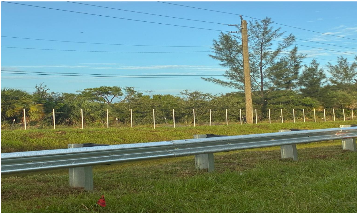
SOUTH CANAL- BUDGET FENCE AND GATE SYSTEMS CONTINUES WITH INSTALLATION OF NEW FENCES ALONG THE SOUTH SIDE OF SOUTH CANAL.
