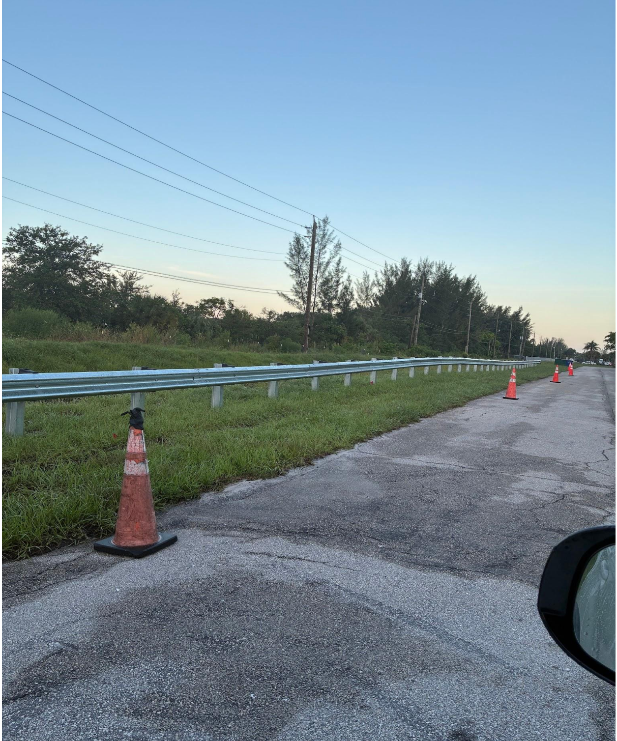
ANDOVER SECTION- ANOTHER SECTION OF GUARDRAIL WAS INSTALLED ALONG SOUTH CANAL ON 7/6.
