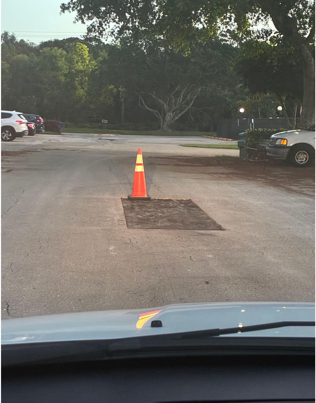
DORCHESTER SECTION- REPAIR OF ROADWAY BY FEDERAL MAINTENANCE.
