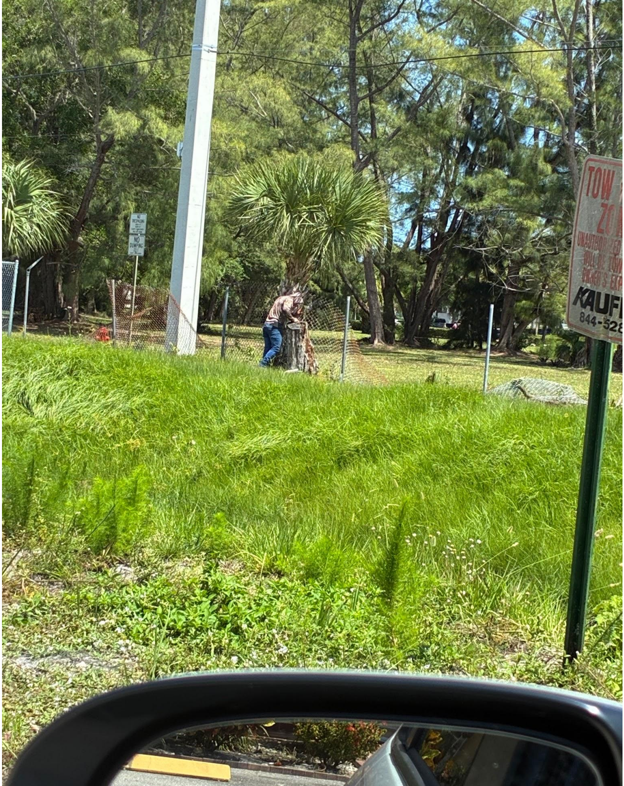
SOUTH CANAL- FENCE INSTALLATION WORK CONTINUES.
