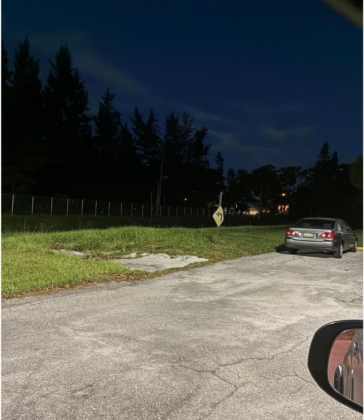
SOUTH CANAL- DARK FLOODLIGHT NEAR WINDSOR A. REPORTED TO FPL, TICKET #45960.
