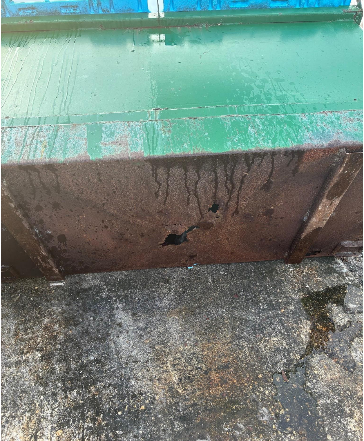
SOMERSET L- RUSTED OUT DUMPSTER. A REQUEST FOR REPLACEMENT WAS SENT TO WASTE PRO.
