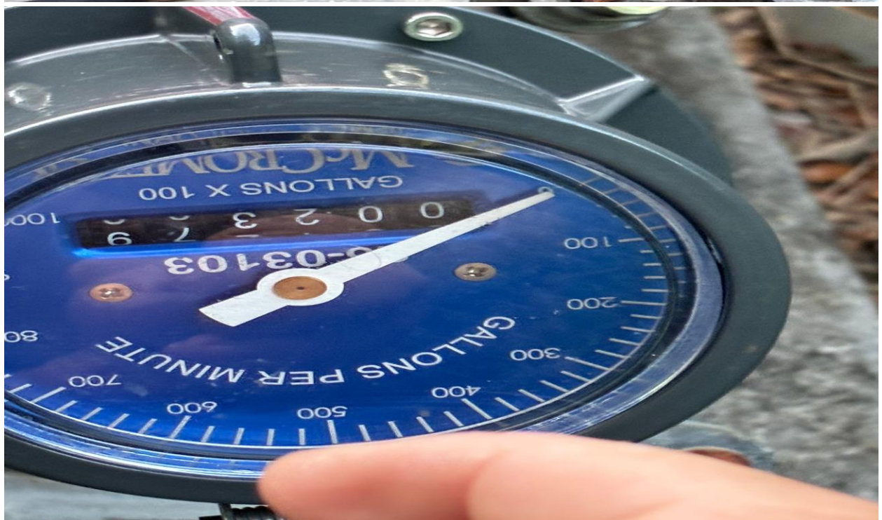
NORTH DRIVE- NEW IRRIGATION FLOWMETER INSTALLED BY CHABOT IRRIGATION.
