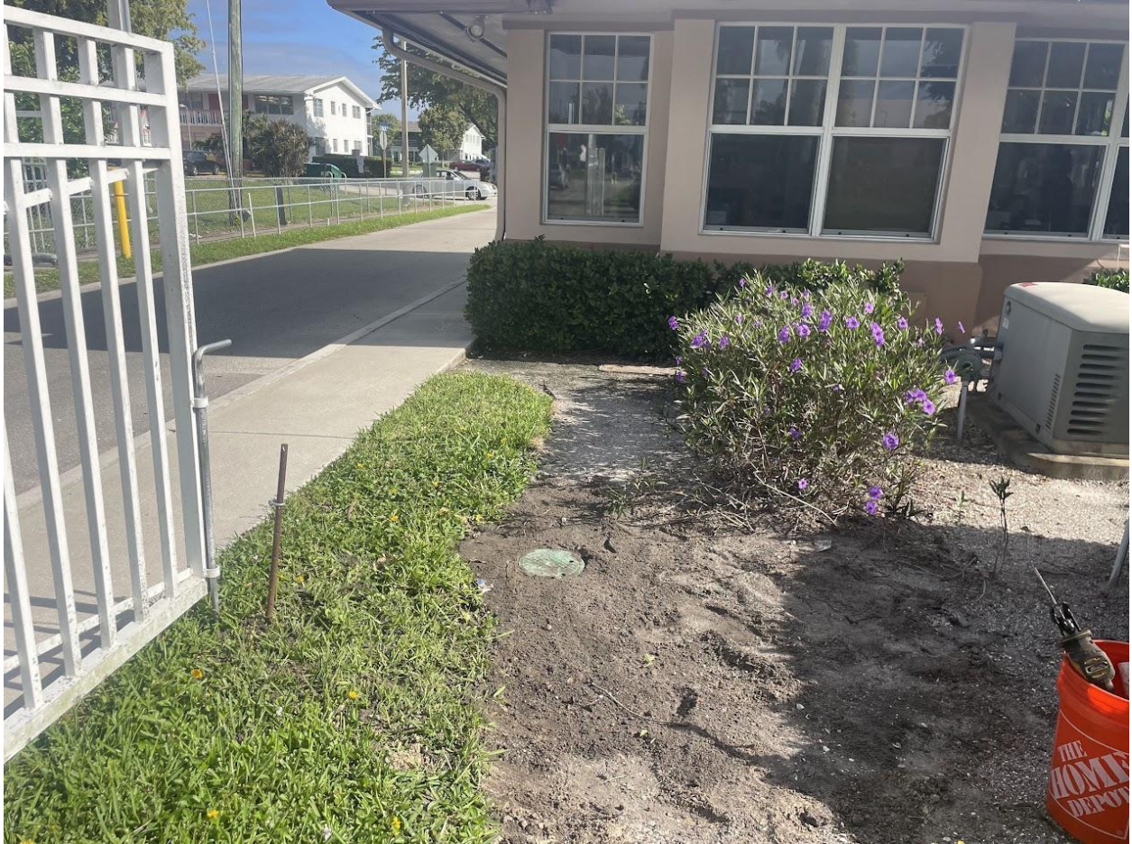
OKEECHOBEE GUARDHOUSE- IRRIGATION REPAIRS MADE BY SEACREST SERVICES LAST WEEK.
