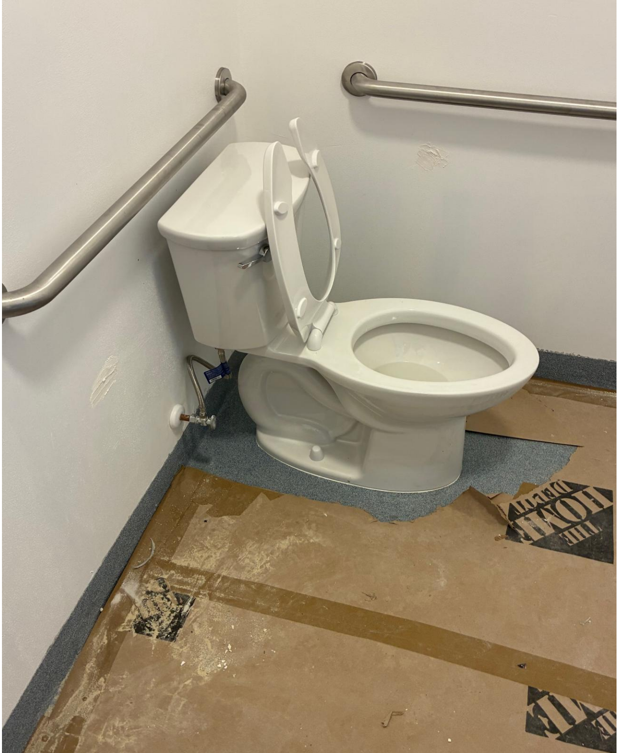
PLYMOUTH LAUNDRY- HANDRAILS INSTALLED. THIS IS AN ADA COMPLIANT RESTROOM.
