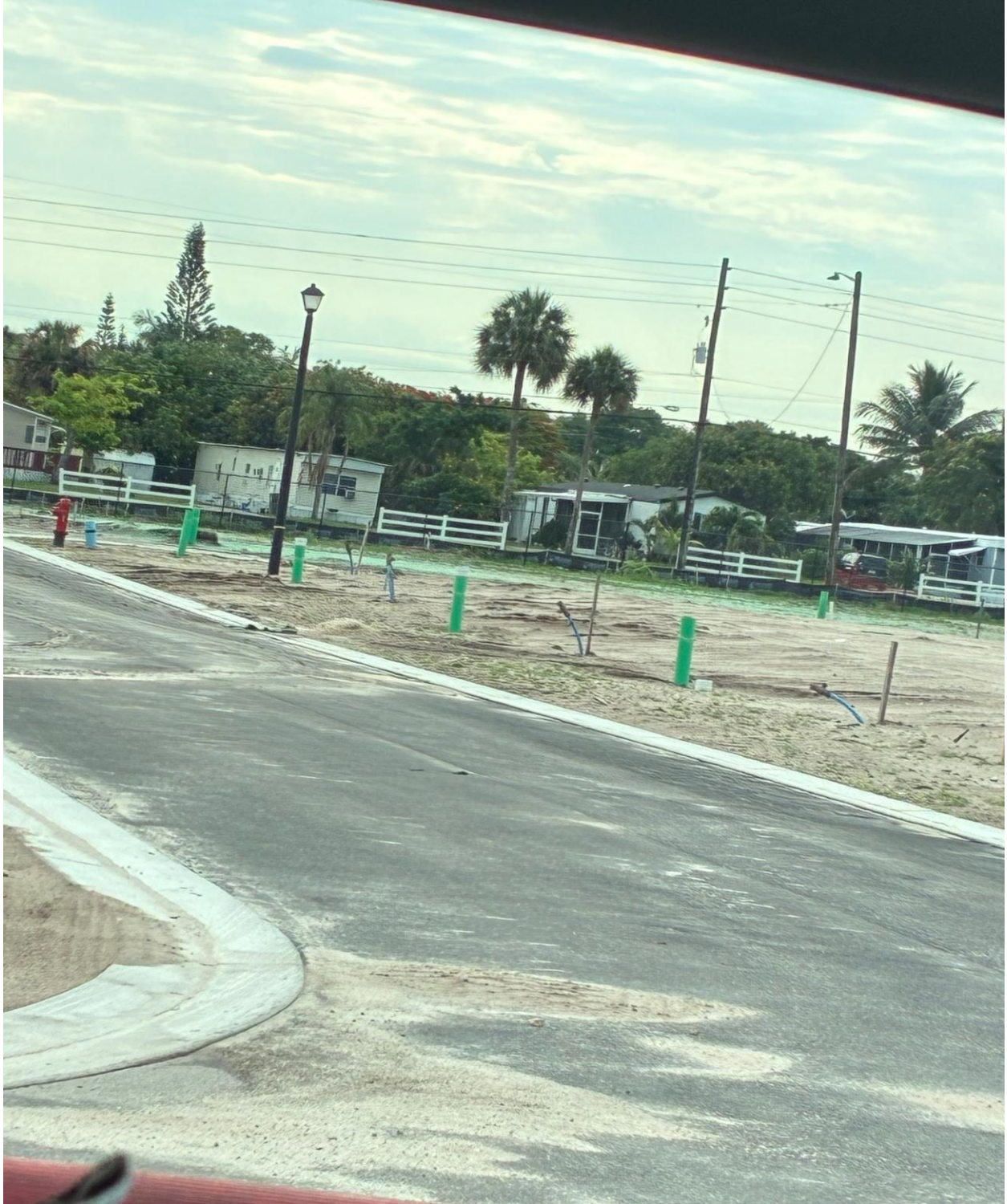
REFLECTION BAY- NEW ROADS, CURBS, ELECTRIC AND WATER SERVICES, FIRE HYDRANTS.
