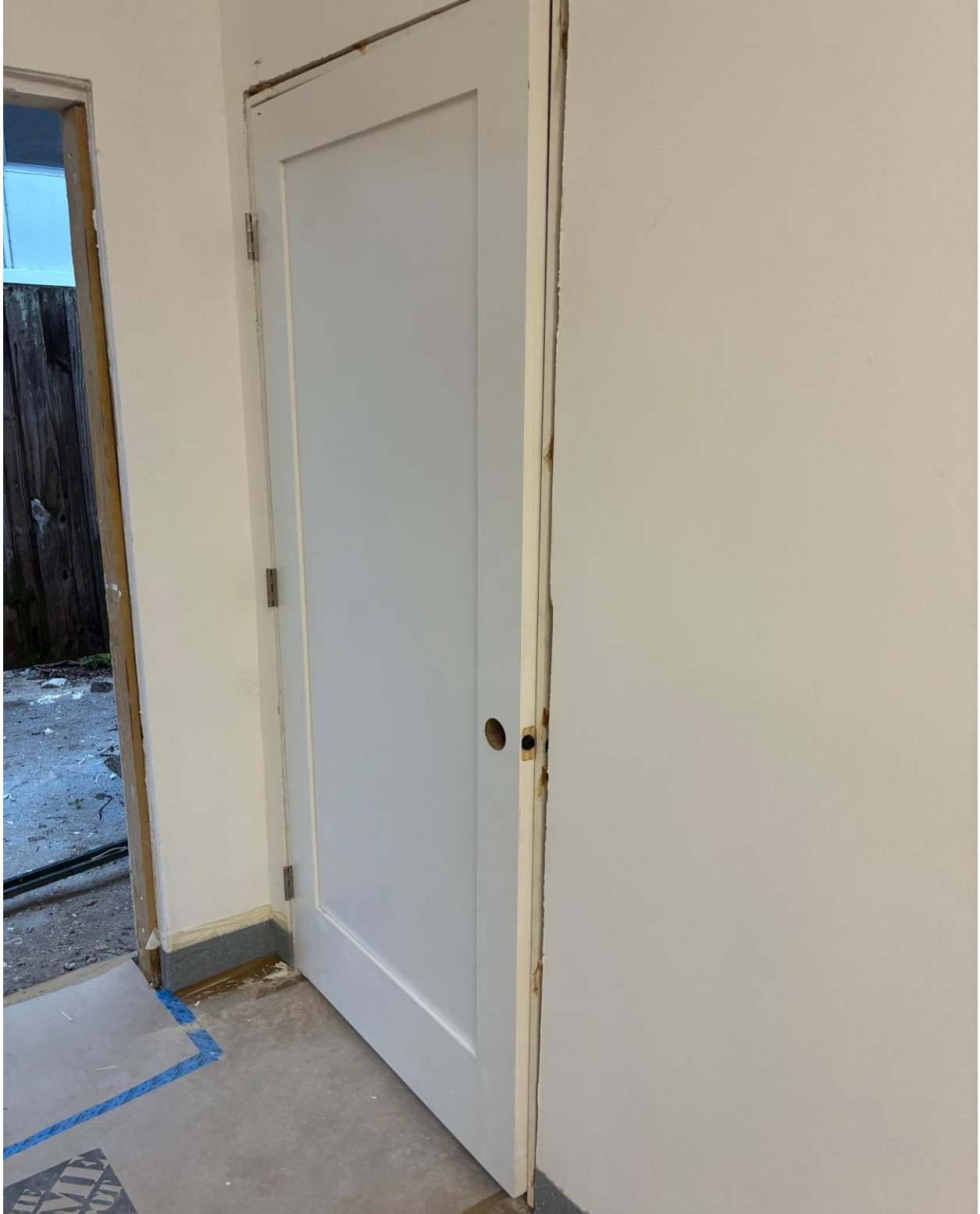
PLYMOUTH LAUNDRY- NEW ENTRY DOOR FOR OUR ADA COMPLIANT REST ROOM.
