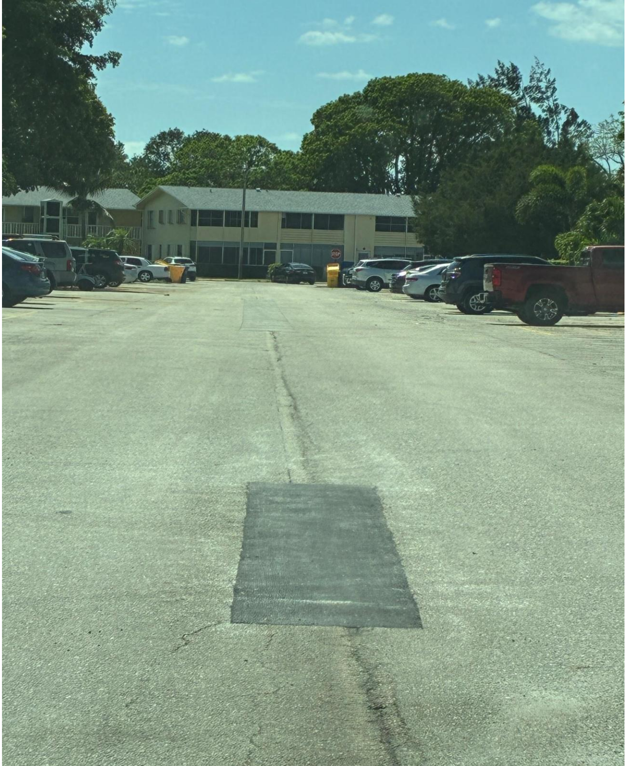
WINDSOR/CAMDEN SECTION- ASPHALT REPAIR COMPLETE.
