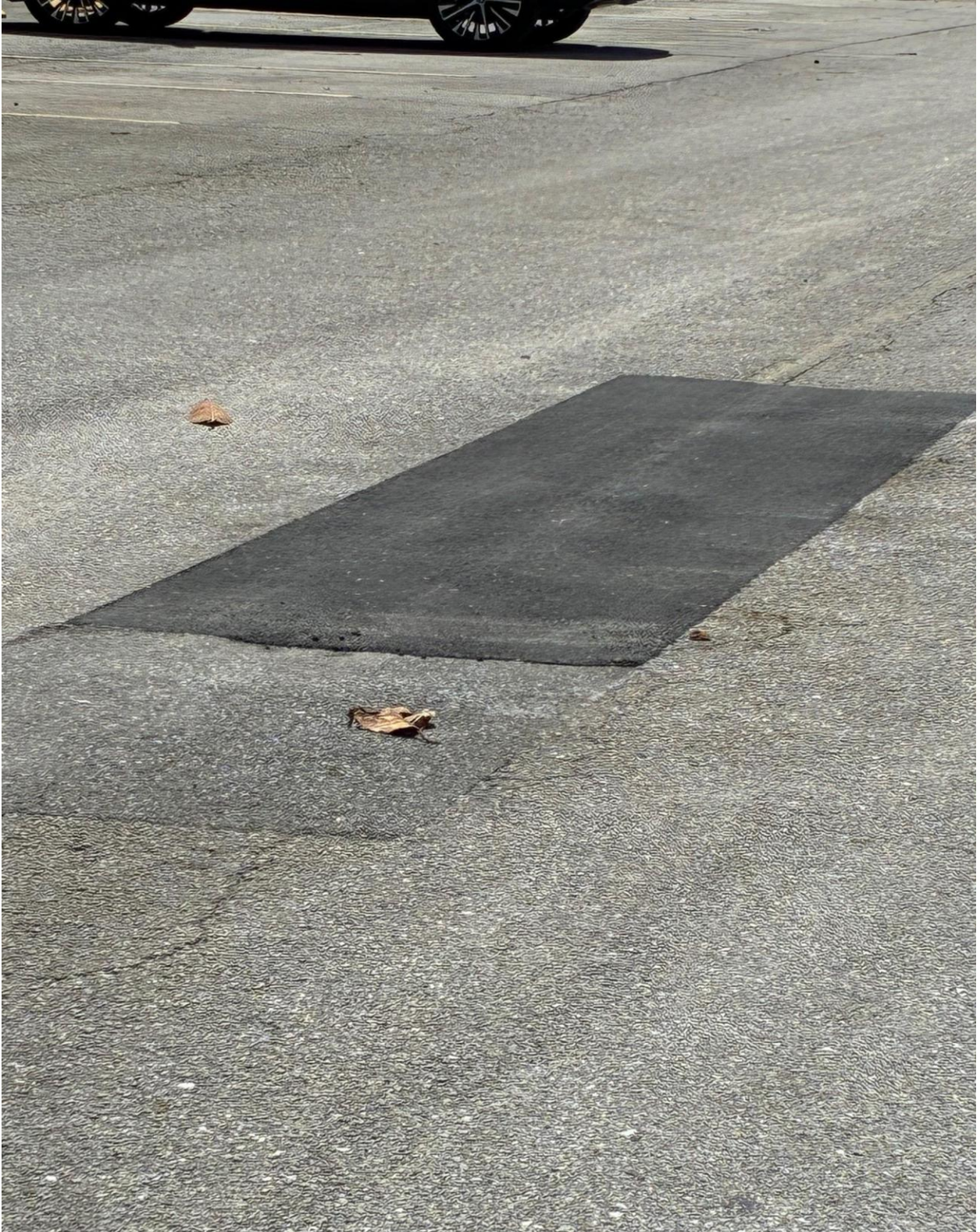
WINDSOR/CAMDEN SECTION- ASPHALT REPAIR COMPLETE.
