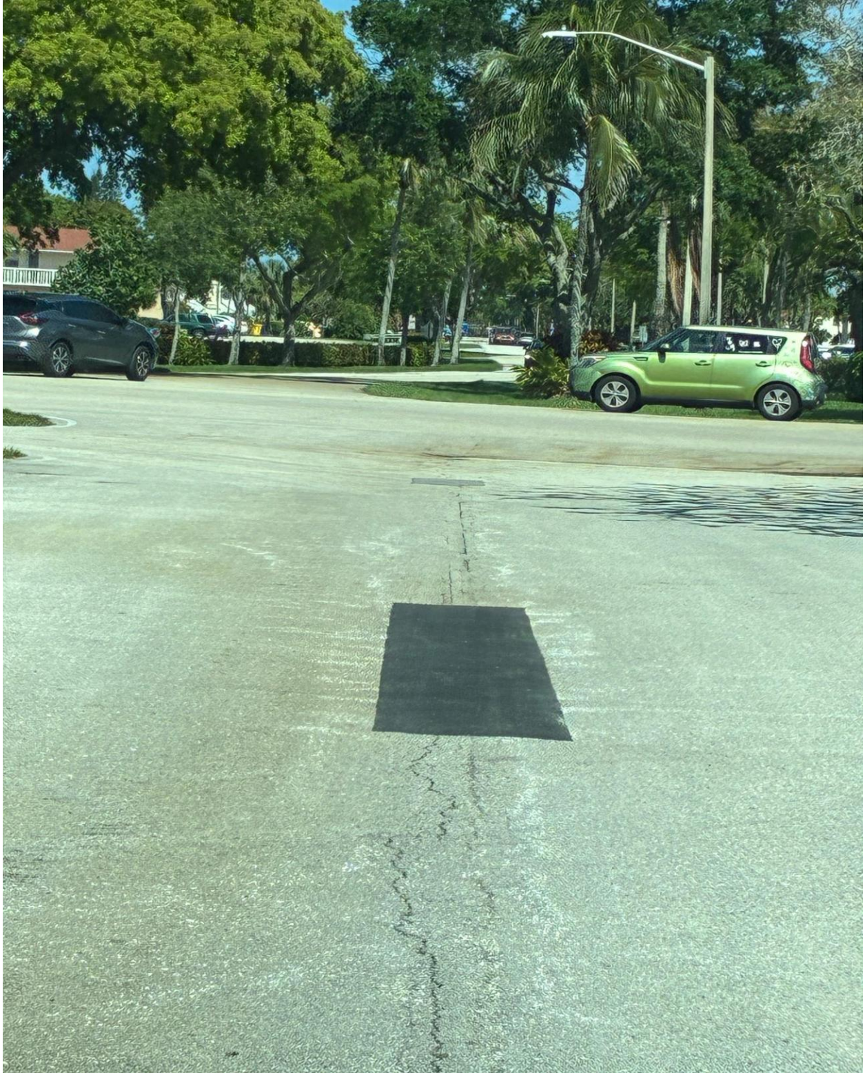
WINDSOR/CAMDEN SECTION- ASPHALT REPAIR COMPLETE.
