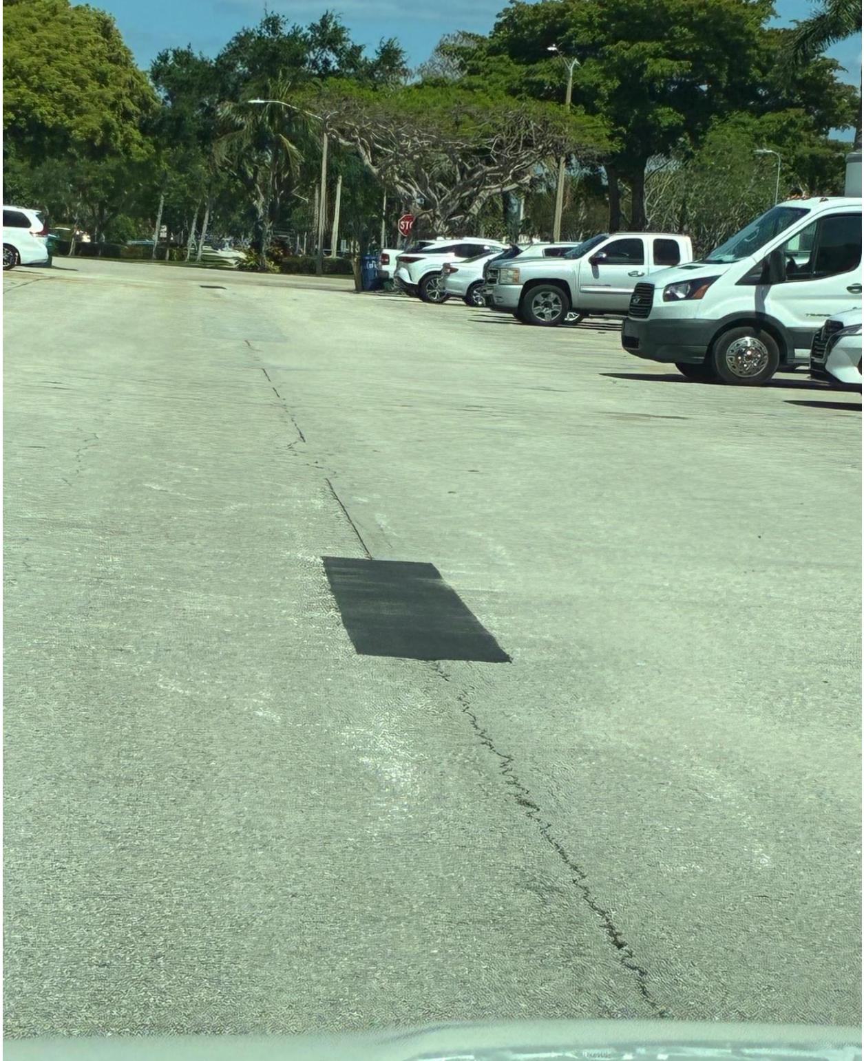
WINDSOR/CAMDEN SECTION- ASPHALT REPAIR COMPLETE.
