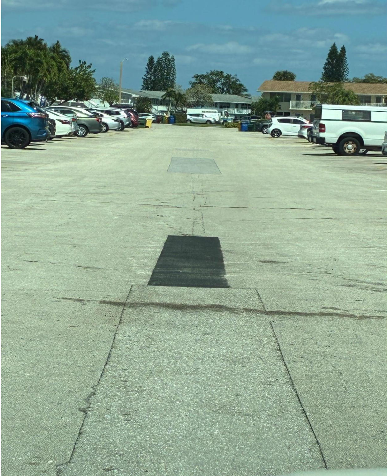
WINDSOR/CAMDEN SECTION- ASPHALT REPAIR COMPLETE.
