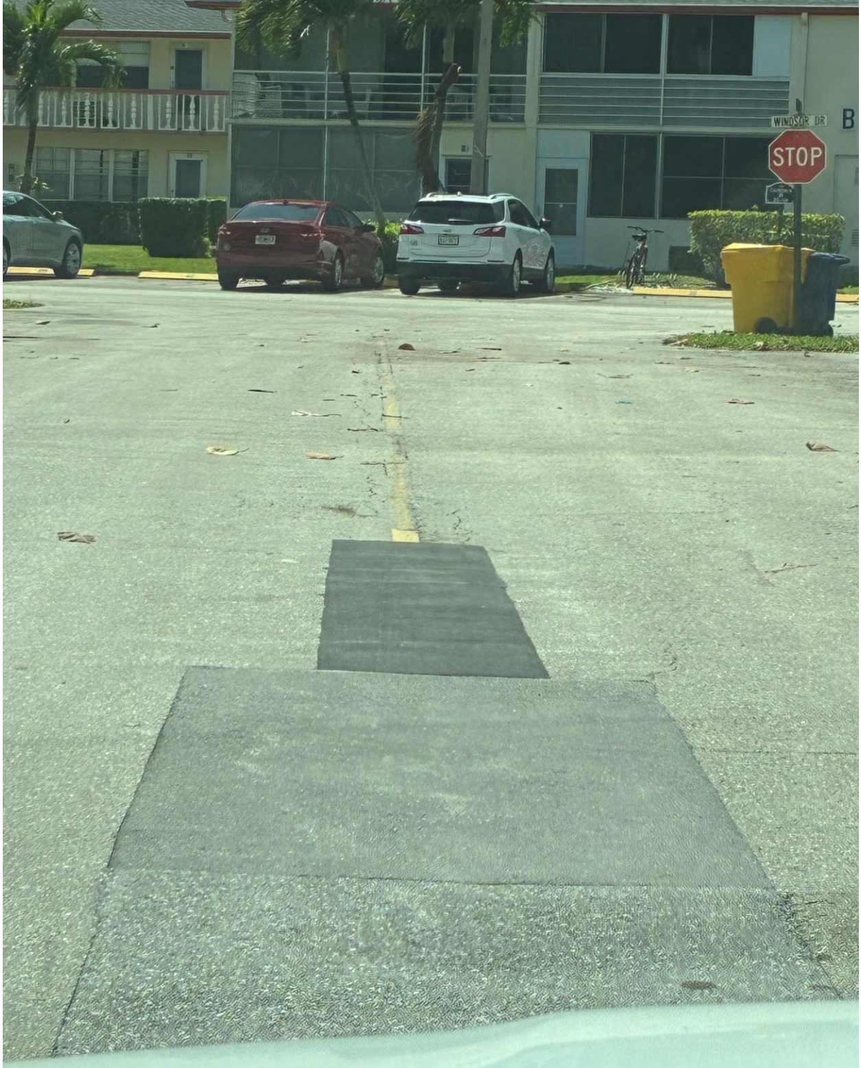
WINDSOR/CAMDEN SECTION- ASPHALT REPAIR COMPLETE.
