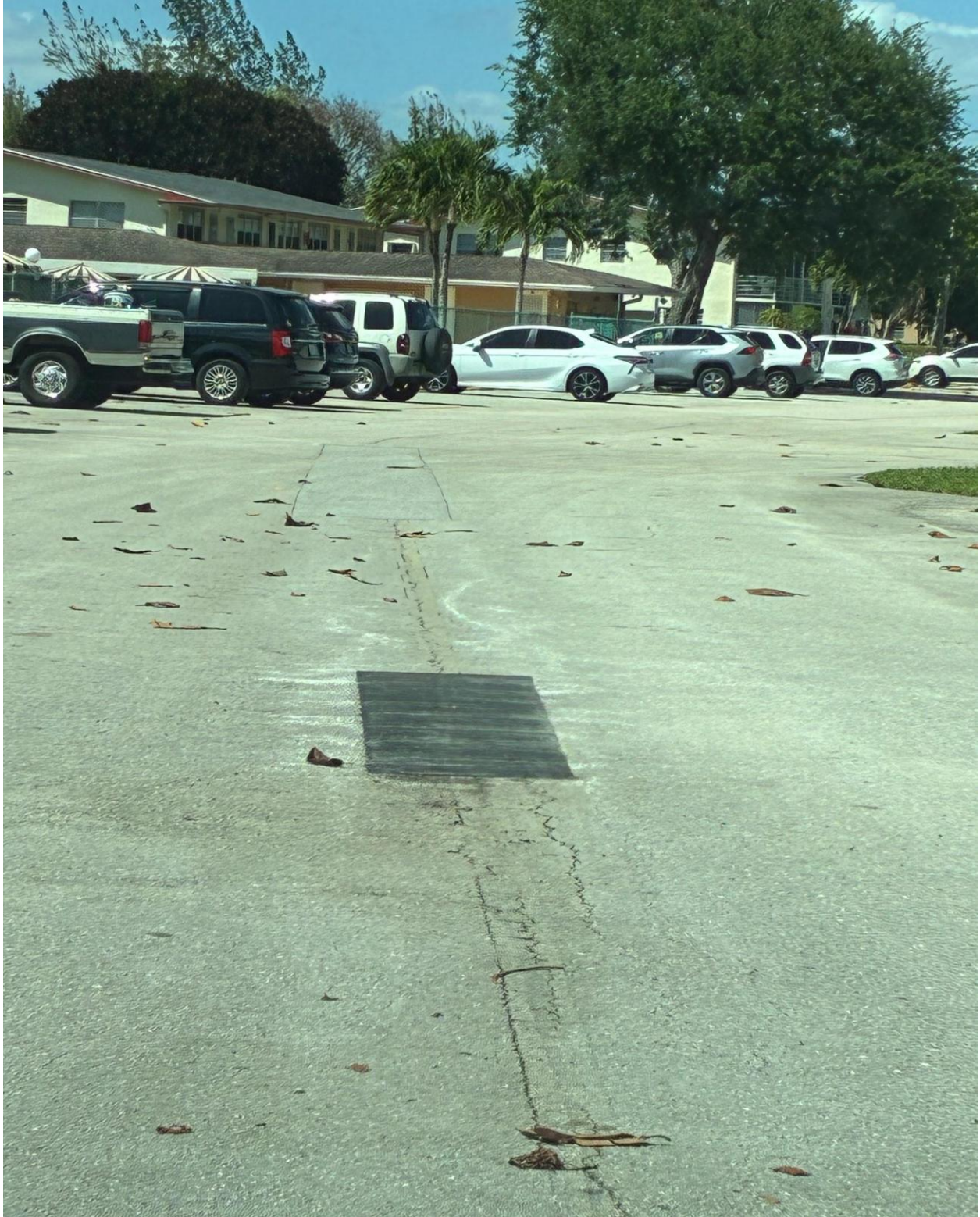
WINDSOR/CAMDEN SECTION- ASPHALT REPAIR COMPLETE.
