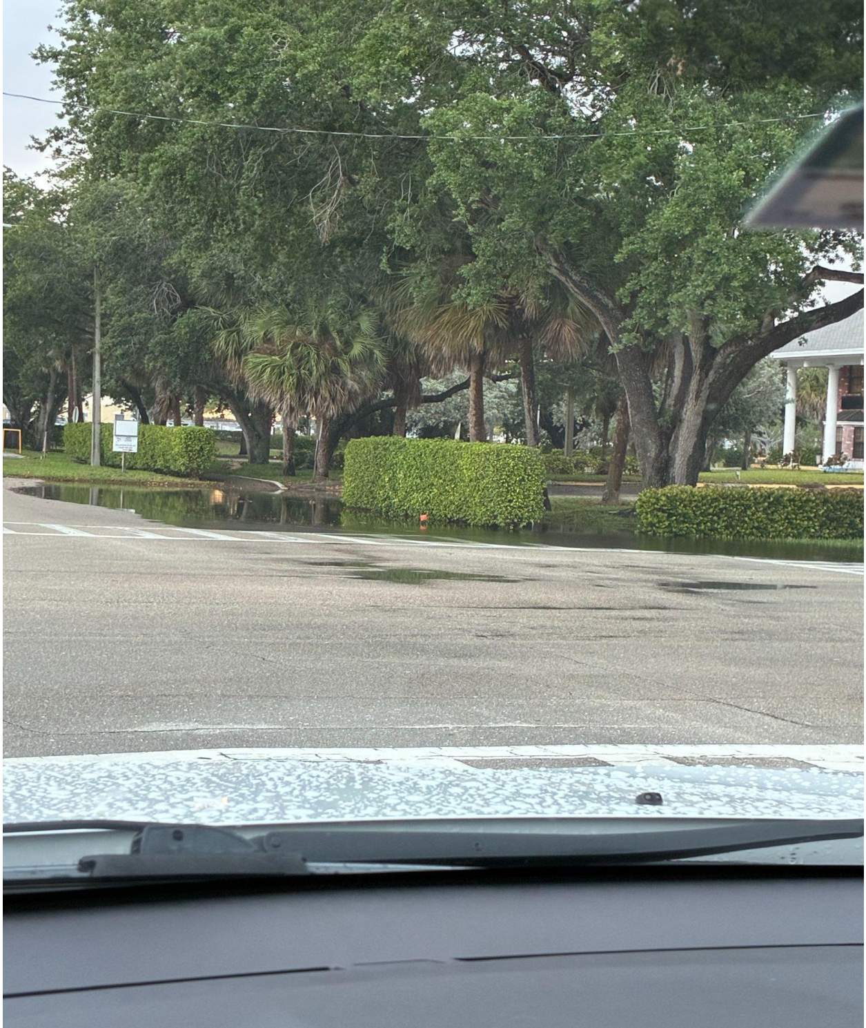
CV MEDICAL BUILDING- THIS CORNER WAS FLOODING AFTER HEAVY RAINS.
