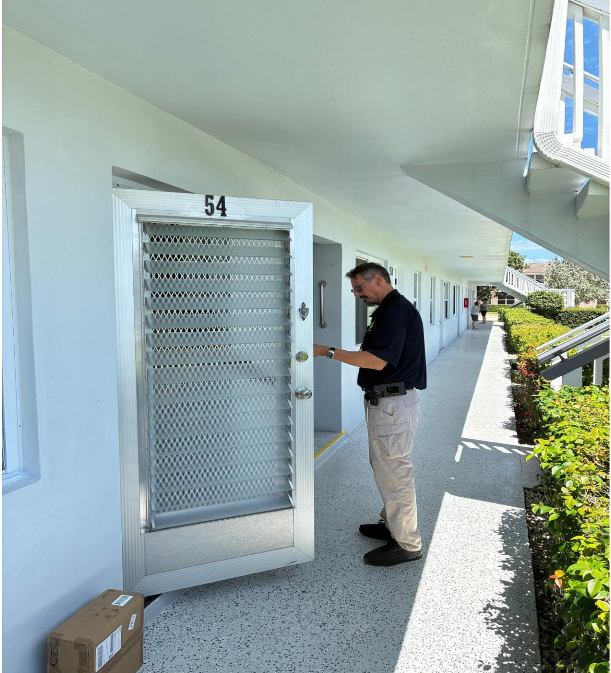
54 KENT D- A CODE COMPLIANCE OFFICER INSPECTED THIS UNIT ON 5/21. A NOTICE OF VIOLATION WAS ISSUED, WITH A 45 DAY DEADLINE FOR COMPLIANCE.
