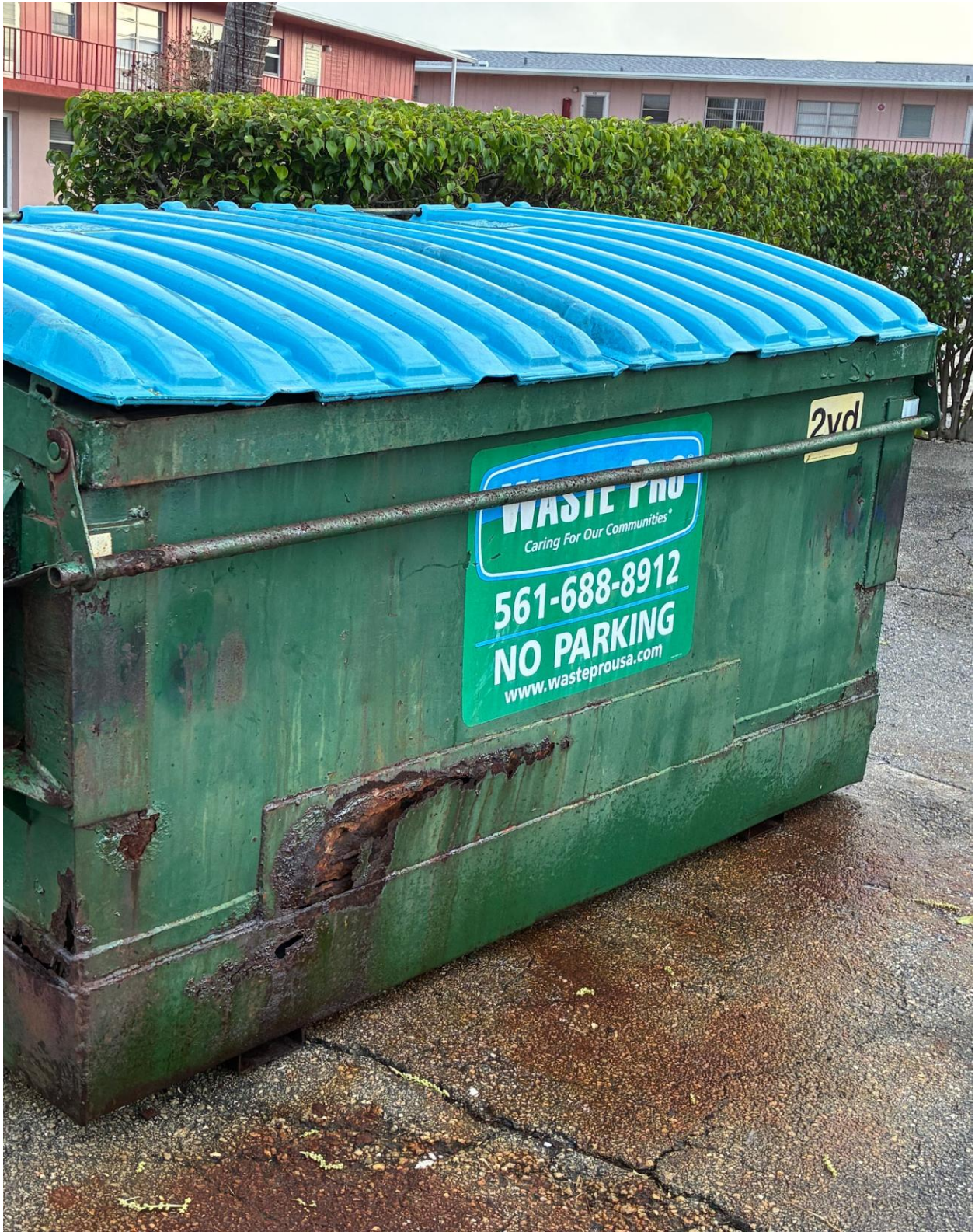
GOLFS EDGE BUILDING 6- RUSTED OUT DUMPSTER. A REQUEST FOR REPLACEMENT WAS SENT TO WASTE PRO.
