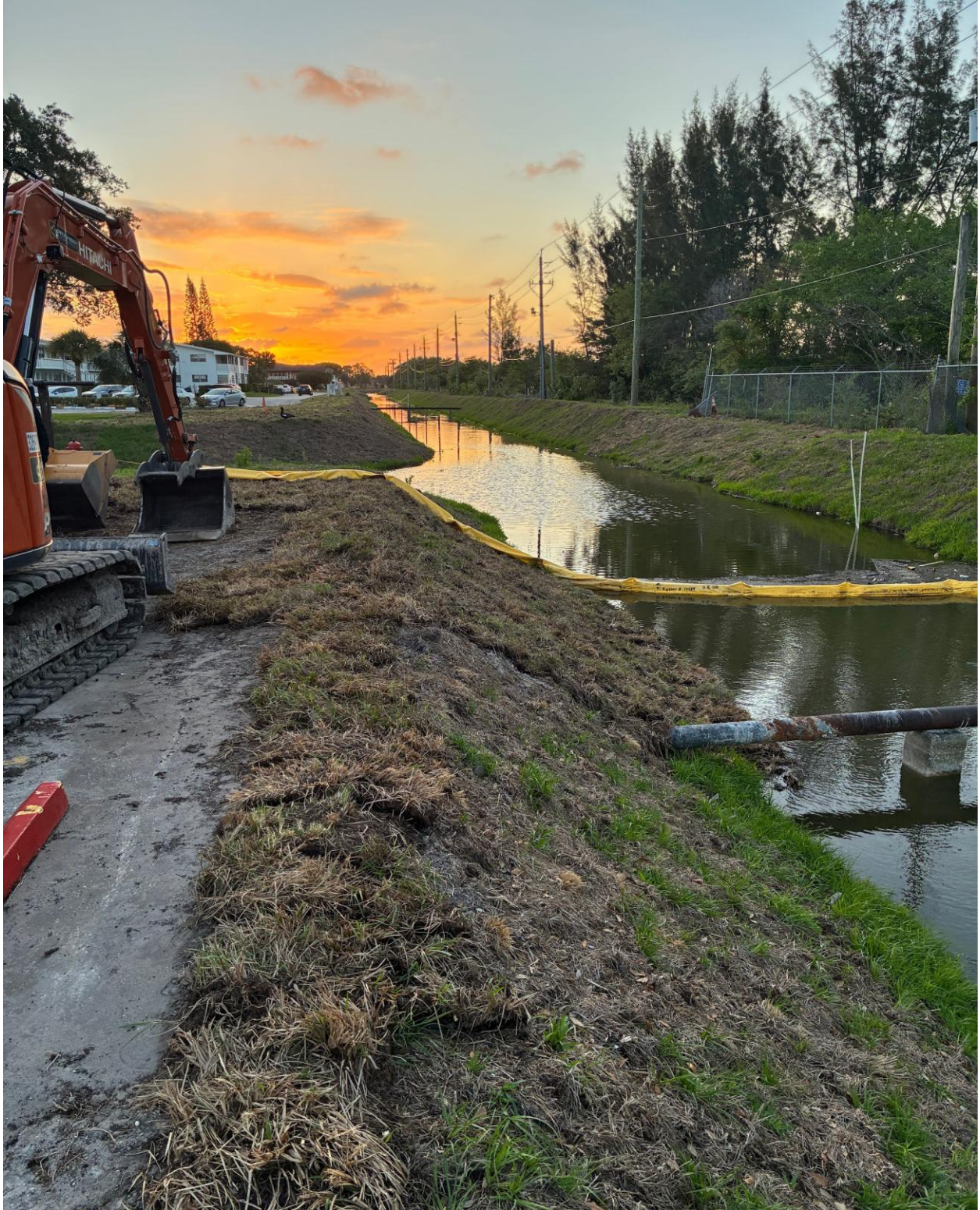
SOUTH CANAL- SOD INSTALLATION AT THIS SECTION IS COMPLETE.
