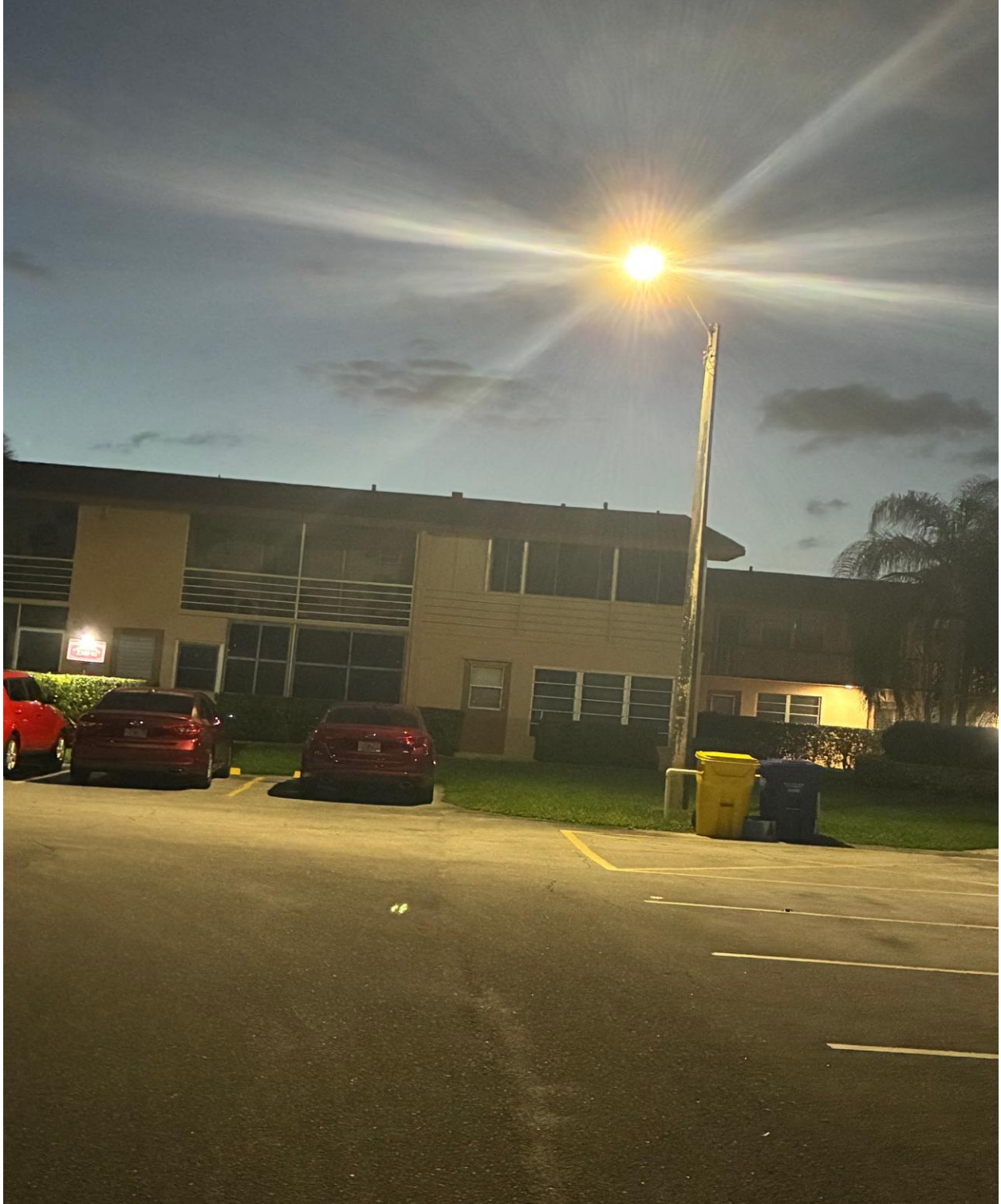
DORCHESTER B- THIS STREETLIGHT WAS REPAIRED BY FPL.
