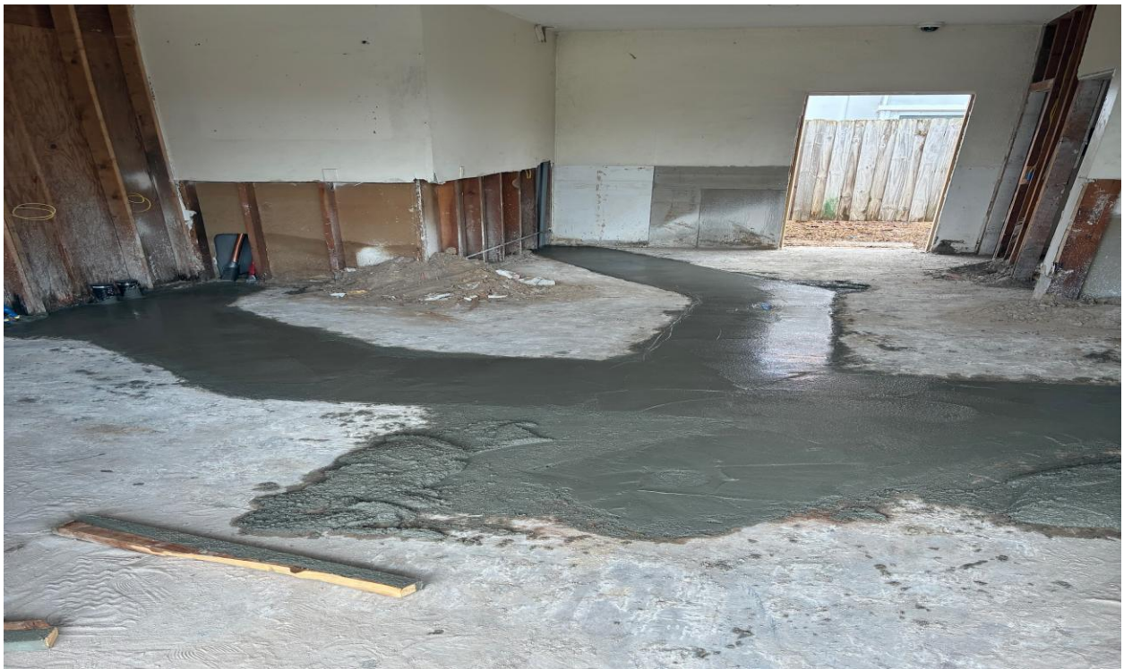
PLYMOUTH LAUNDRY- CONCRETE FLOORS WERE POURED ON 3/14.
