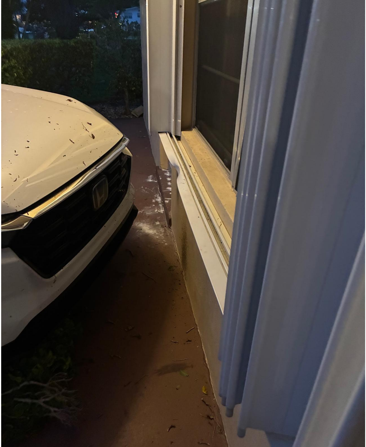
NORTHAMPTON M- THE SUV STOPPED JUST SHORT OF THE BUILDING.
