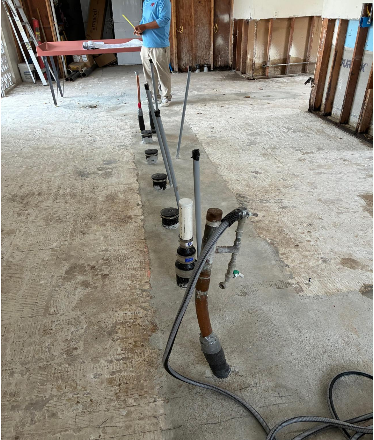
PLYMOUTH LAUNDRY- CONCRETE FLOORS WERE POURED ON 3/14.
