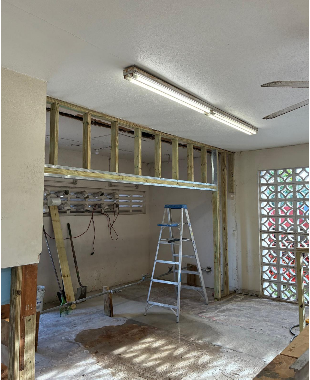
PLYMOUTH LAUNDRY- THIS FRAMING IS FOR THE DRYER AREA.
