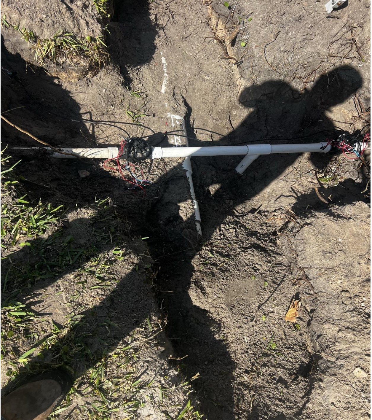
ANDOVER K- IRRIGATION LEAK REPAIRED BY SEACREST SERVICES.
