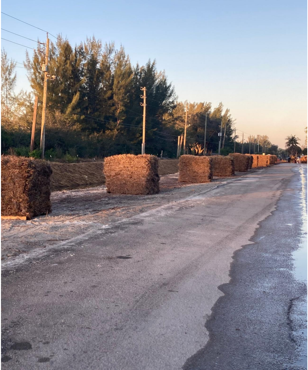
ANDOVER SECTION- NEW SOD READY TO BE INSTALLED ALONG SOUTH CANAL.
