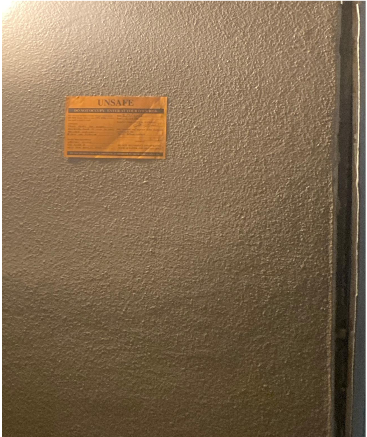
DOVER C- THE PBC BUILDING INSPECTOR TAGGED THE UNIT UNSAFE FOR OCCUPANCY.
