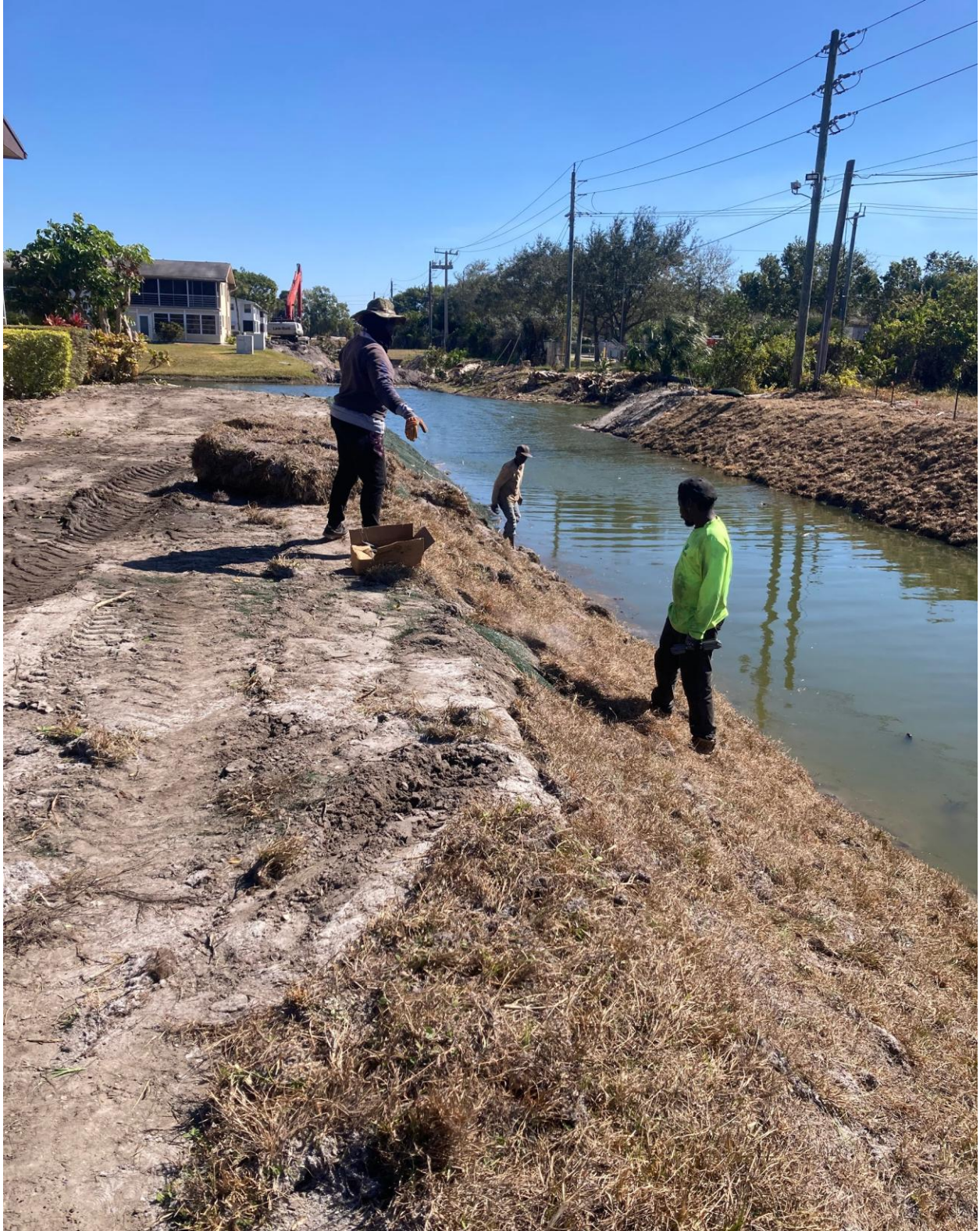
ANDOVER SECTION- SOD WAS INSTALLED ALONG THE CANAL BANKS ON 2/7.
