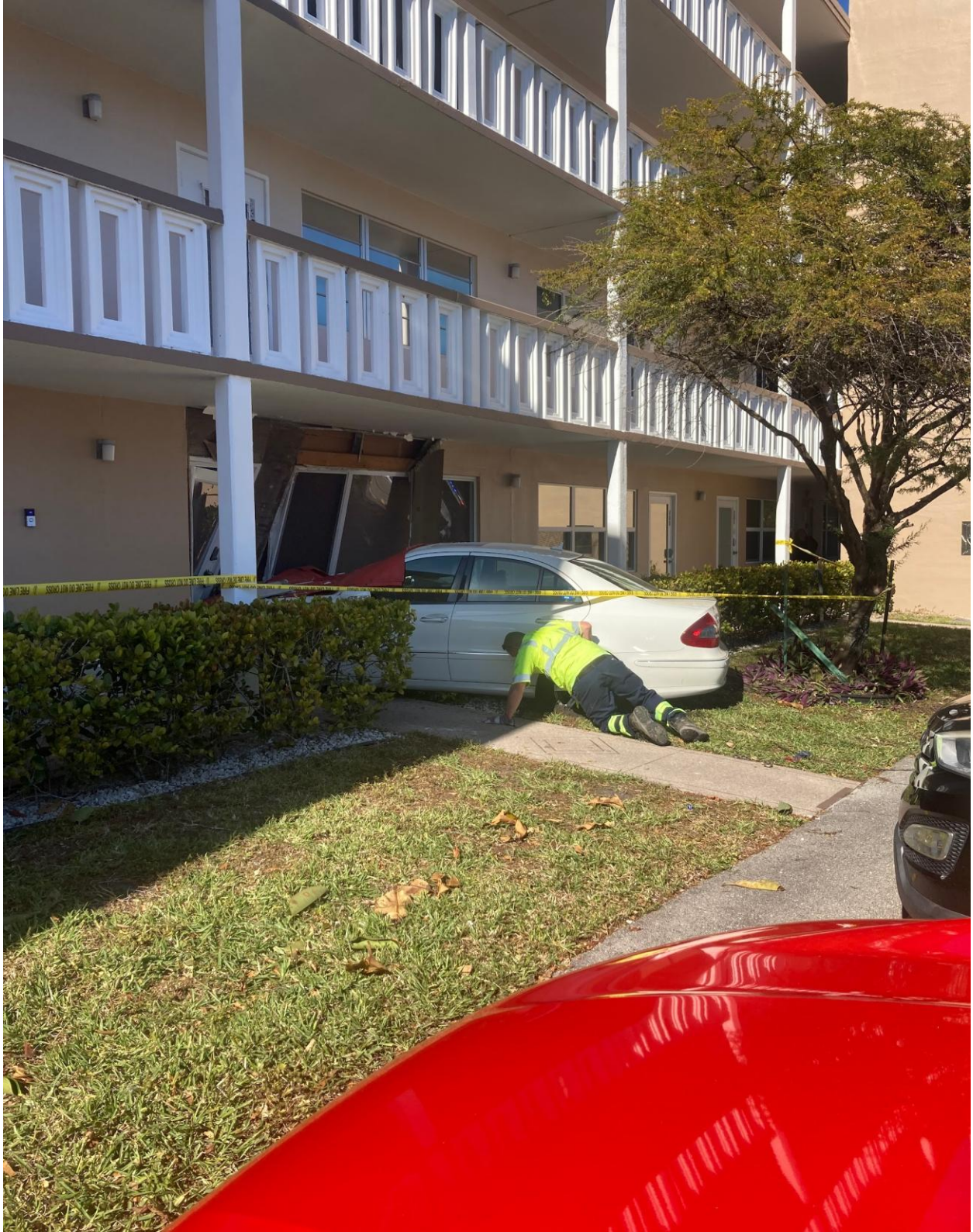
DOVER C- 2/7, CAR VS. BUILDING. THE DRIVER WAS UNHURT. THE UNIT WAS UNOCCUPIED AT THE TIME OF THE CRASH.
