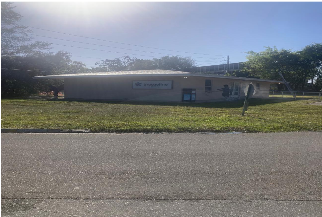
5400 FAIRWAY STREET- EM PRESSURE CLEANING, WELL, PRESSURE CLEANED THE ROOF, EXTERIOR WALLS, AND WALKWAYS AT THIS BUILDING ON 1/27.
