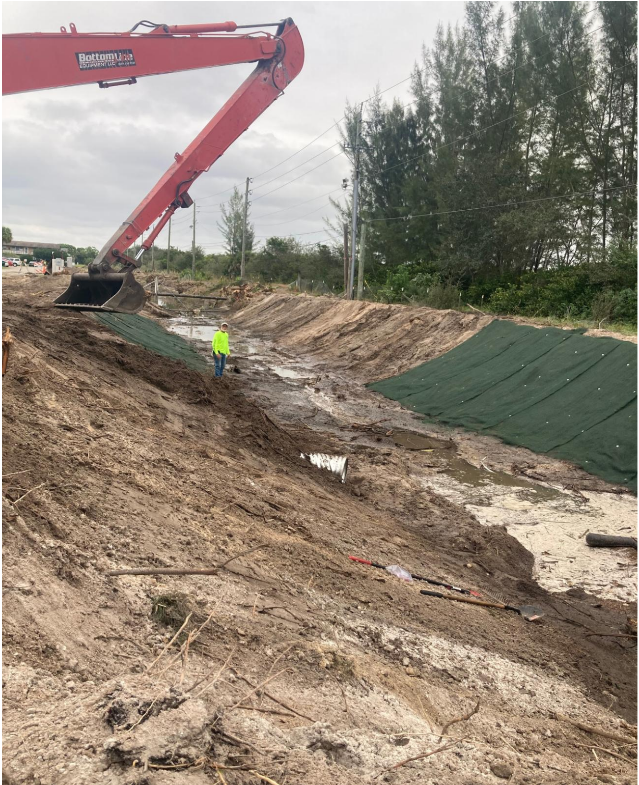
ANDOVER SECTION- CONSTRUCTION WORK AT SOUTH CANAL CONTINUES.
