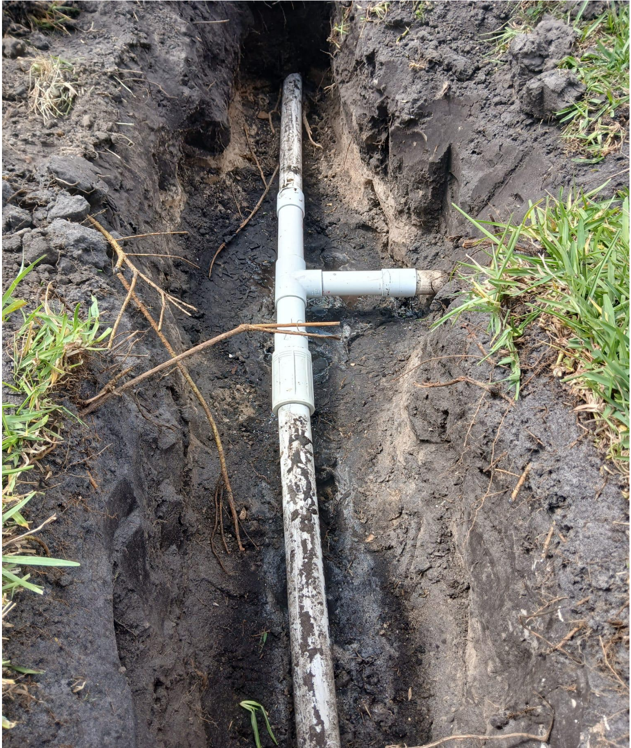
ANDOVER E- SEACREST SERVICES REPAIRED THIS UNDERGROUND IRRIGATION SUPPLY PIPE ON 5/6.
