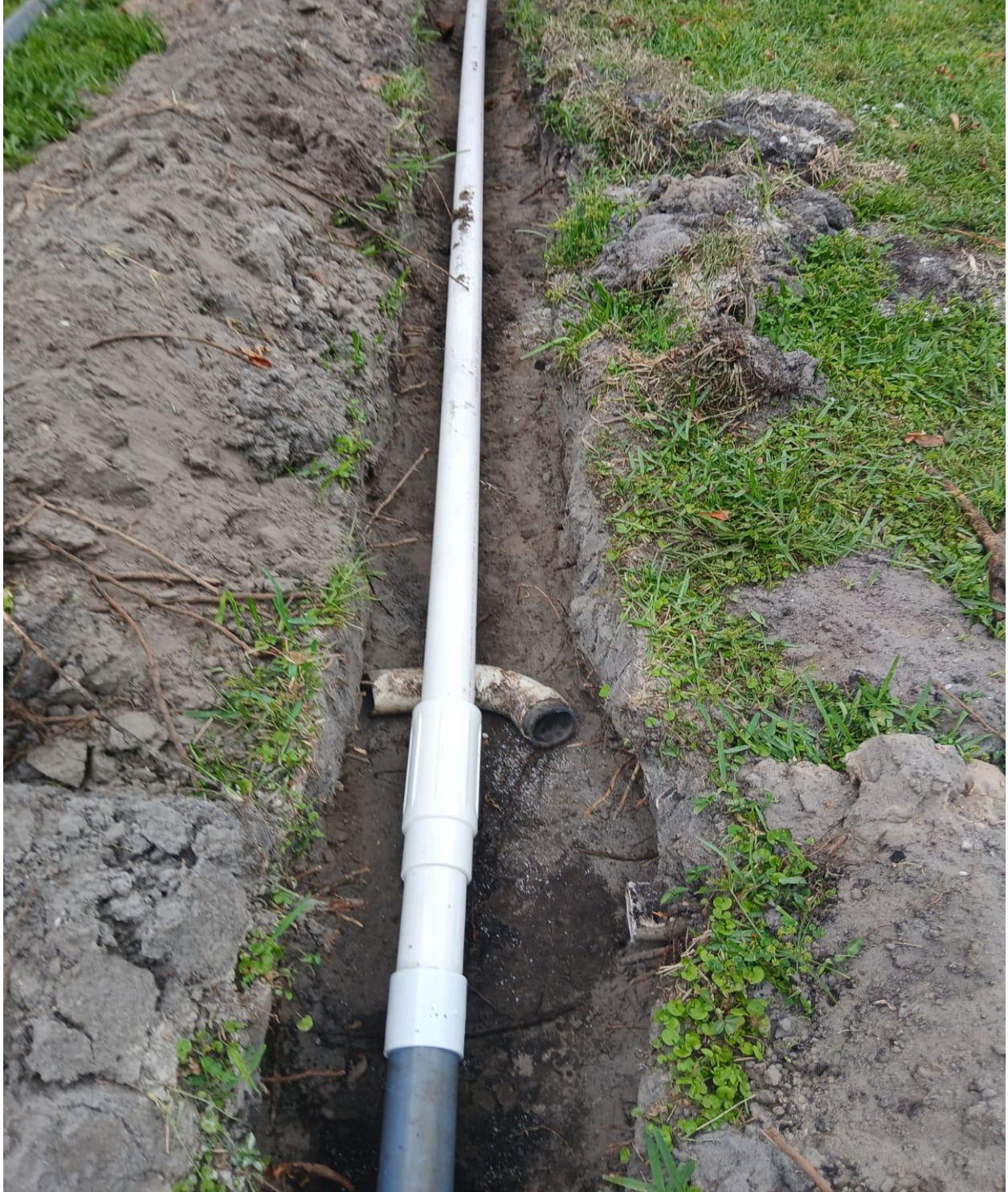
NORWICH D- SEACREST SERVICES REPAIRED THIS UNDERGROUND IRRIGATION SUPPLY PIPE ON 5/6.
