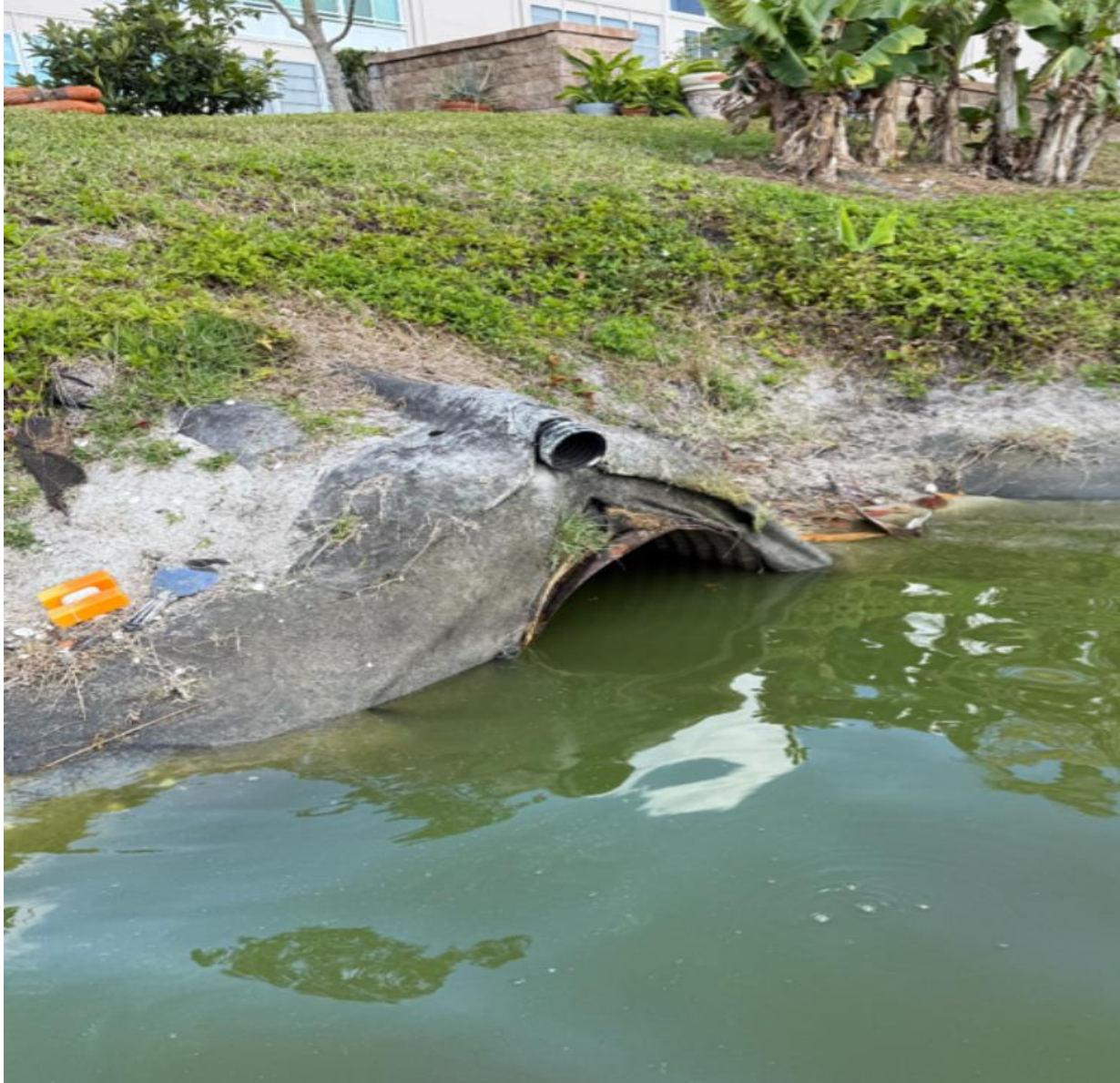
WELLINGTON J- THIS STORM DRAIN PIPE WAS FOUND TO BE CLOGGED UP WITH TREE BRANCHES AND PALM FRONDS, WHICH TRAPS SAND AND LITTER.
