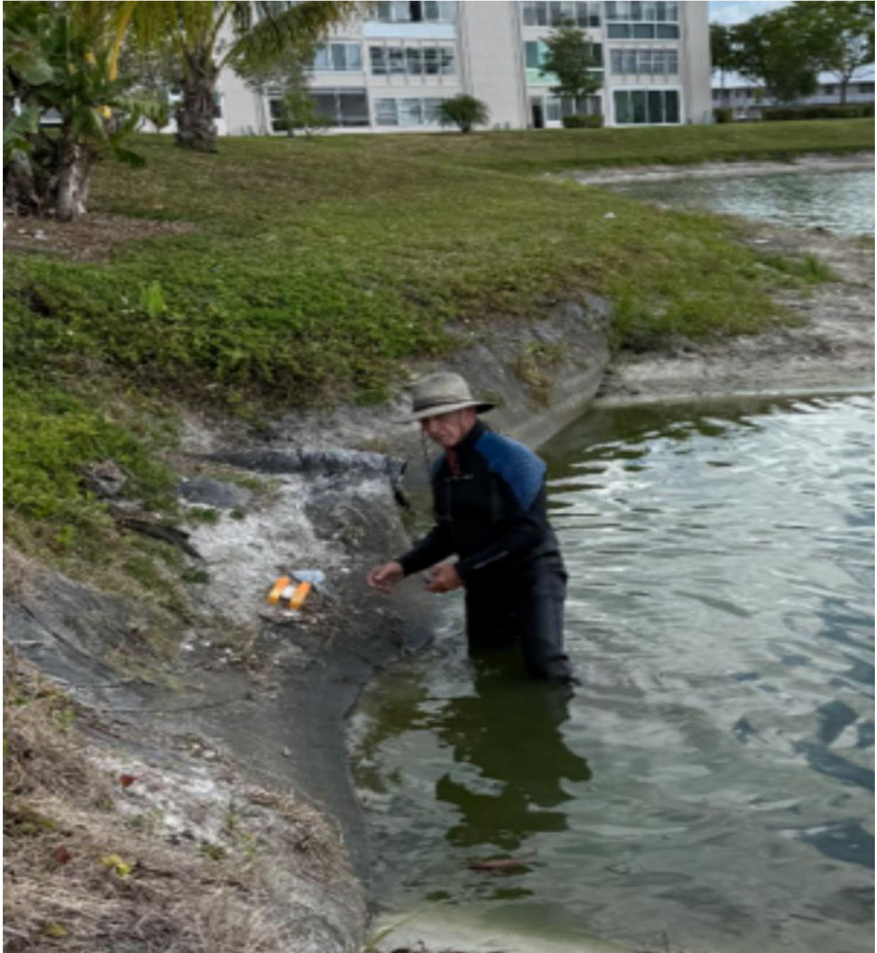
WELLINGTON J- THIS IS PETE FROM ANCHOR MARINE. HIS JOB IS TO SWIM OR CRAWL UP THIS STORM DRAIN PIPE AND CLEAR IT. WHEN THE LAKE LEVELS ARE HIGH, HE WEARS DIVING GEAR, BUT RIGHT NOW IT'S MOSTLY A CRAWLING JOB.
