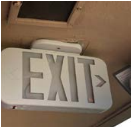
OUTDOOR EXIT SIGNS- THIS ONE IS A FAIL. IT DOES NOT LIGHT UP WHEN TESTED, AND THE PLASTIC LETTERS HAVE FADED FROM THEIR ORIGINAL RED COLOR. THEY ALSO TEND TO GET BUSTED EVERY TIME SOMEONE BUYS A NEW REFRIGERATOR OR SOFA.
