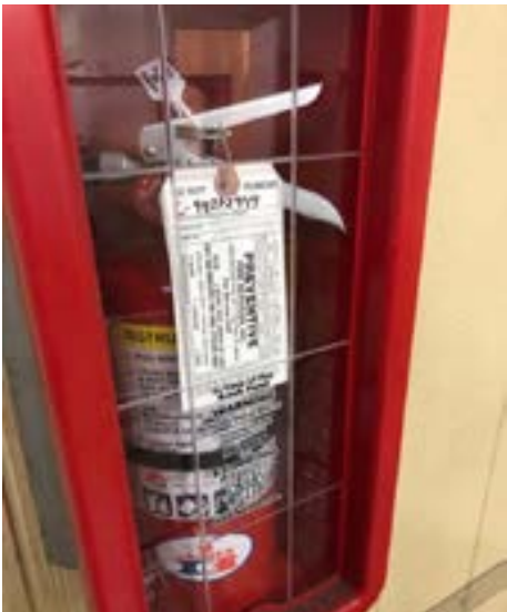
FIRE DEPARTMENT INSPECTIONS- CHECK YOUR OUTDOOR FIRE EXTINGUISHERS, MAKE SURE INSPECTION TAGS ARE CURRENT, STORAGE CABINETS ARE SOUND.
