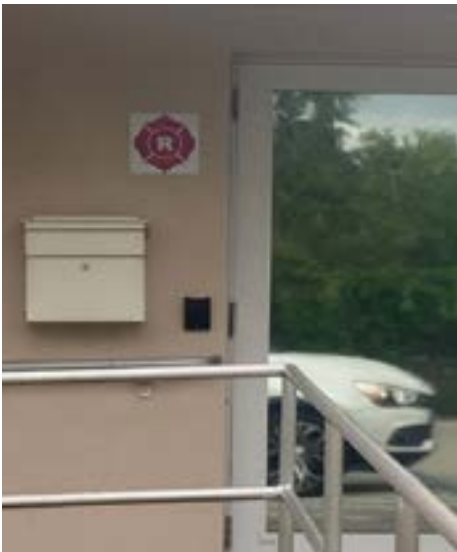
BREEZELINE OFFICE- THIS ROOF TRUSS SIGN WAS INSTALLED IN 2018 WHEN THE BUILDING WAS CONVERTED FROM A STORAGE BUILDING TO AN OFFICE BUILDING.
