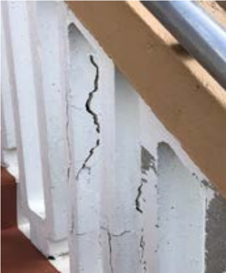
STAIRWAY RAILINGS- IF THE INSPECTOR SEES DETERIORATED BALUSTERS OR FEELS LOOSE HANDRAILS, THAT’S A FAIL.
