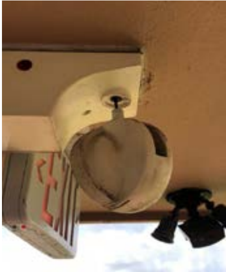
EXTERIOR STAIRWAY AND WALKWAY LIGHTS- ANOTHER FAIL. FIXTURES HANGING FROM THE CEILING AND LIGHT BULBS REMOVED.
