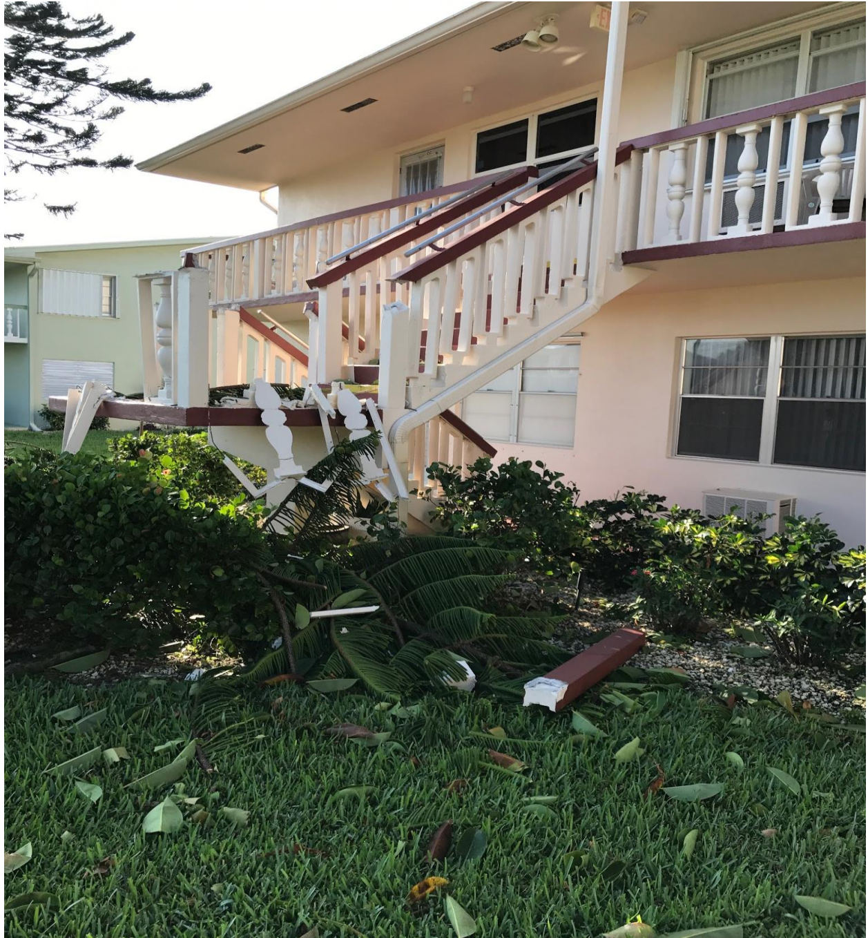
NORWICH SECTION- THE 2017 HURRICANE KNOCKED OVER A BIG NORFOLK PINE WHICH DAMAGED A STAIRCASE. IN THAT STORM, THERE WERE QUITE A FEW MAJOR DAMAGES CAUSED BY MASSIVE TREES THAT WERE TOO CLOSE TO BUILDINGS.
