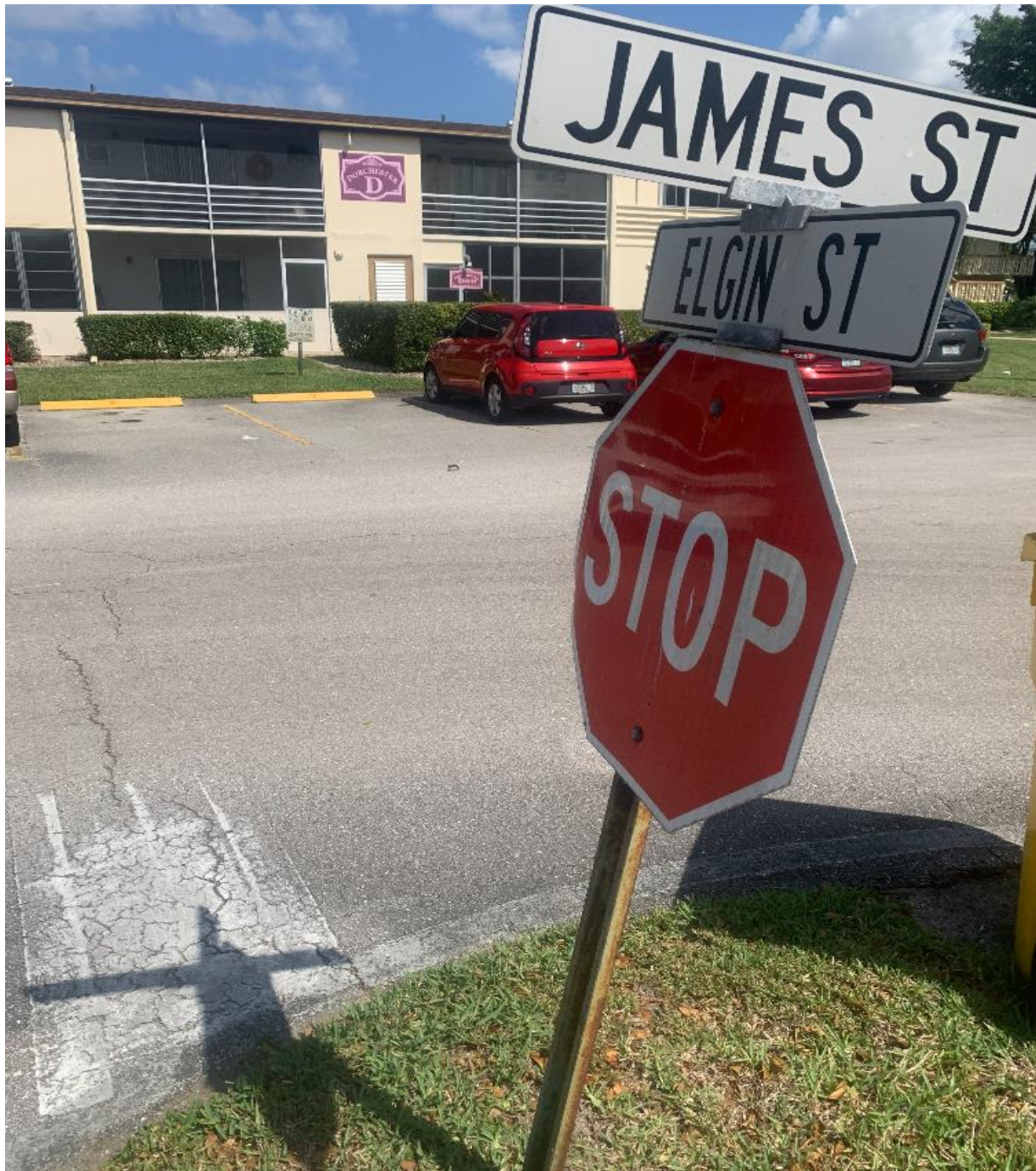
DORCHESTER SECTION- ANOTHER MIDGET STOP SIGN WITH A FADED STOP BAR.
