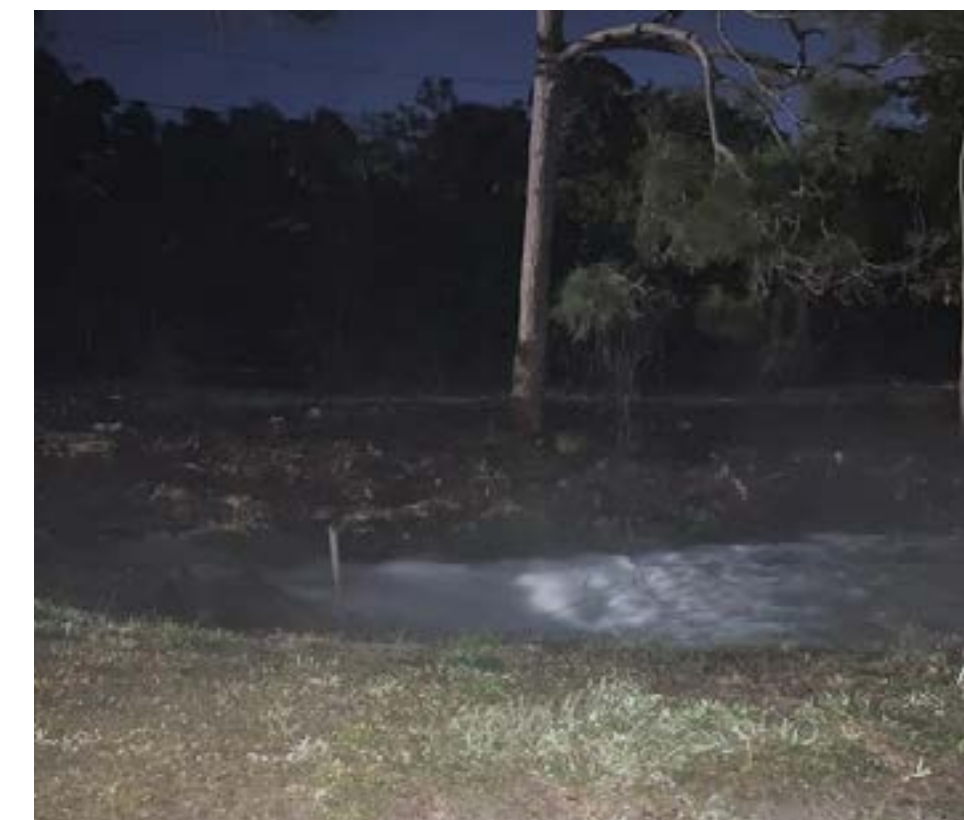
NORTH CANAL- THIS SUPPLY OF RECLAIMED WATER FROM PBC WATER UTILITIES KEEPS OUR LAKES FROM COMPLETELY DRYING OUT, BUT ONLY RAIN CAN BRING THE LAKES TO NORMAL LEVELS.
