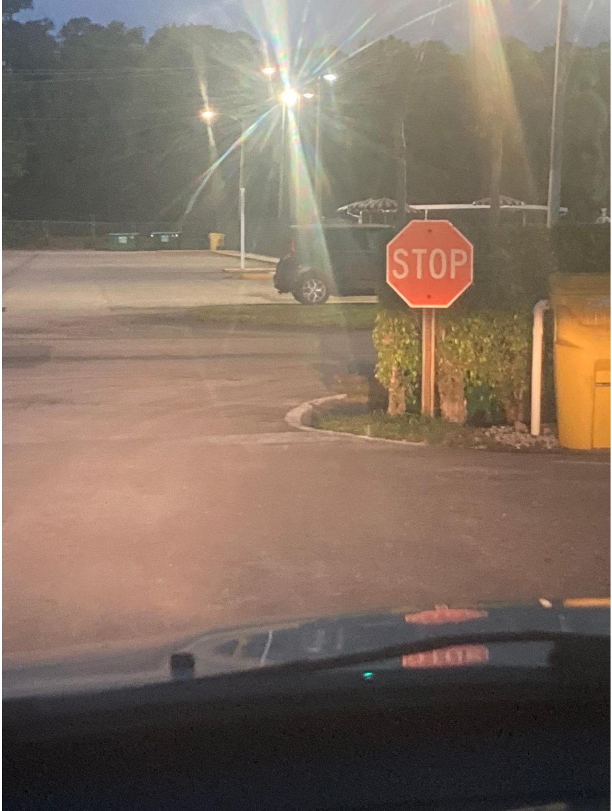
HASTINGS SECTION- MIDGET STOP SIGN AND FADED STOP BAR.
