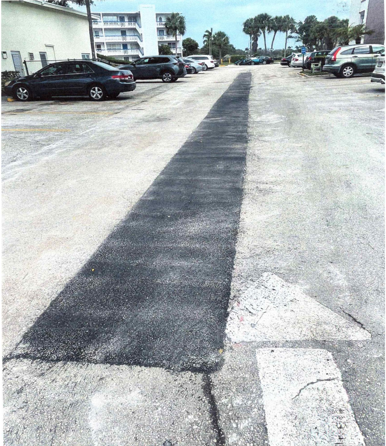
GREENBRIER C- PAVING REPAIR COMPLETE.
