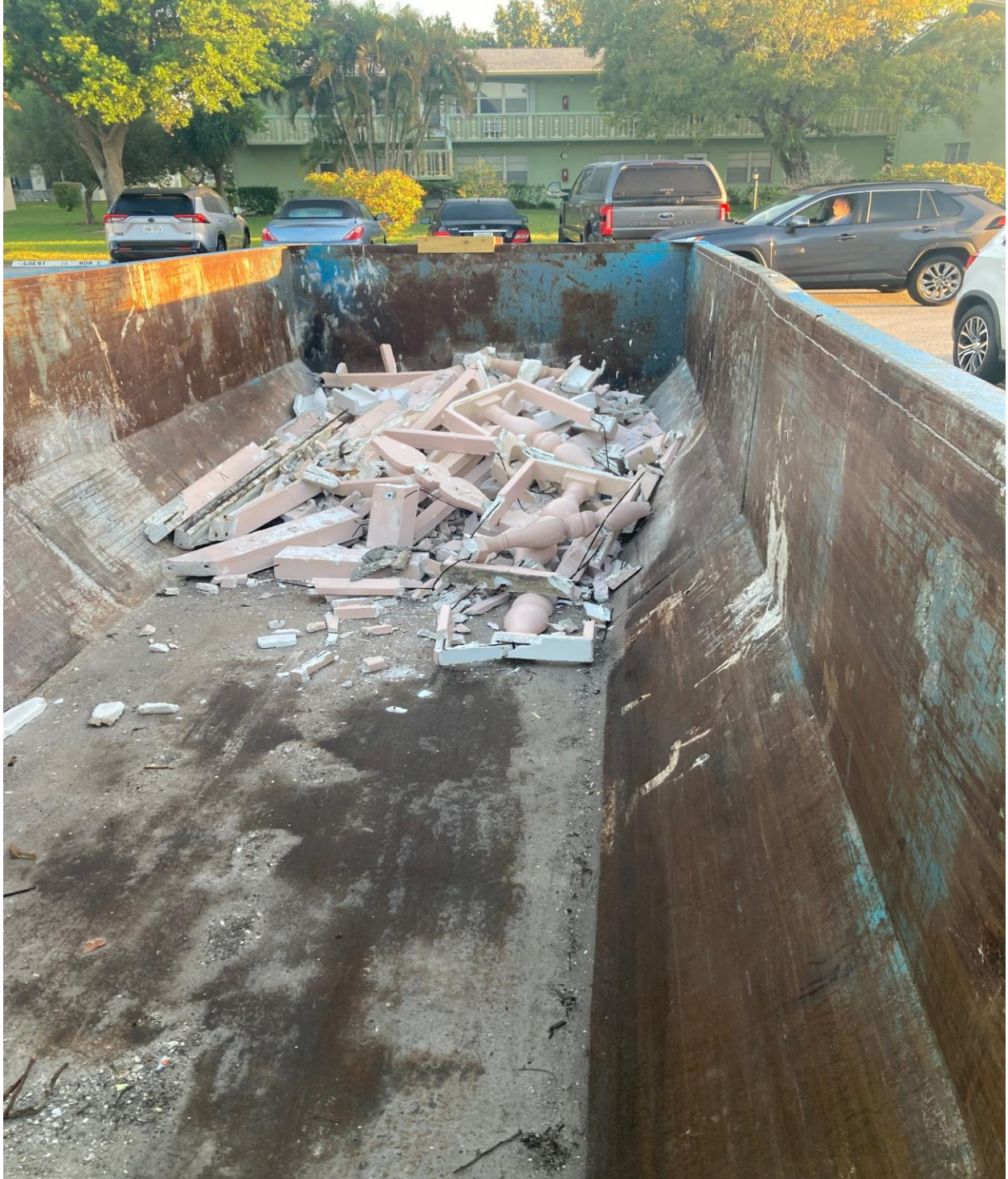
NORWICH B- DETERIORATED RAILINGS, BANISTERS, AND BALUSTERS ARE BEING REMOVED AND REPLACED. THIS ASSOCIATION IS ON ITS WAY TO BEING A SAFE PLACE TO LIVE.
