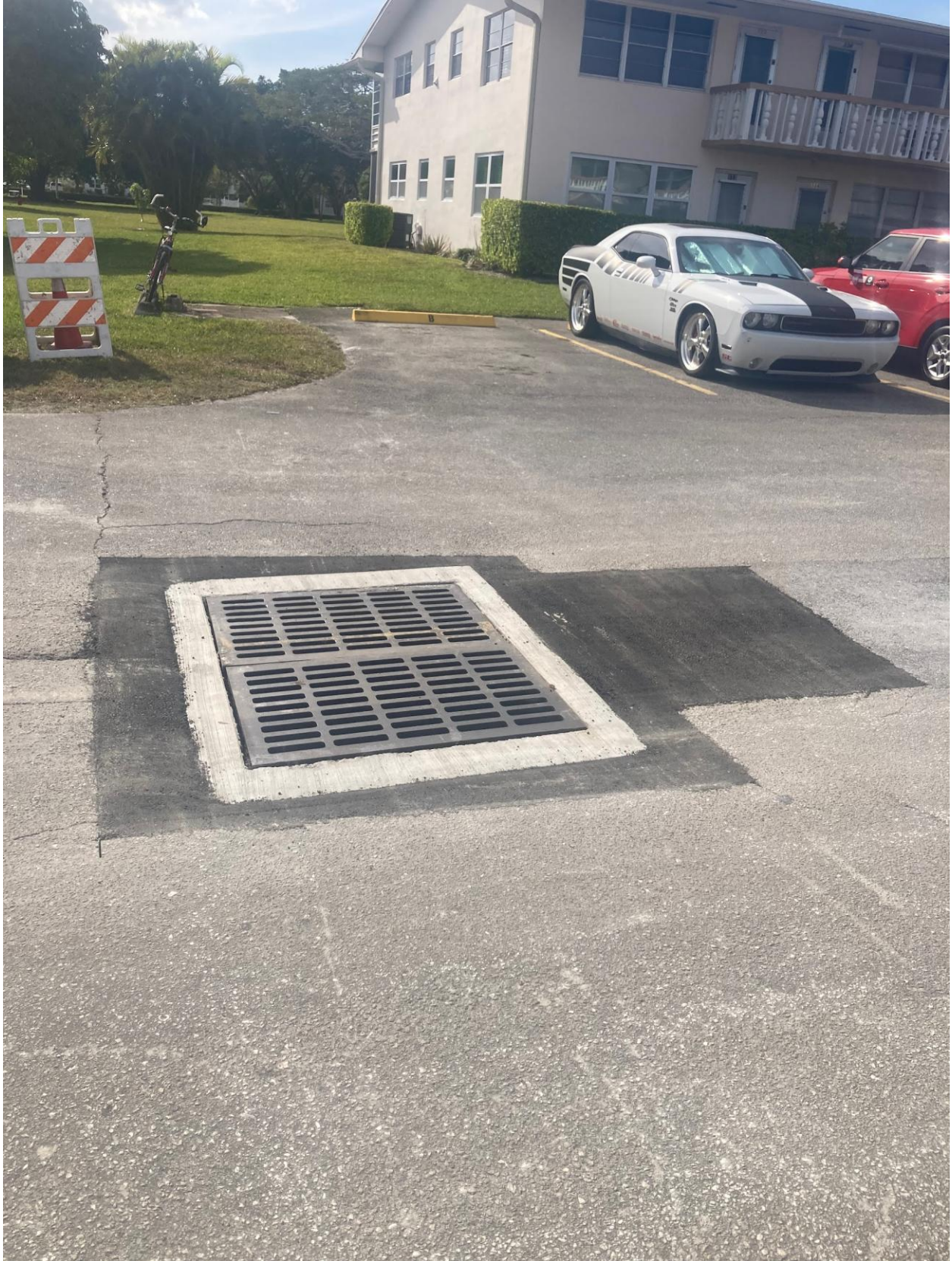
KENT SECTION- CATCH BASIN REPAIR COMPLETE.
