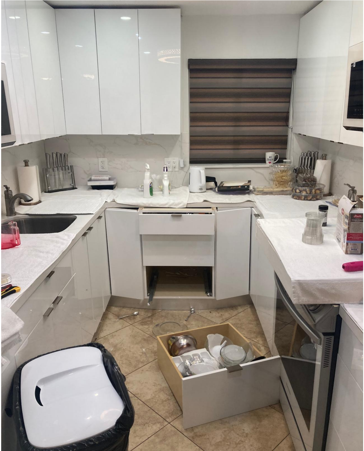
111 PLYMOUTH M- THE FRONT WALL WAS PUSHED IN, AND DAMAGED THE KITCHEN CABINETS.
