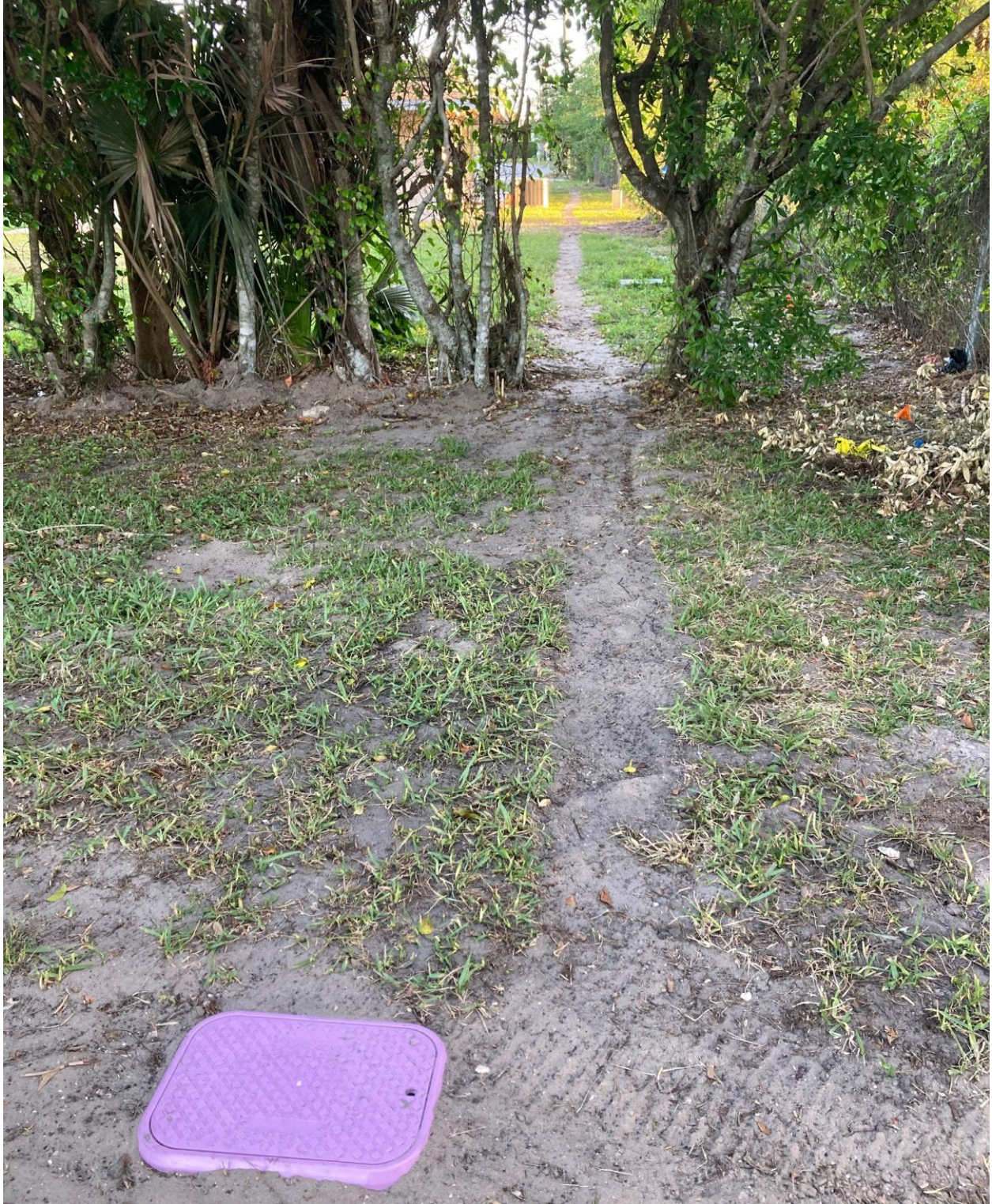
SOUTHAMPTON A- IRRIGATION LINE INSTALLATION COMPLETE.
