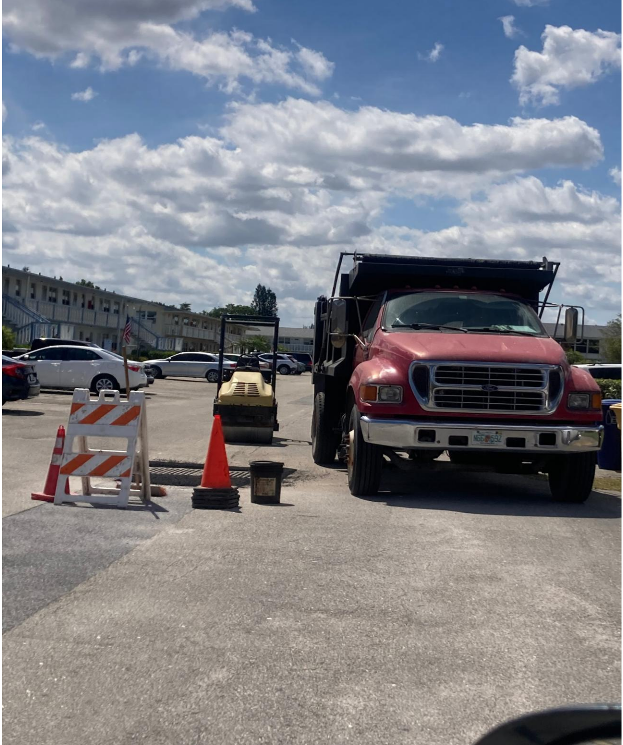
KENT SECTION- FEDERAL MAINTENANCE COMPLETED THIS REPAIR ON 3/22.
