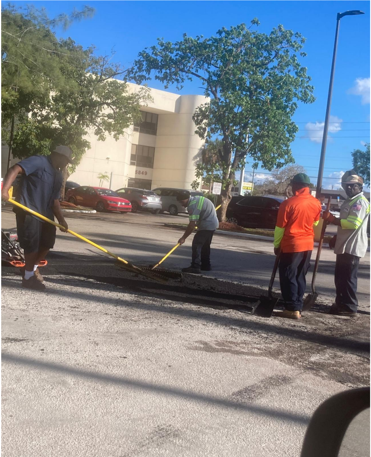
WEST DRIVE- PAVING REPAIR BY SUNSHINE SERVICES UNLIMITED, 2/26.
