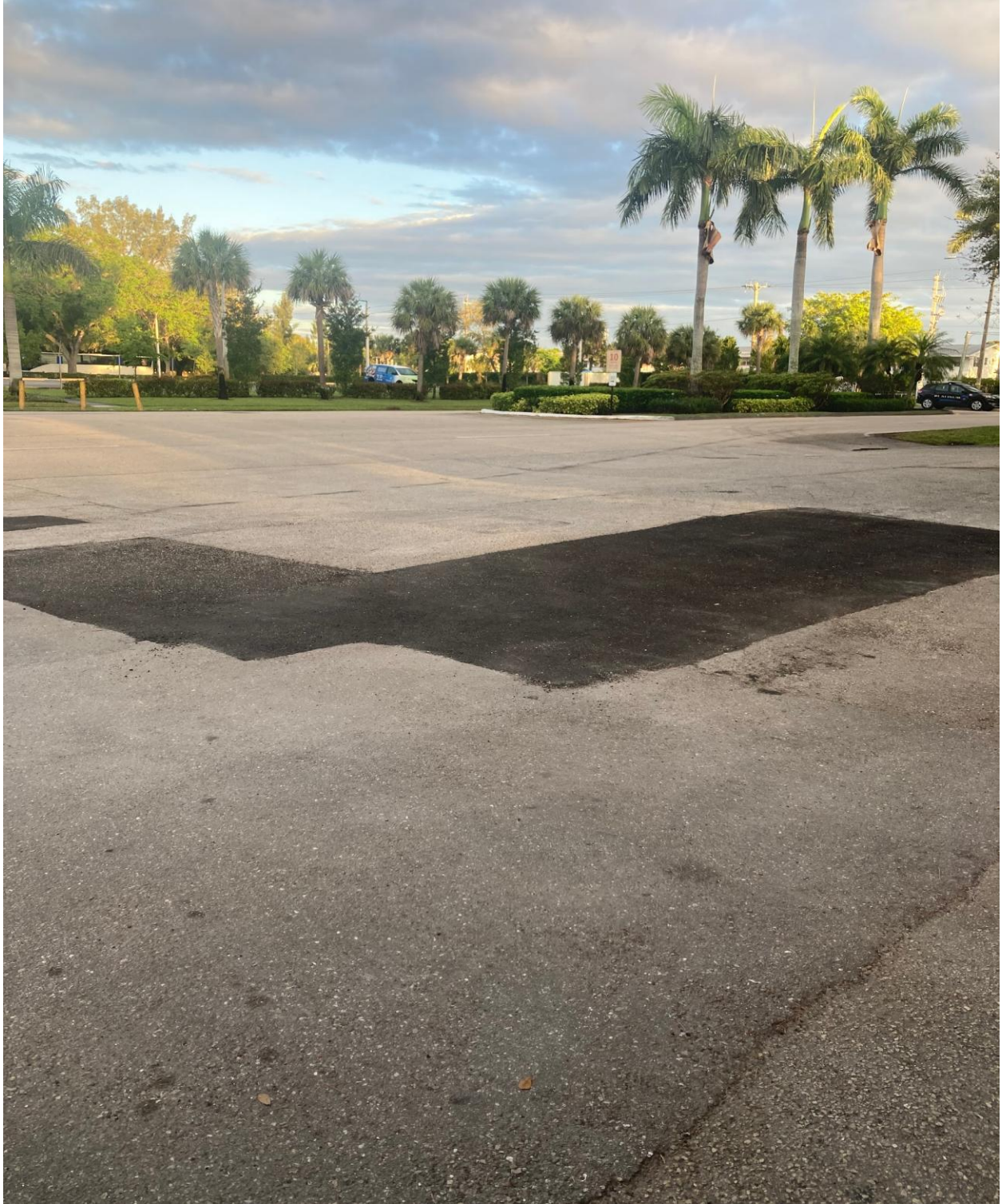
WEST DRIVE- PAVEMENT REPAIR COMPLETE.
