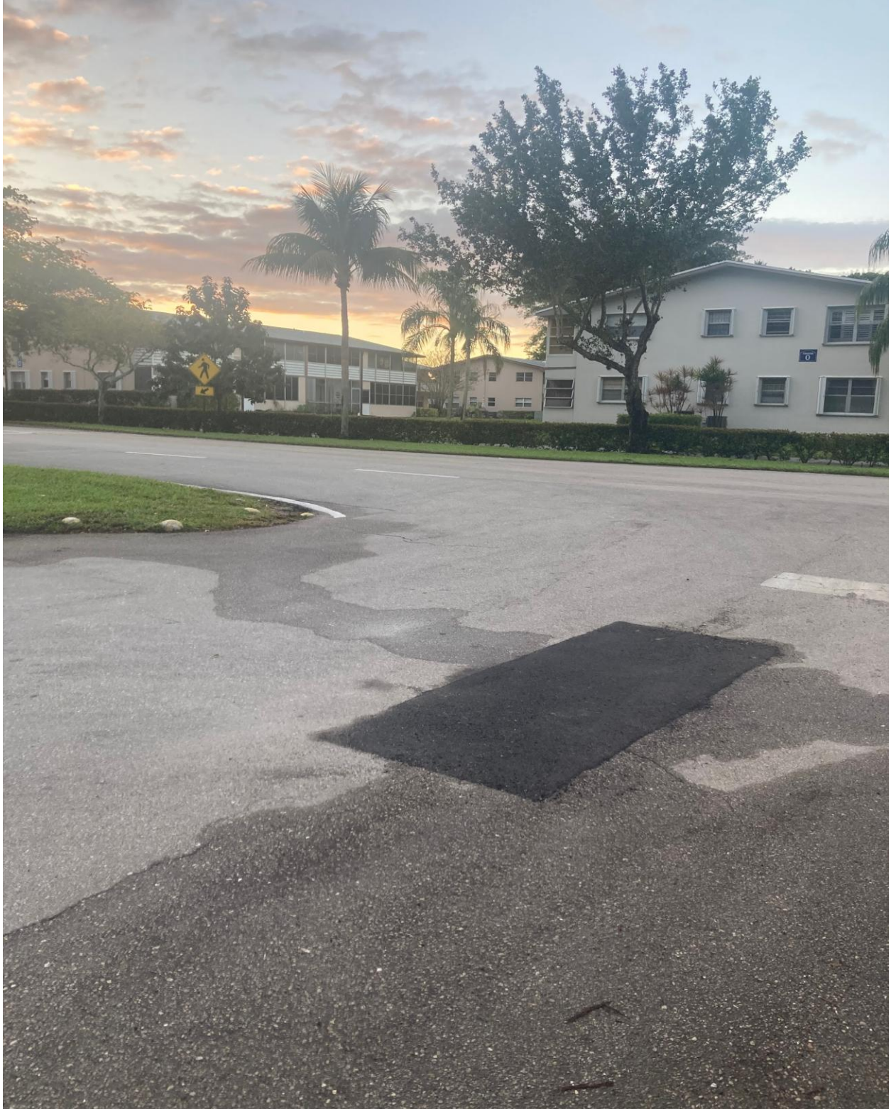
OXFORD SECTION- PAVEMENT REPAIR COMPLETE.
