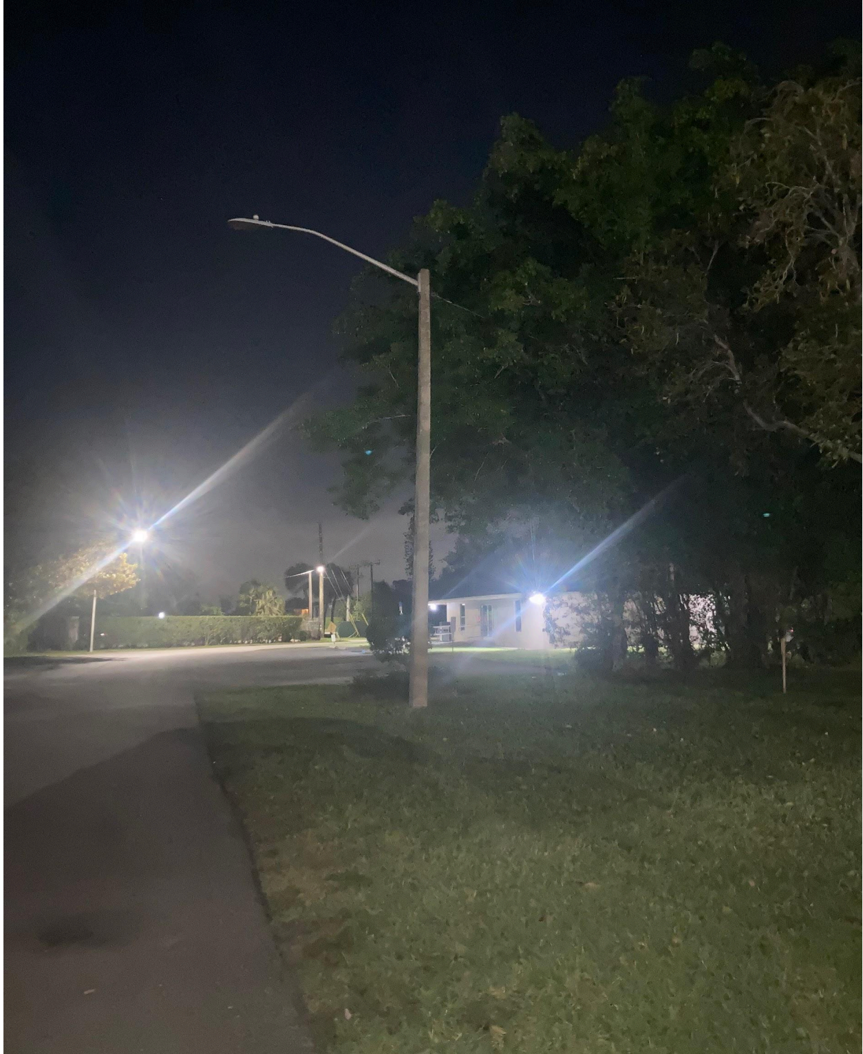
FAIRWAY STREET- THIS STREETLIGHT, NEAR SOUTHAMPTON A, IS STILL DARK. THE FPL REPAIR TICKET NUMBER IS 45669.
