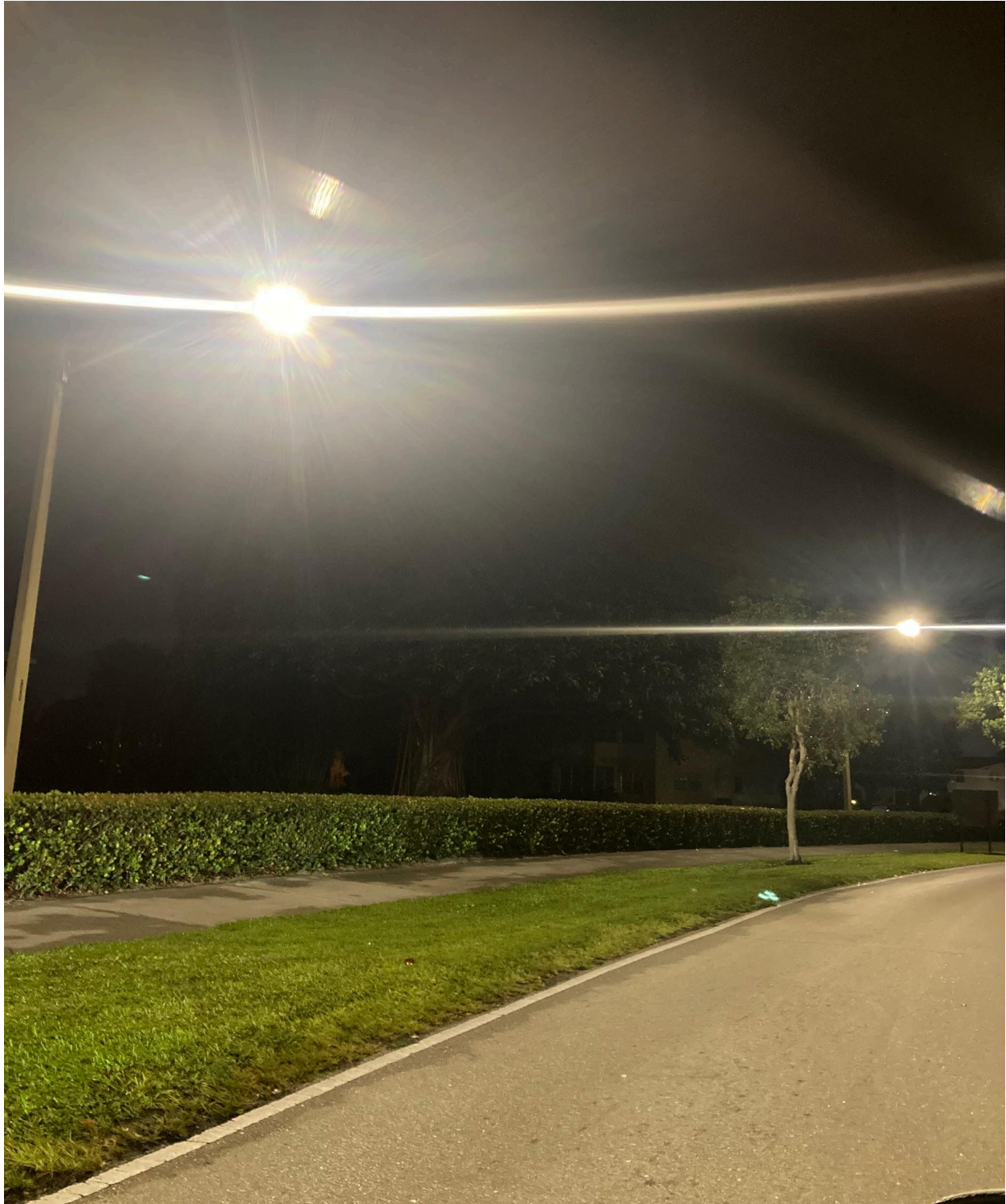
WALTHAM SECTION- THESE TWO STREETLIGHTS WERE REPAIRED BY FPL ON 3/24.
