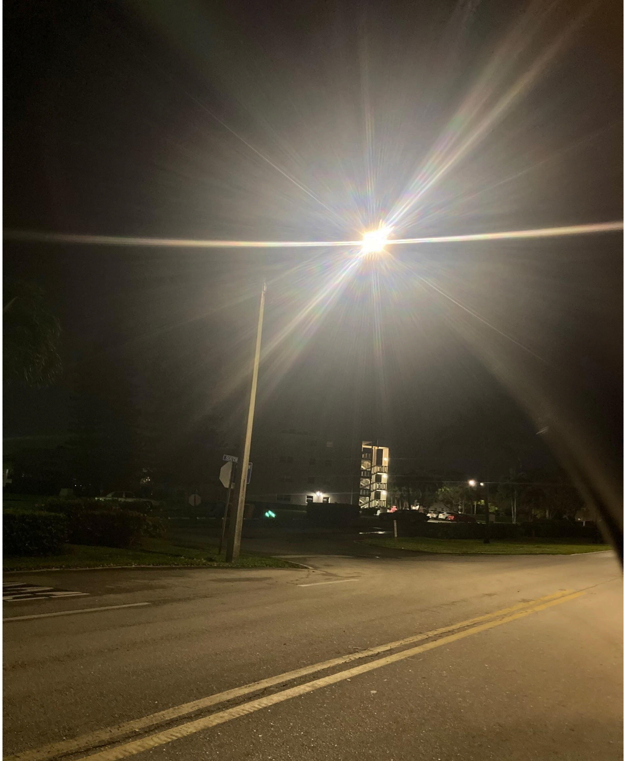
WELLINGTON H/J- THIS STREETLIGHT WAS REPAIRED BY FPL ON 3/24.
