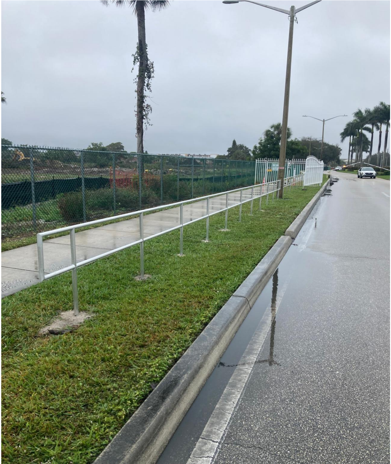
CENTURY BOULEVARD- RAILING INSTALLATION COMPLETE.
