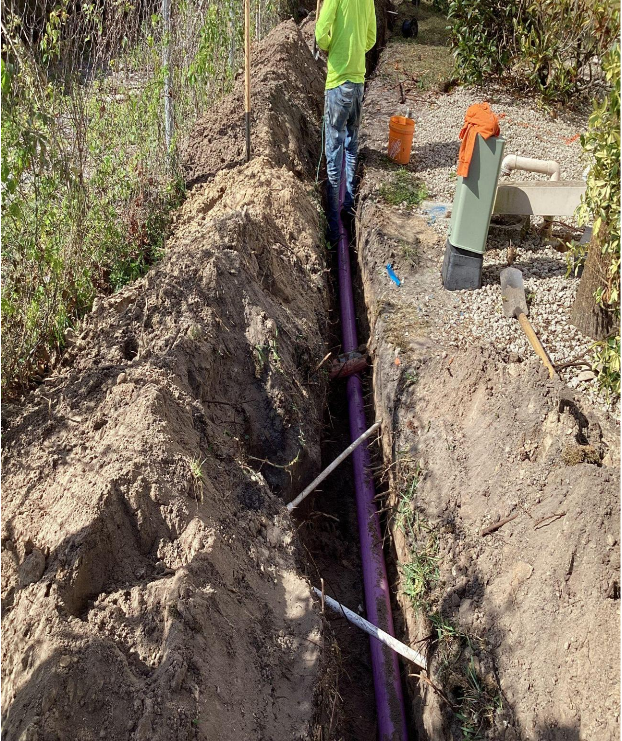
GREENBRIER SECTION- INSTALLATION OF NEW IRRIGATION SUPPLY PIPES IS COMPLETE.
