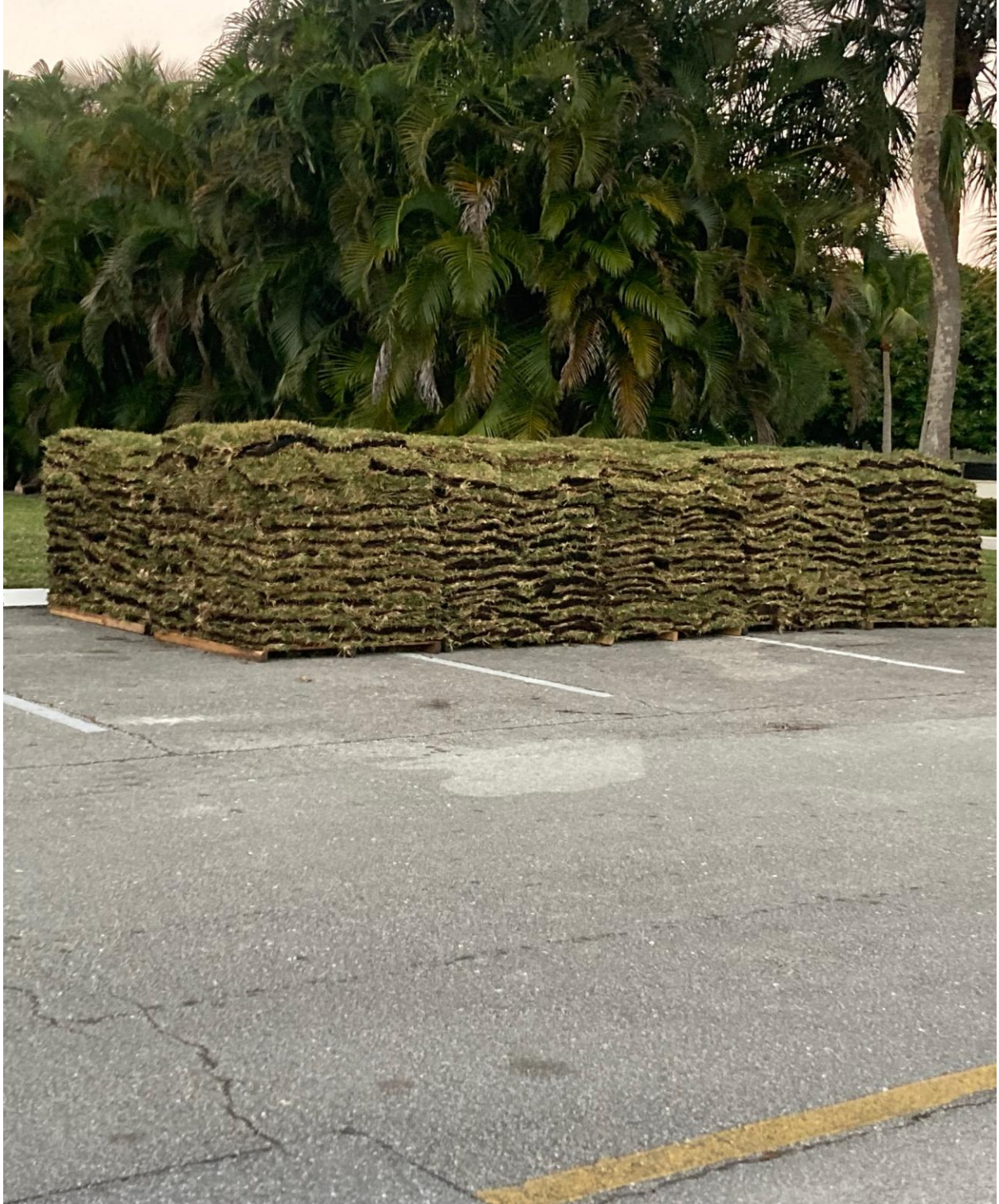
GOLFS EDGE- SOD DELIVERY FOR THE IRRIGATION REROUTE PROJECT.
