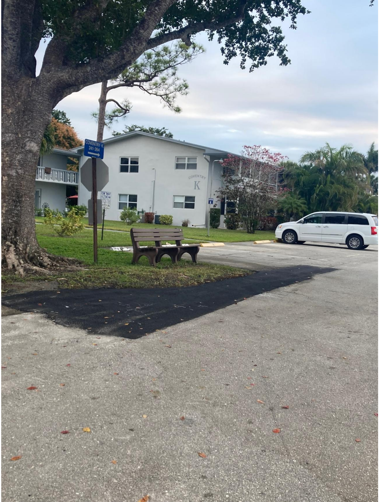
COVENTRY SECTION- PAVING REPAIR COMPLETE.
