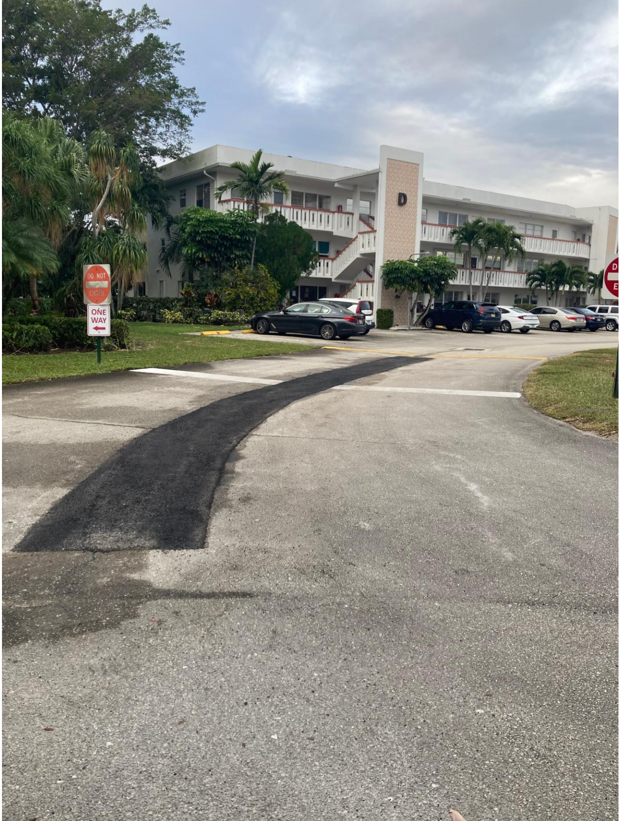
WELLINGTON SECTION- PAVING REPAIR COMPLETE.
