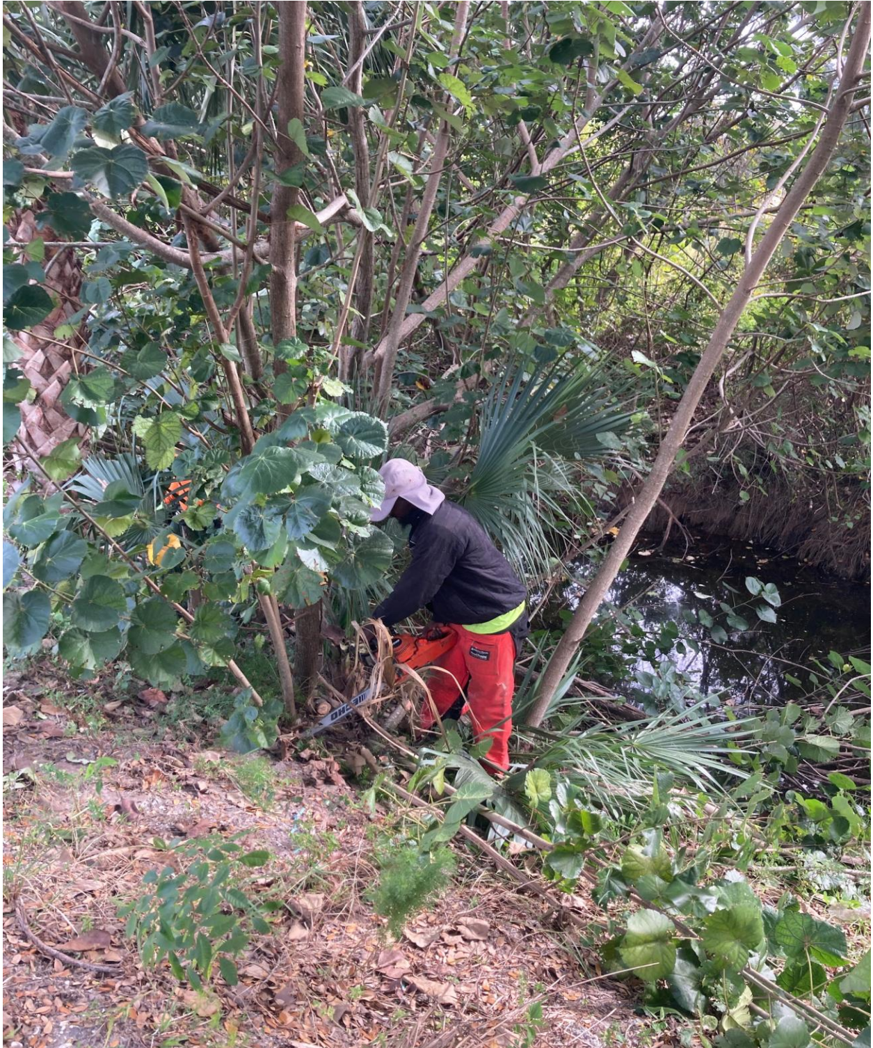
WINDSOR SECTION- SEACREST SERVICES CONTINUES LAND CLEARING AT SOUTH CANAL.
