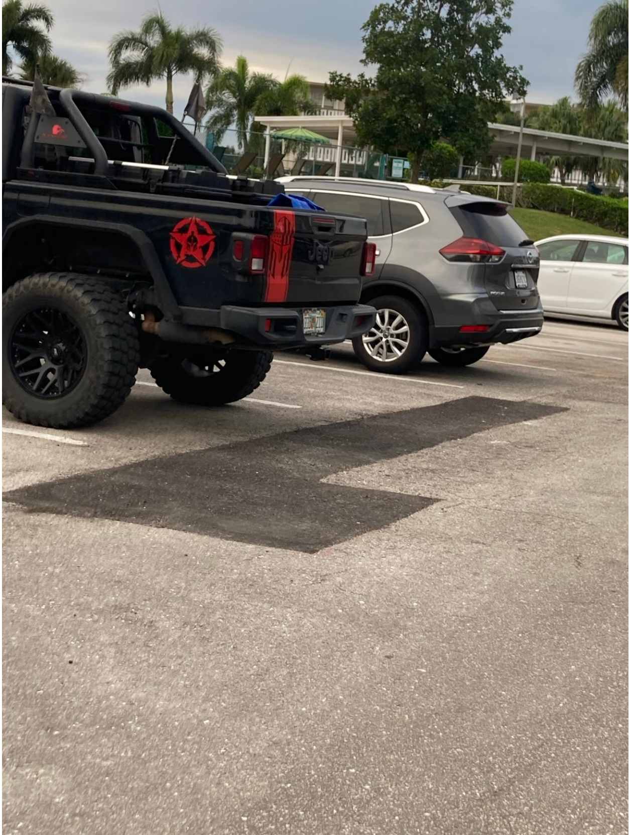
GREENBRIER SECTION- SECTION- PAVING REPAIR COMPLETE.
