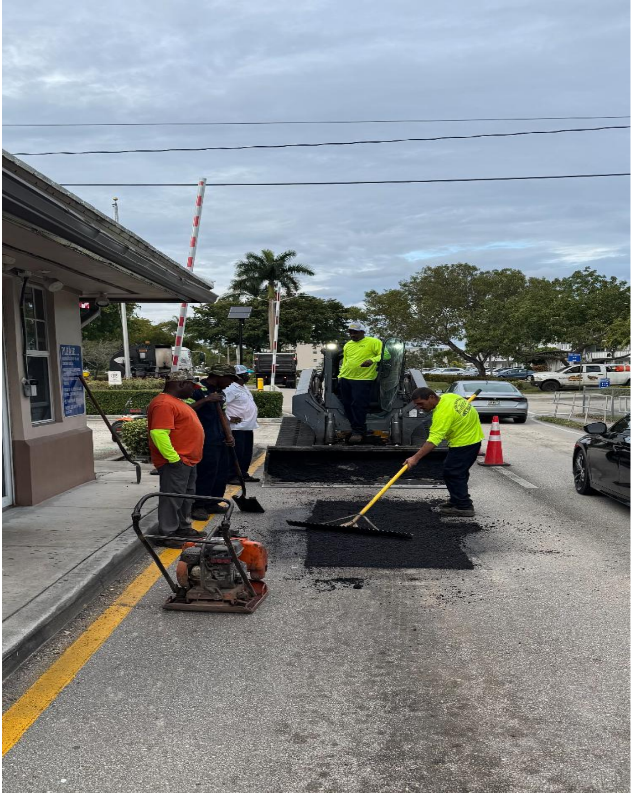
OKEECHOBEE BOULEVARD ENTRANCE- PAVING REPAIR BY SUNSHINE SERVICES UNLIMITED ON 1/16.
