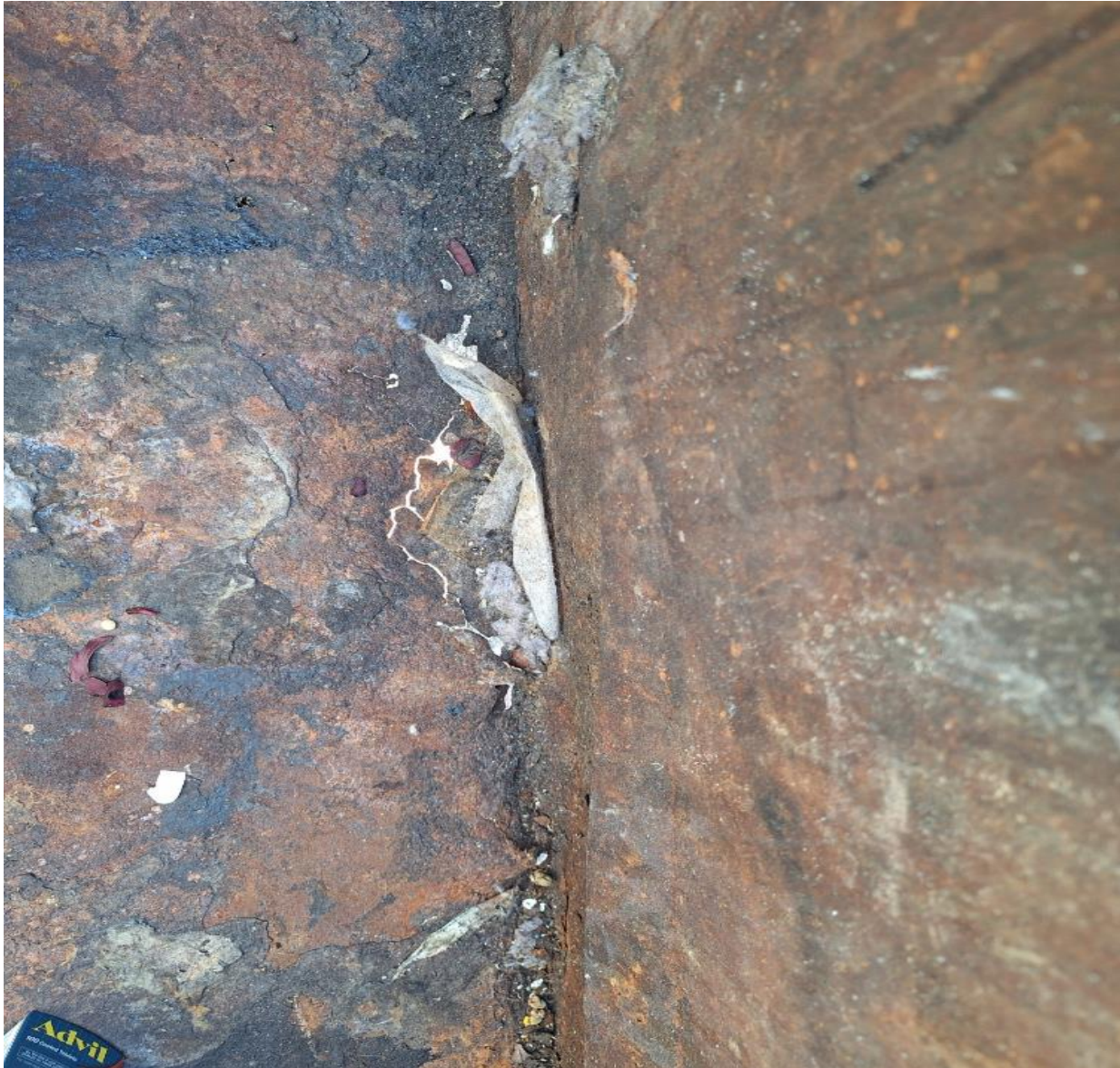
GOLFS EDGE #20- DUMPSTER WITH ROTTED OUT BOTTOM. REPORTED IN BY THE GOLFS EDGE PM. A REQUEST FOR REPLACEMENT WAS SENT TO WASTE PRO.
