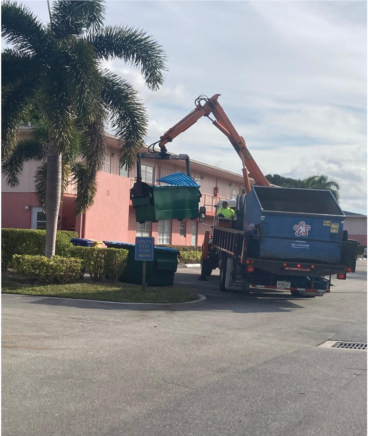
GOLFS EDGE- WASTE PRO DELIVERED REFURBISHED DUMPSTERS ON 12/10.
