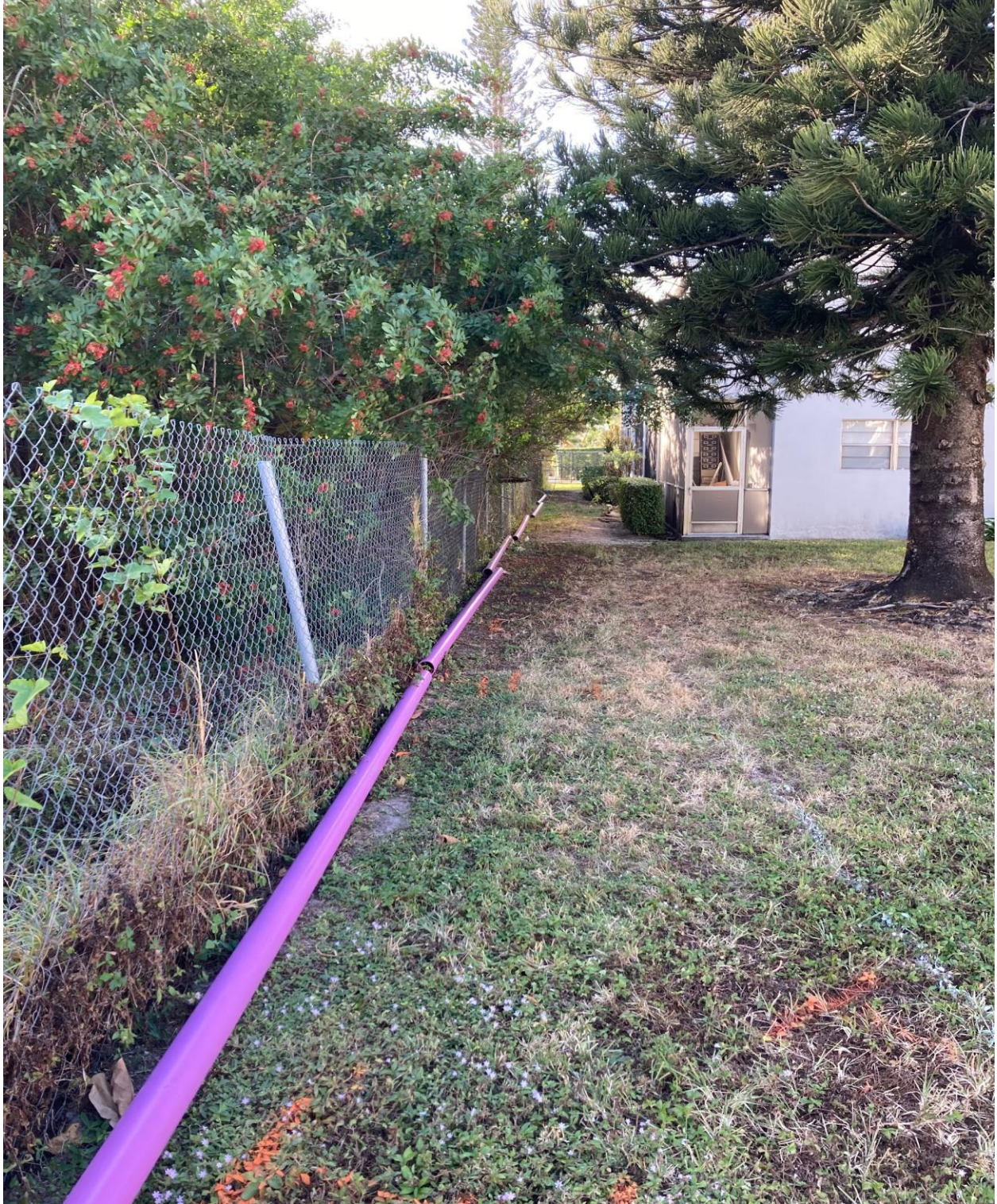
GREENBRIER B/KINGSWOOD F- THE IRRIGATION PIPE INSTALLATION BY SEACREST SERVICES CONTINUES.
