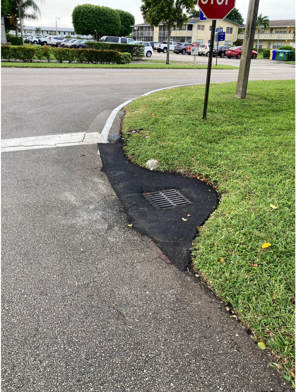
WEST DRIVE, OXFORD SECTION- PAVING REPAIR COMPLETE.
