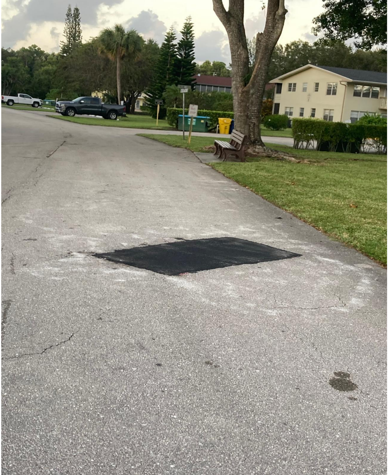
NORTHAMPTON STREET, SUSSEX SECTION- PAVING REPAIR COMPLETE.
