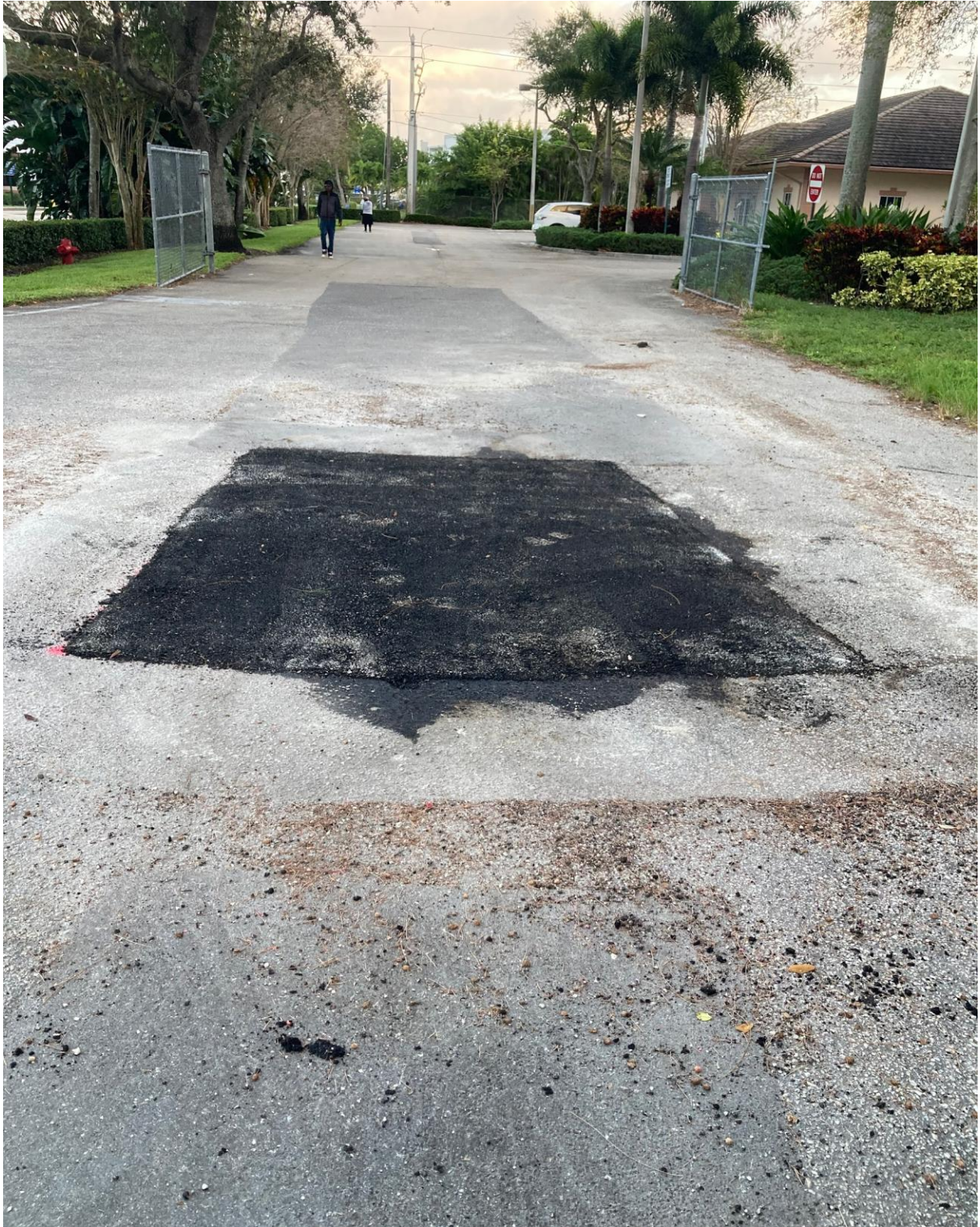
UCO OFFICE- PAVING REPAIR COMPLETE.
