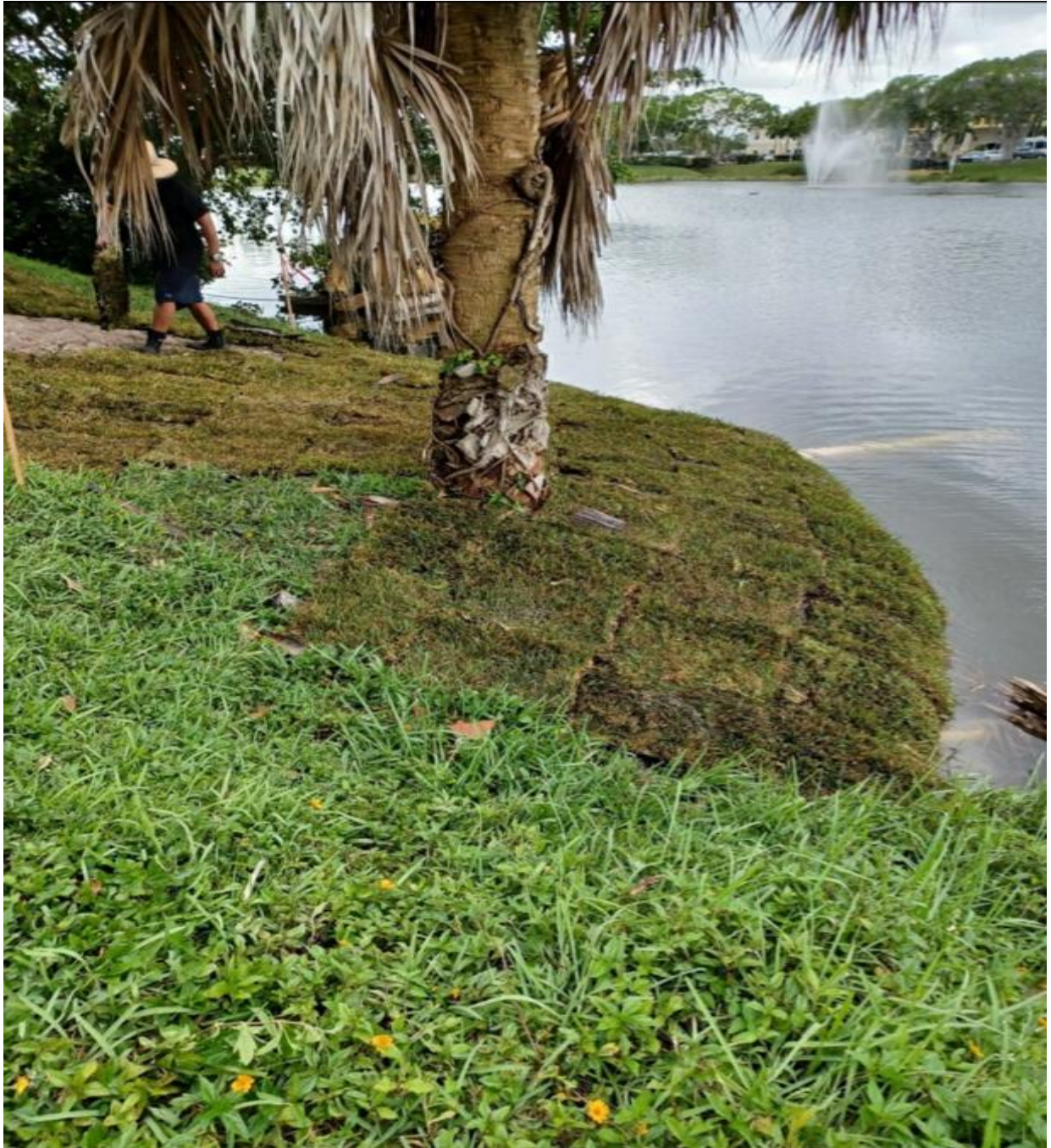
CV MEDICAL BUILDING- SHORELINE REPAIR IS COMPLETE.
