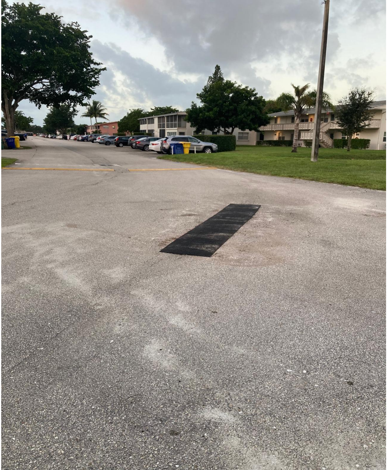
GLENCOE STREET, HASTINGS SECTION- PAVING REPAIR COMPLETE.
