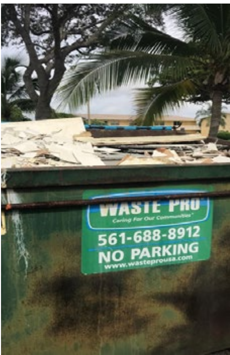
STRATFORD SECTION- THIS DUMPSTER WAS FILLED WITH CONSTRUCTION/DEMOLITION MATERIAL, LEAVING NO ROOM FOR REGULAR RESIDENTIAL GARBAGE. NO WASTE PRO TRUCK COULD PICK IT UP. THE RESPONSIBLE UNIT OWNER WAS IDENTIFIED, AND THE DUMPSTER WAS EVENTUALLY EMPTIED. CV ASSOCIATIONS, AND THEIR PROPERTY MANAGERS, NEED TO KEEP ON TOP OF THIS ACTIVITY, ESPECIALLY SINCE IT IS A FIRST SIGN OF AN UNAUTHORIZED GUT RENOVATION.
