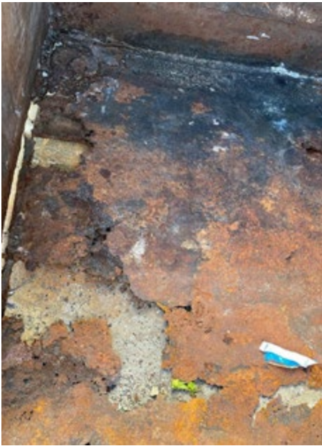
COVENTRY E- RUSTED OUT DUMPSTER. REPORTED IN BY A CV UNIT OWNER. A REQUEST FOR REPLACEMENT WAS SENT TO WASTE PRO. PLEASE SEND BUSTED DUMPSTER REPORTS TO UCOGARBAGE@GMAIL.COM. PICTURES ARE VERY HELPFUL.
