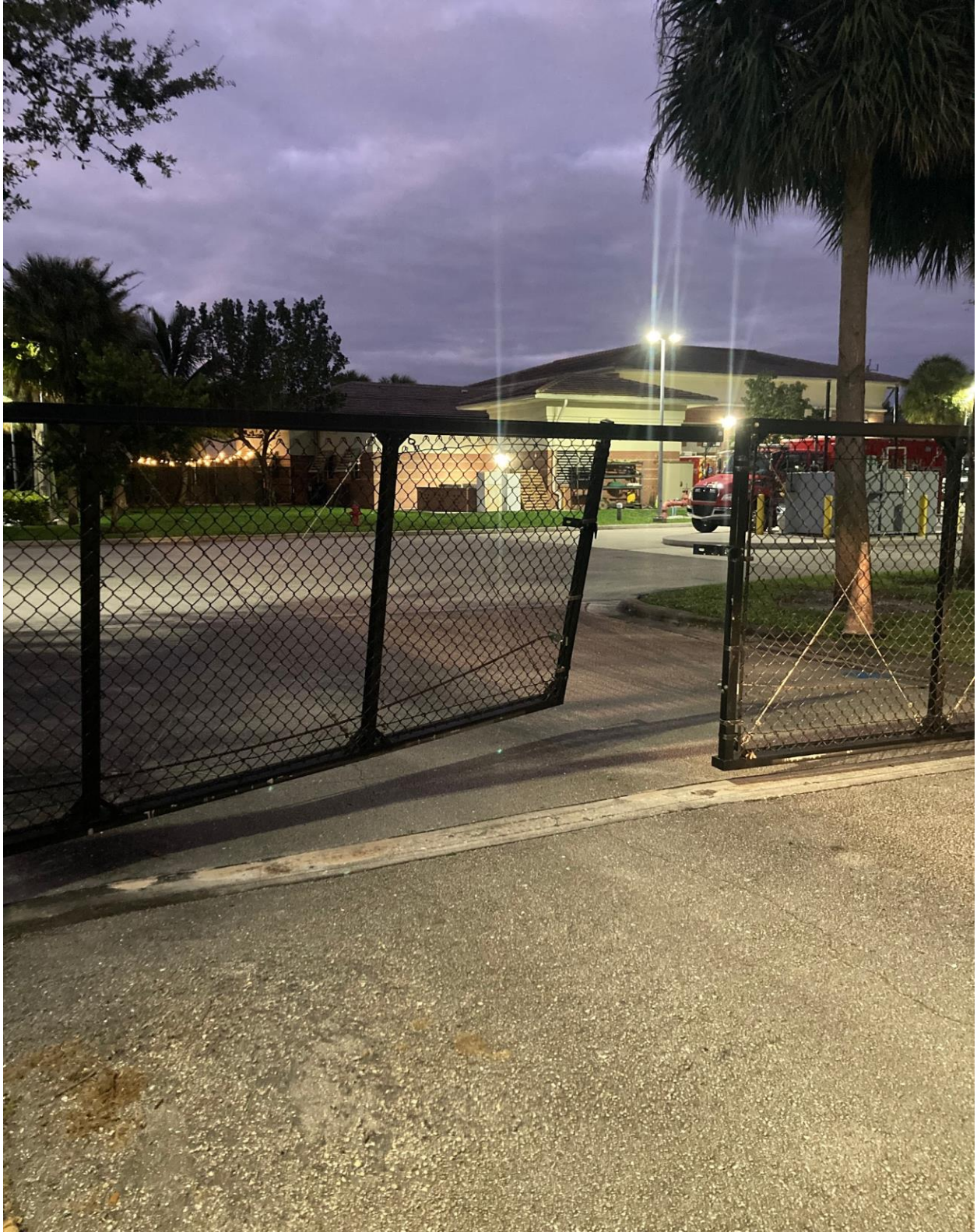
BEDFORD SECTION- PLATINUM SECURITY ROVING PATROL OFFICER LOGAN FOUND THIS SMASHED GATE EARLY AM ON 11/17.
