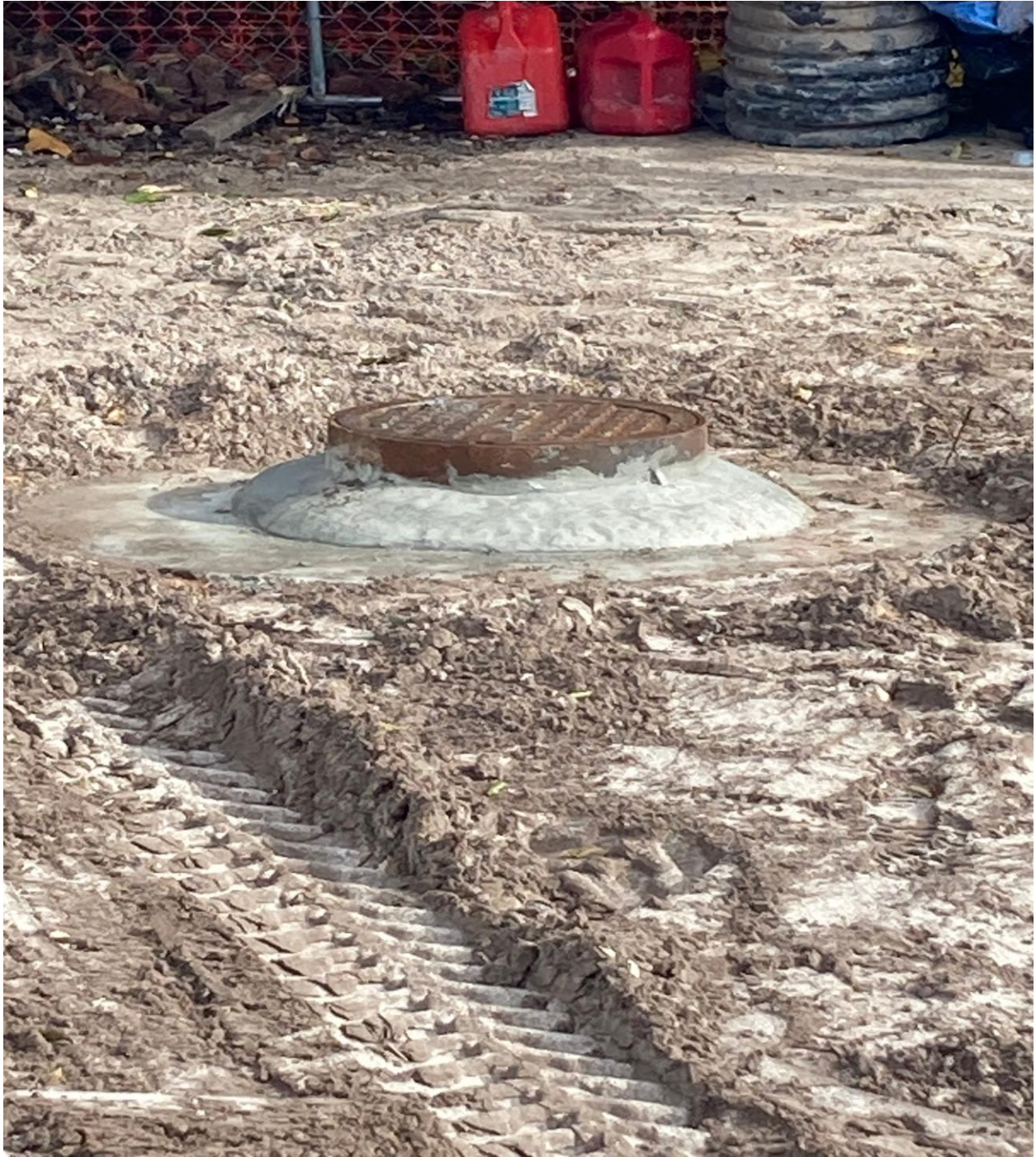
100 CENTURY BOULEVARD- NEW MANHOLE BOX INSTALLED AT THE CV MEDICAL BUILDING.
