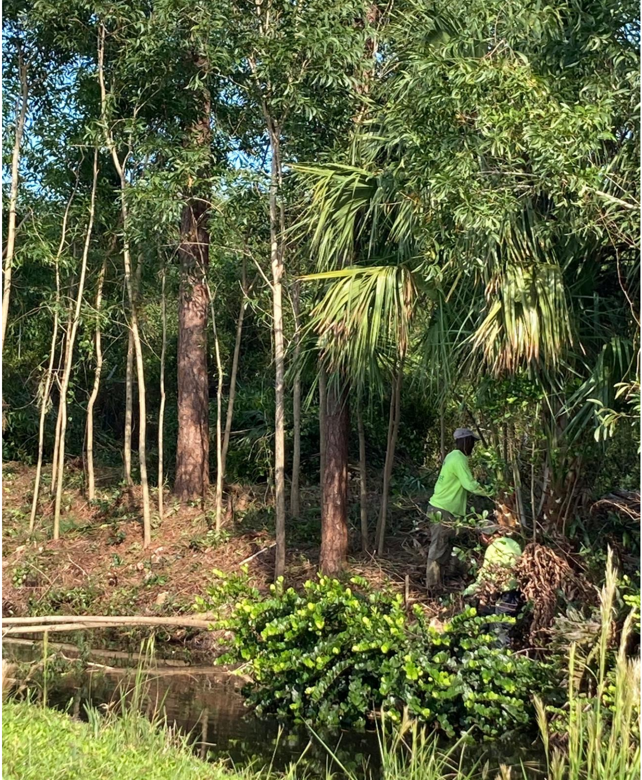
SOUTH CANAL, CANTERBURY SECTION- JUNGLE CLEARANCE CONTINUES.
