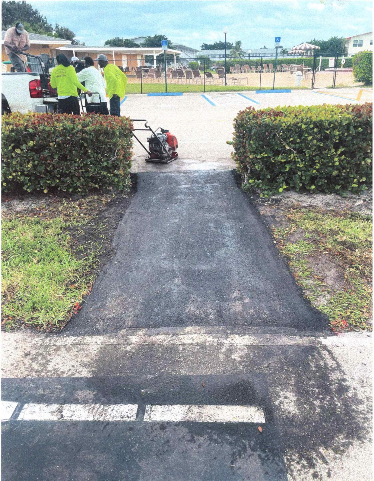
WEST DRIVE- WALKWAY REPAIR COMPLETE.
