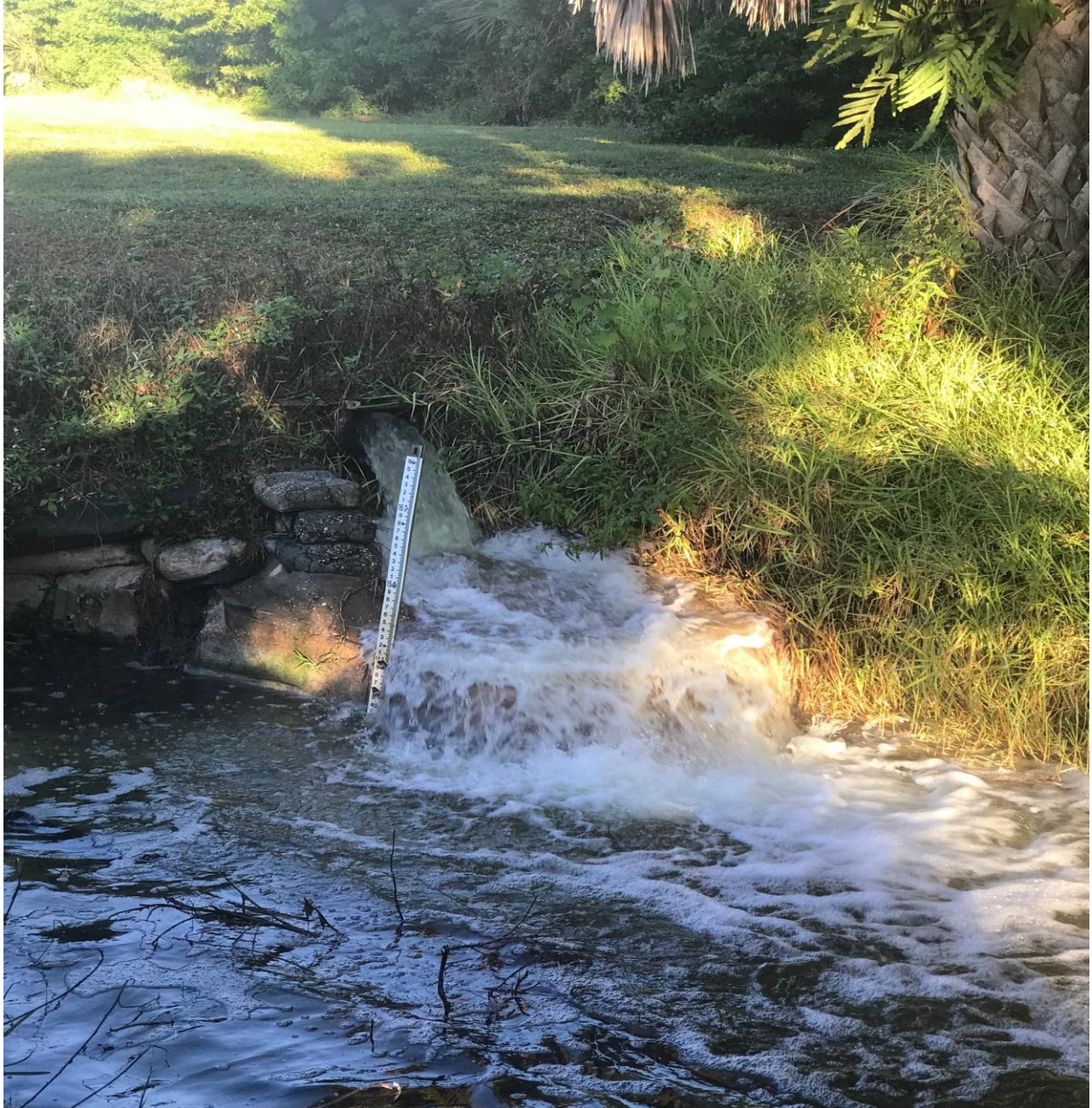
RECLAIMED IRRIGATION WATER ENTERING NORTH CANAL. THIS WATER HELPS KEEP OUR WATERWAY LEVELS UP DURING DRY MONTHS.
