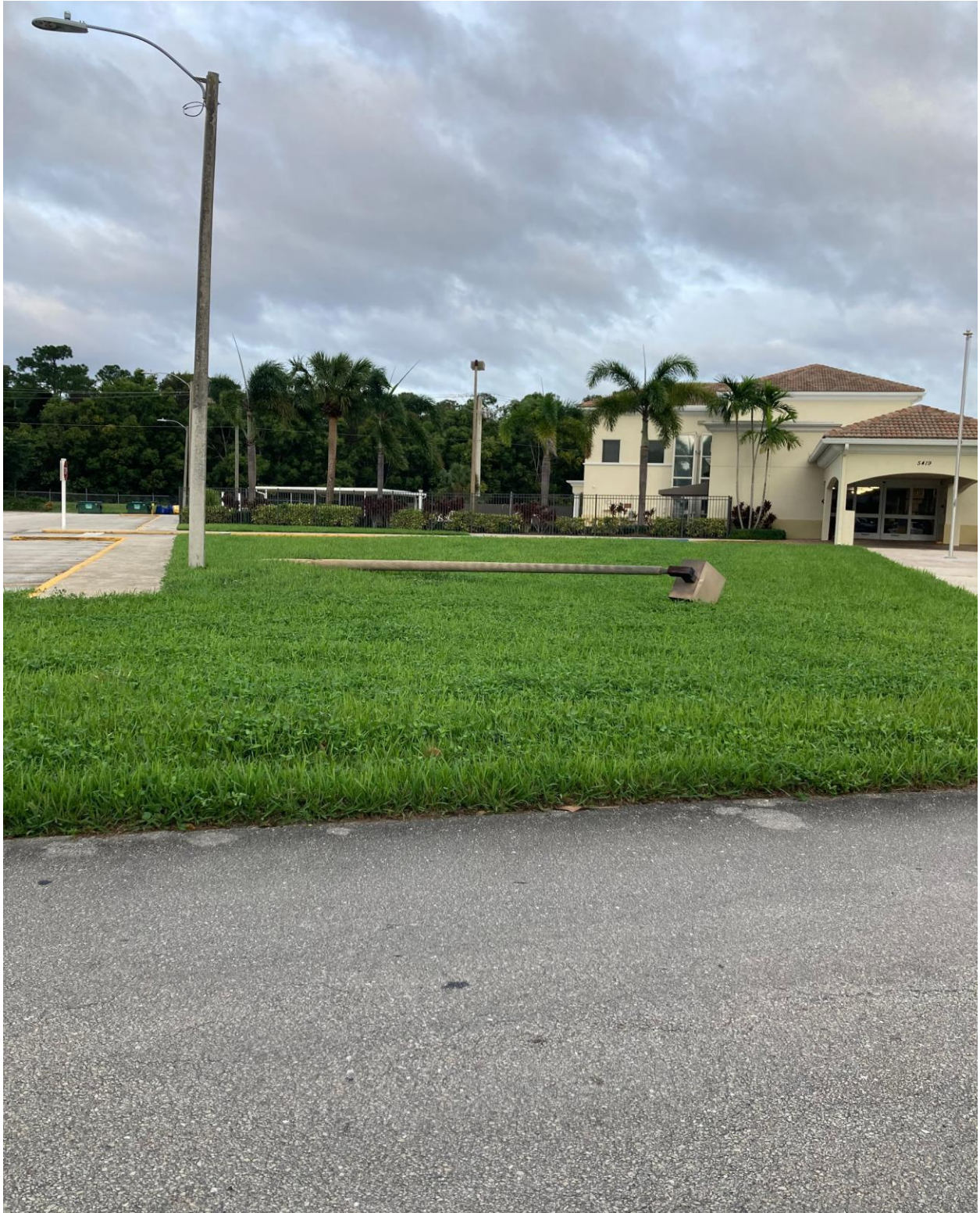
HASTINGS FITNESS CENTER- BLOWN DOWN STREETLIGHT, REPORTED TO WPRF ON 10/10.
