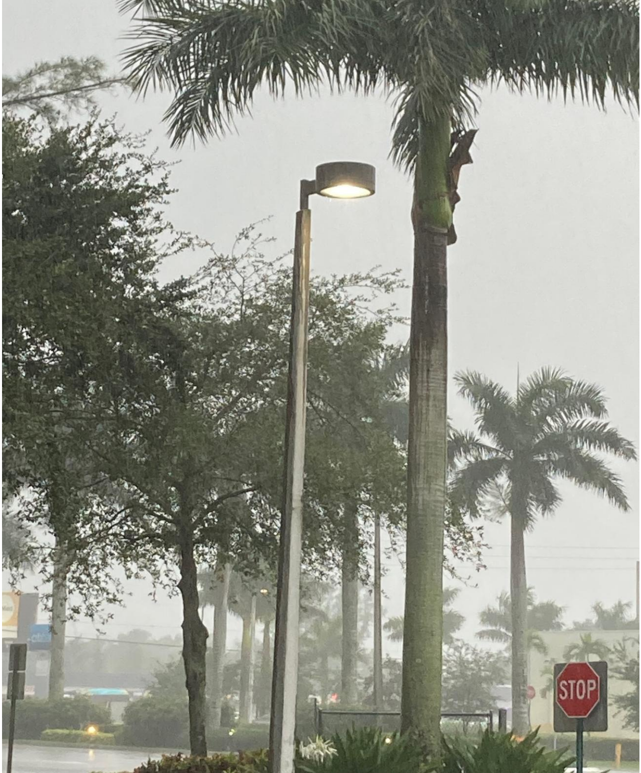
2102 WEST DRIVE- ALL PARKING LOT STREETLIGHTS ARE NOW FUNCTIONAL.
