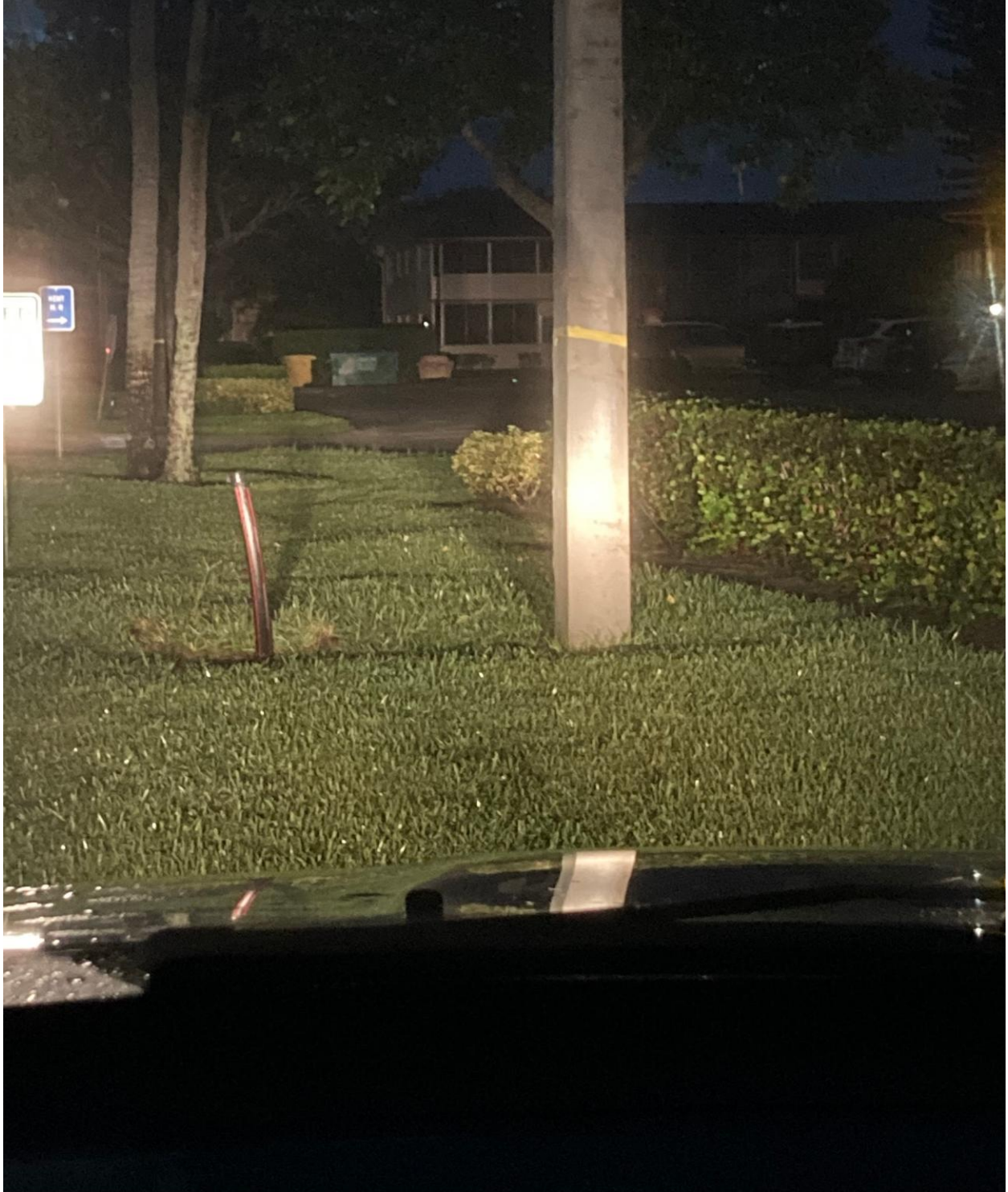
NORTH DRIVE- FPL INSTALLED A NEW UNDERGROUND POWER LINE FOR STREETLIGHTS NEAR KENT M.
