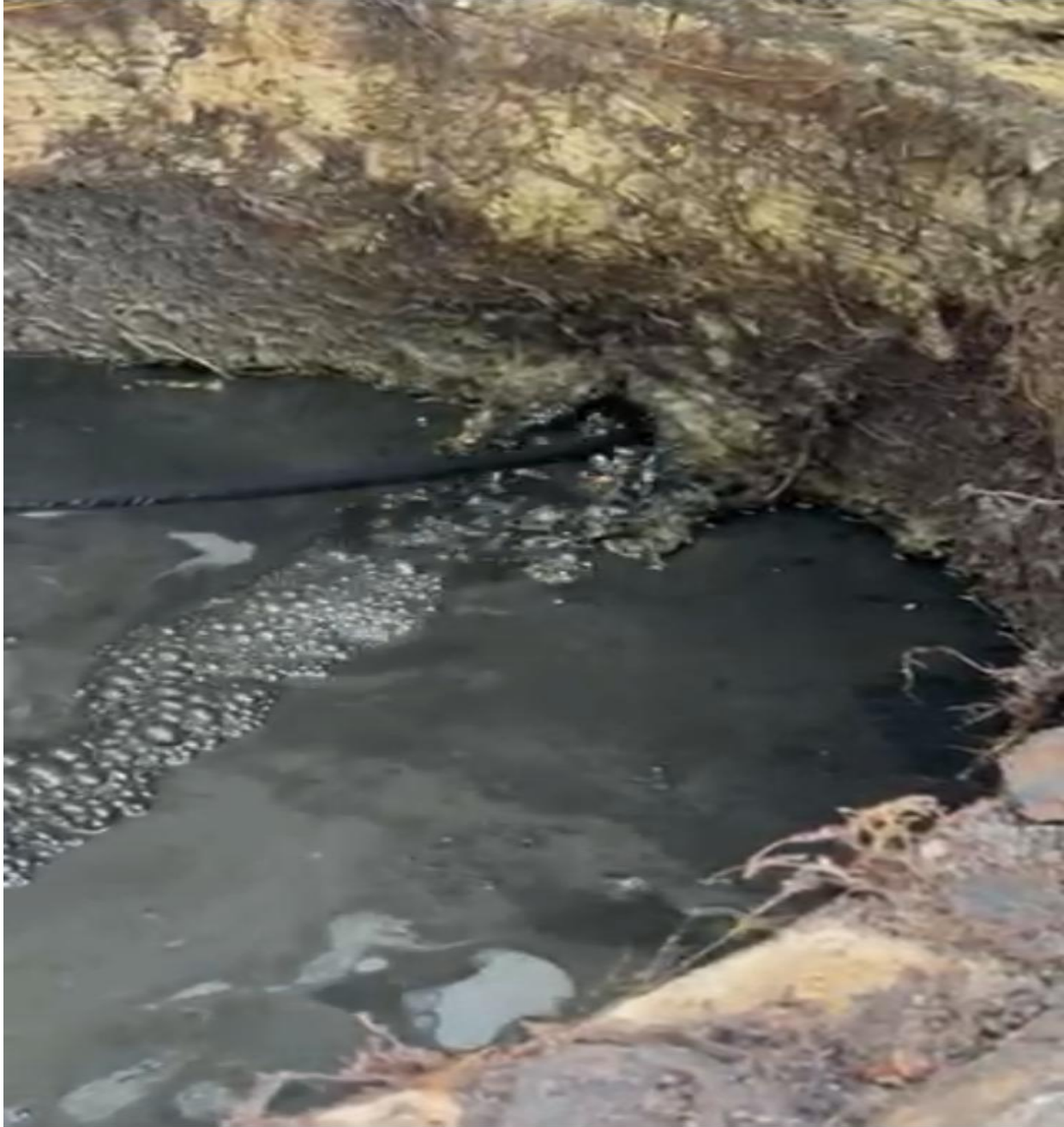
PLYMOUTH LAUNDRY- ON 9/13, THE GREYWATER DRAIN LINES AND LINT TRAP WERE CLEANED OUT BY TOP OF THE LINE PLUMBING. A NASTY, ONCE PER YEAR JOB.
