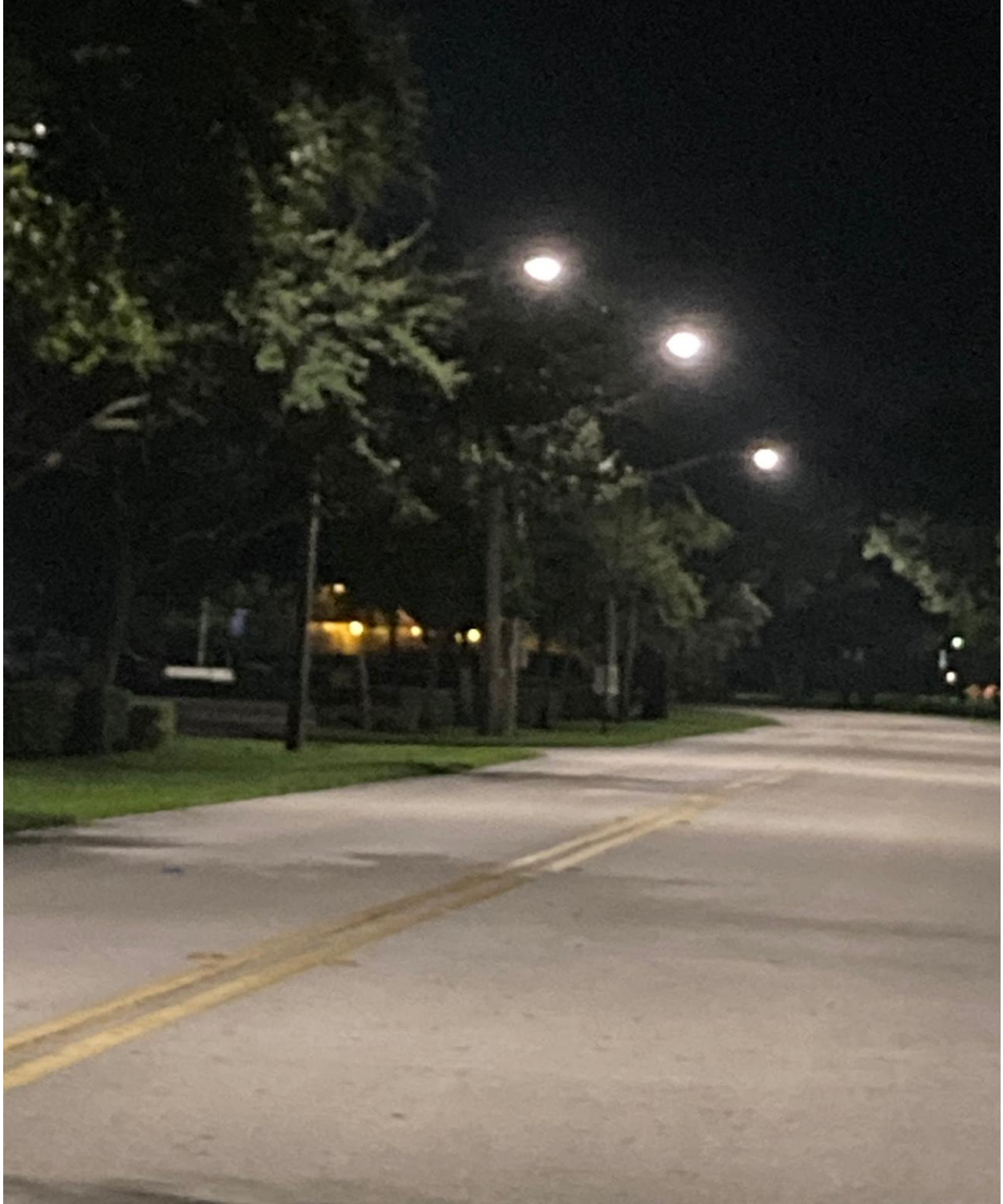
NORTH DRIVE- THE STREETLIGHTS AT THIS SECTION ARE BACK ON.
