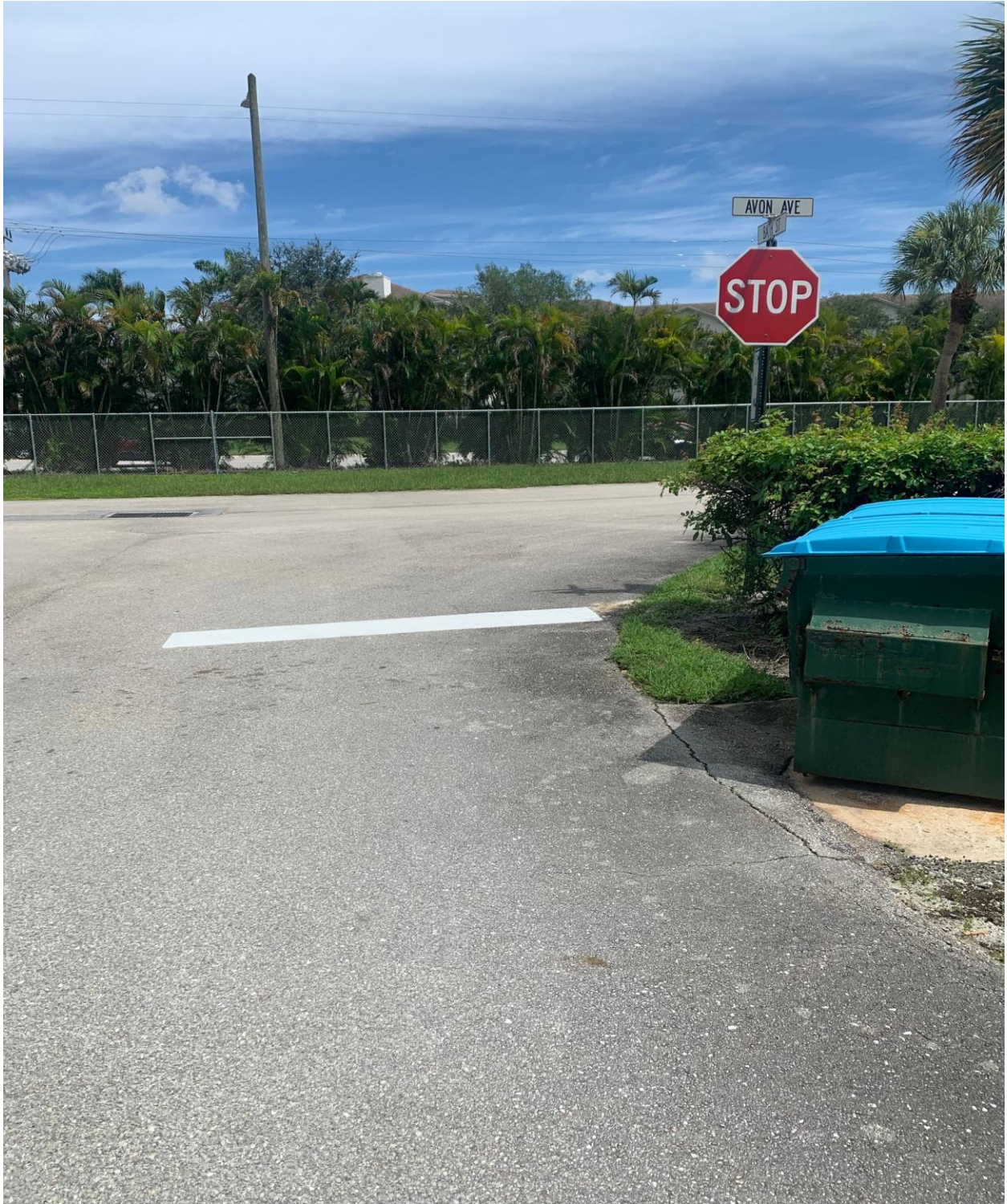
EASTHAMPTON SECTION- NEW STOP SIGN AND STOP BAR. NICE JOB, JOSE.
