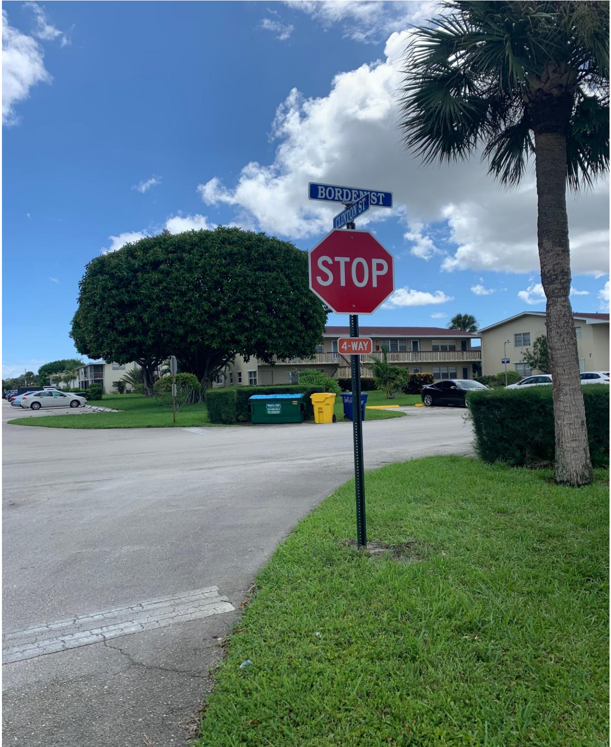
WALTHAM SECTION- NEW, MANUAL COMPLIANT STOP SIGN INSTALLED BY HANDYMAN JOSE. FADED STOP BAR WILL BE PAINTED AS WELL.
