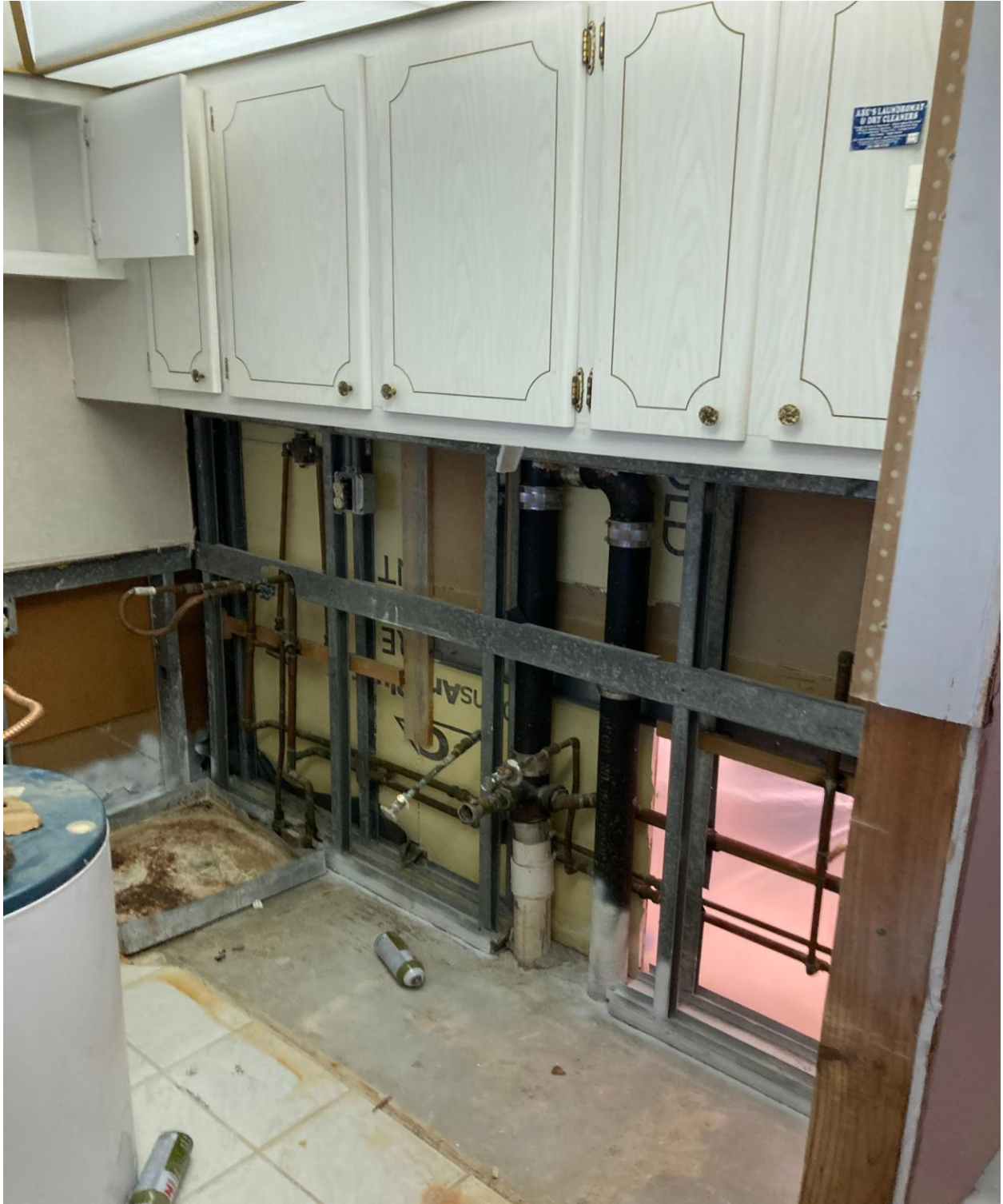
180 COVENTRY H- GUT WORK ON THIS UPPER UNIT IS NEARLY COMPLETE.
